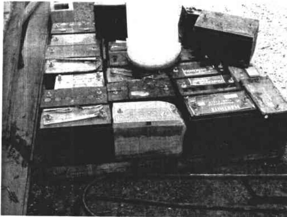
Photo no. 4: Lead acid batteries on a pallet next to trailer no. 2.
