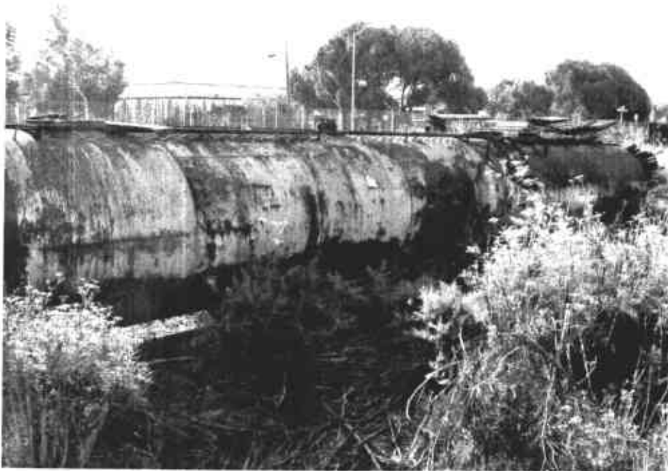
Photo no. 14: Tank T-1 on the south side of the property.
