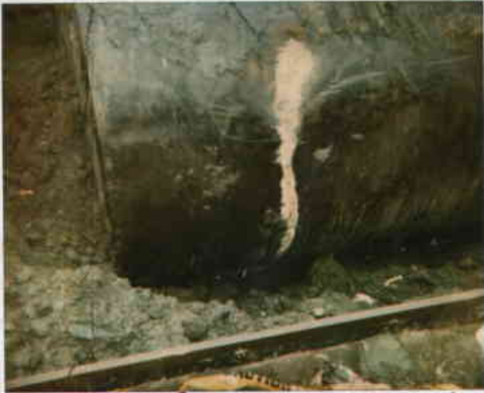
PLUMBER'S PUTTY FILLING CRACK 4-23-99
