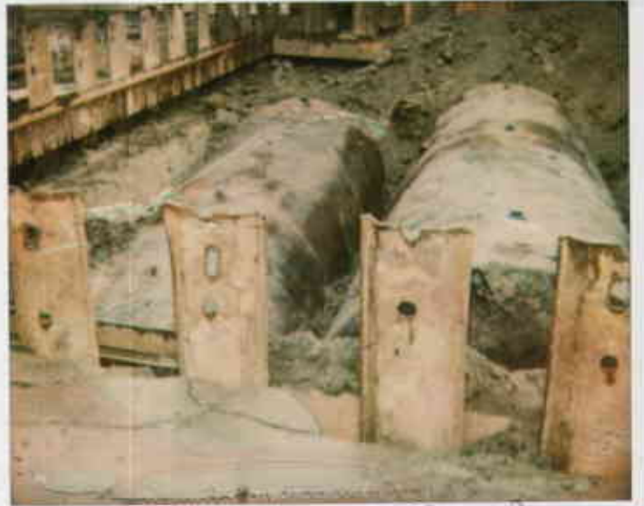
SCHOOL ST (END) OF TANK PIT 4-23-98
