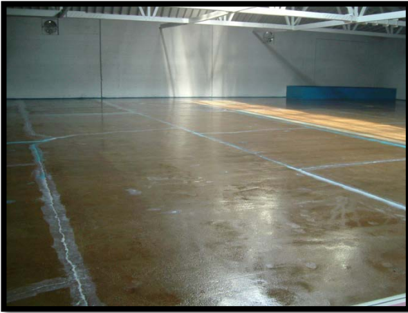
Completed surface preparation consisting of shot blasting, Retro-Coat PREP to fill joints and cracks and a 6 mil application of Retro-Coat PRIMER
