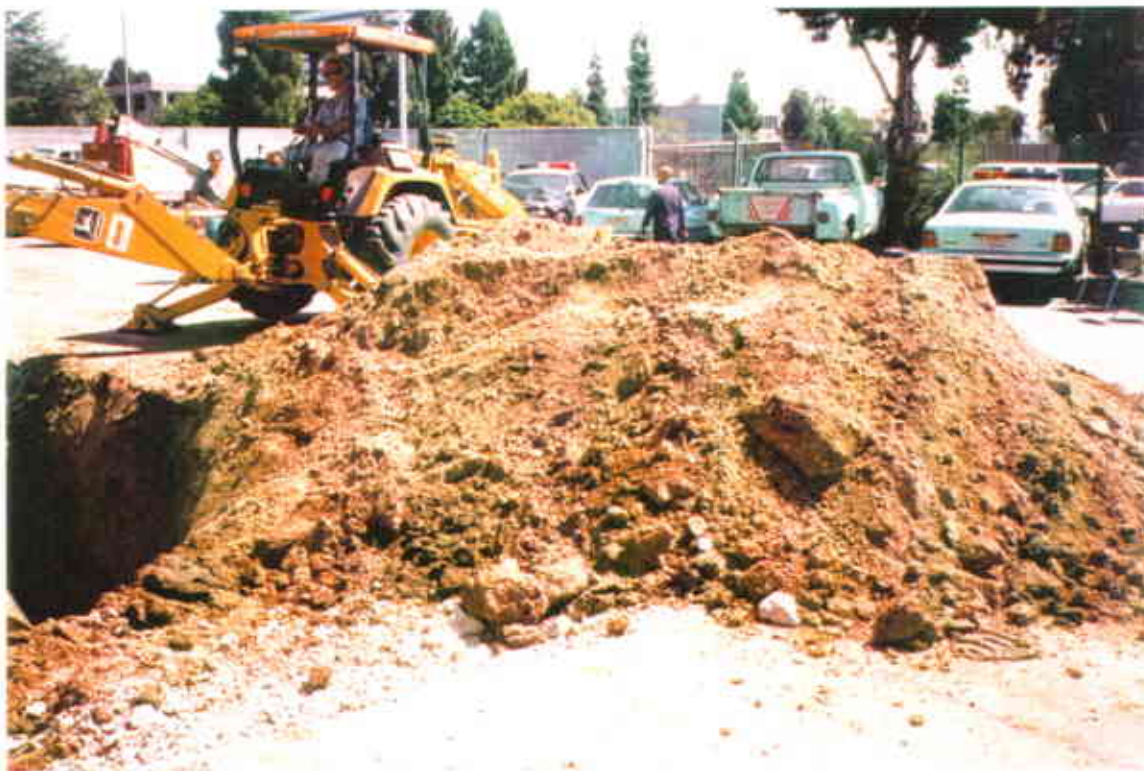
b. The vent/fuel lines are being prepared for removal.
