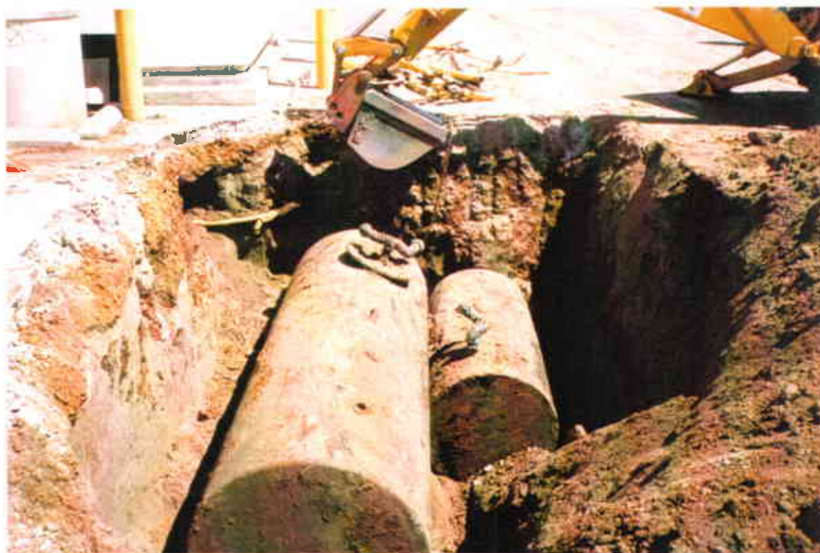
e. The removal of the USTs commenced.
