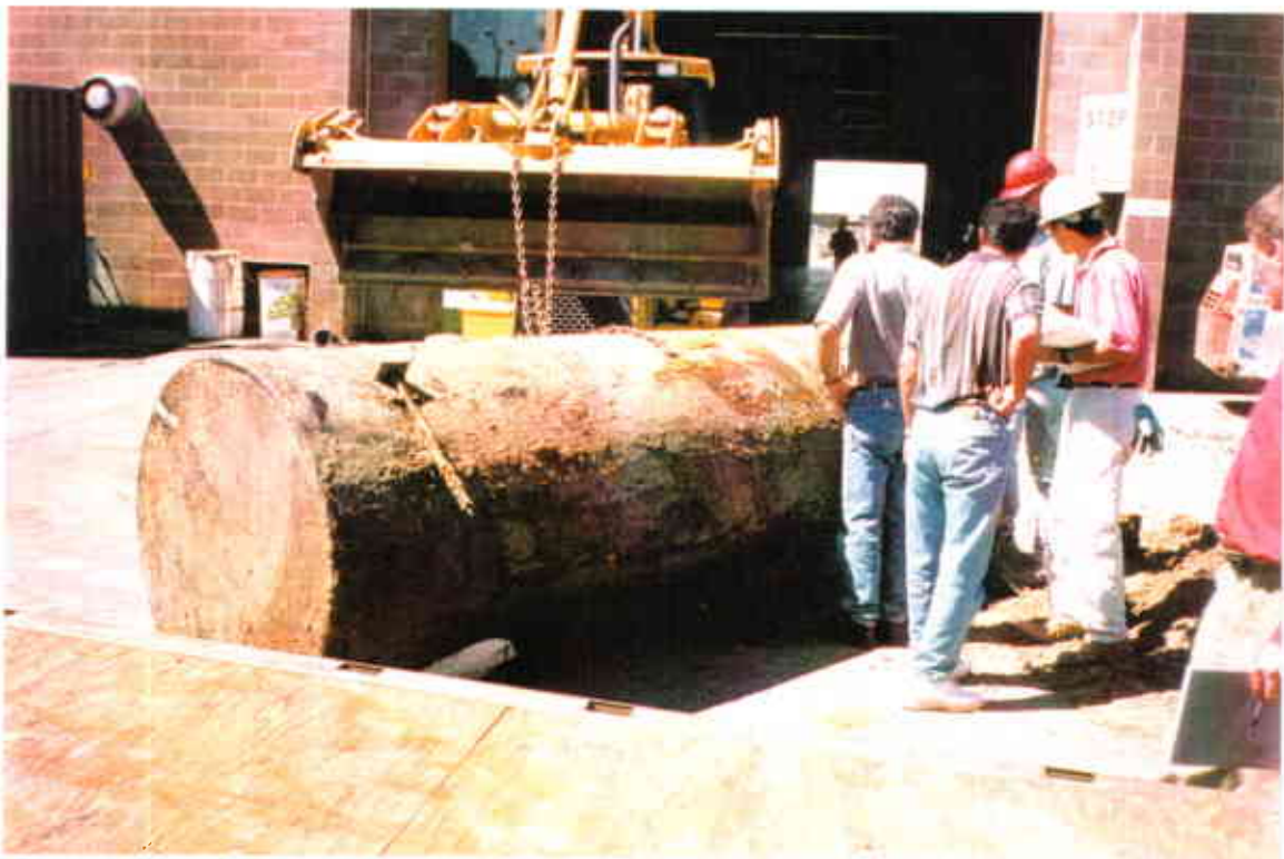
h. UST#10 is staged for inspection by City and County Officials.
