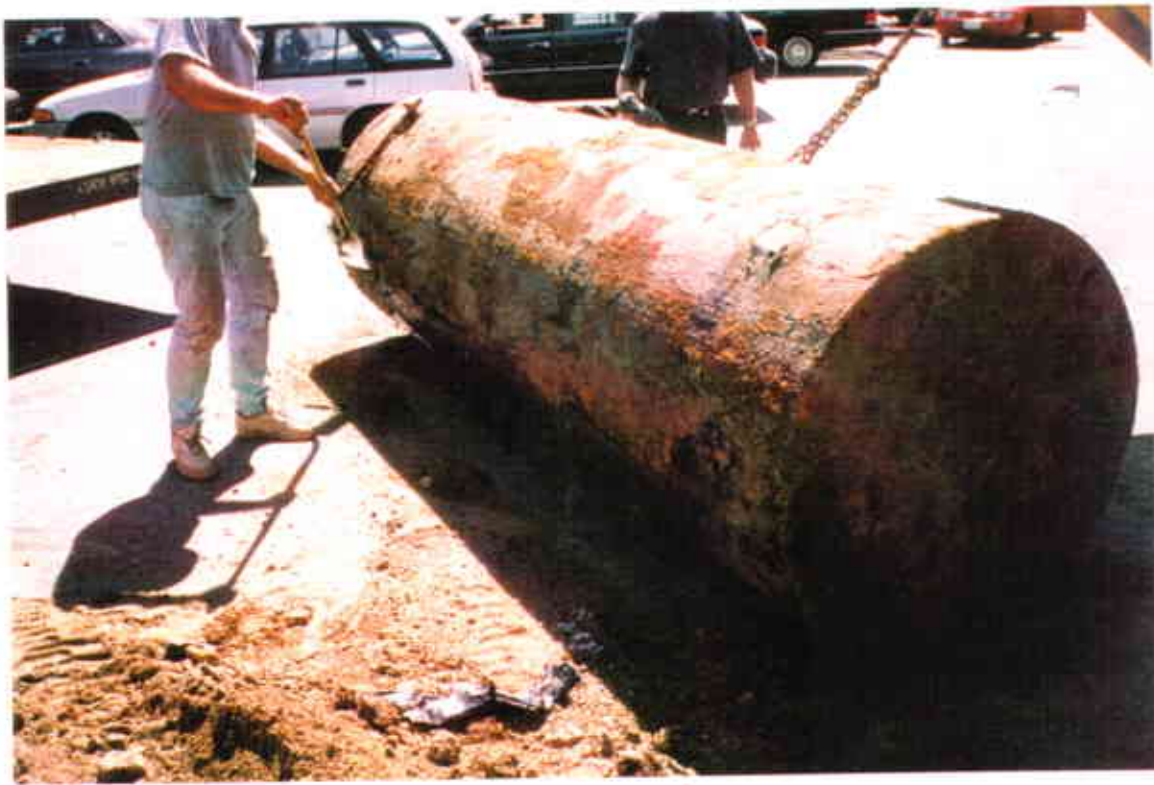
i. UST #10 is staged for transportation and disposal.
