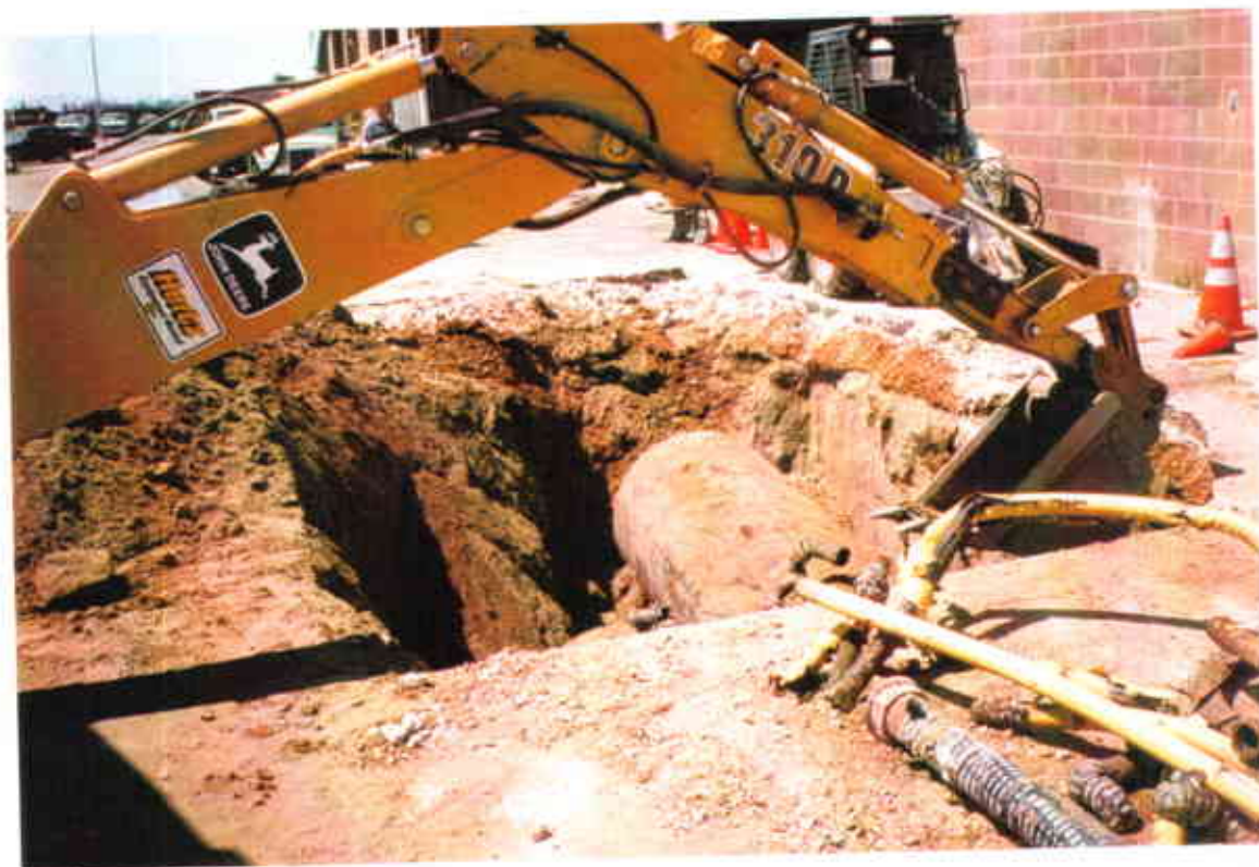
c. Vent/fuel lines removal commenced.
