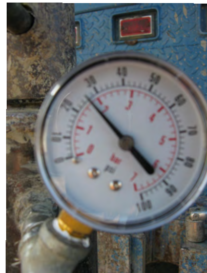
Pressure Grout at 26 PSI for 5 minutes at MW-4
