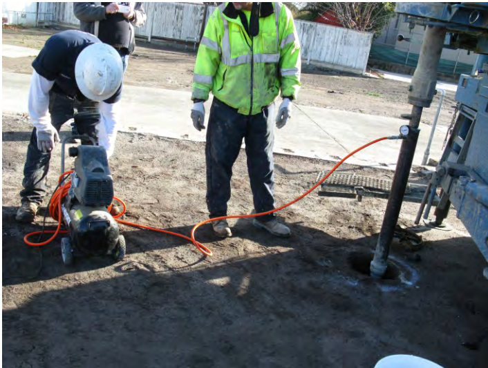
Pressure Grout with Threaded Coupling at MW-4
