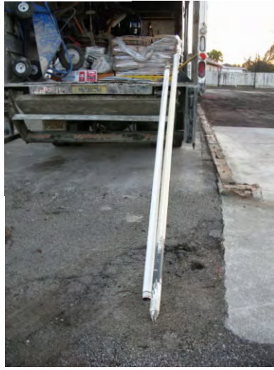
Casing Pulled at MW-3
