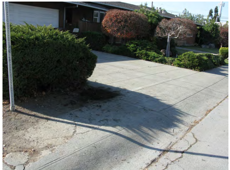
Completed Well Abandonment at MW-5
