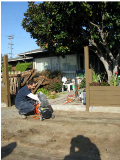
Pressure Grout at MW-6
