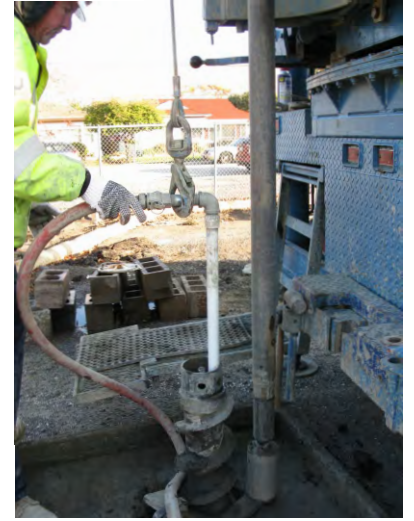
Tremmie Grout at MW-3
