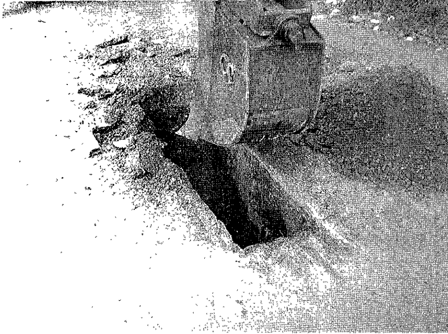
Photo 1: Excavator rig trenching in area of SP-4.
