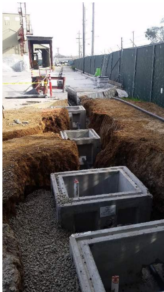
Figure 3: Well Vault Placement
