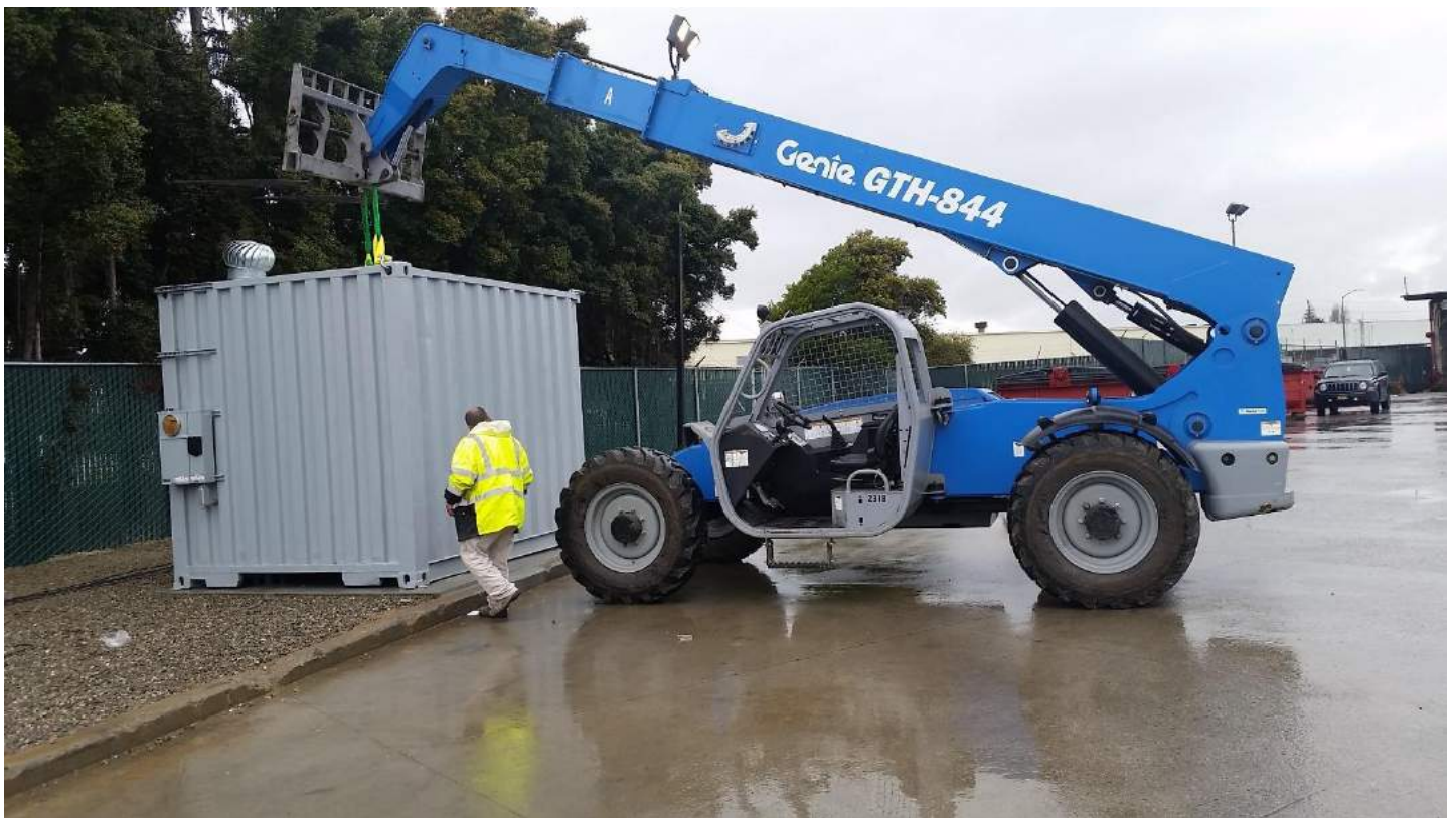
Figure 13: Placing Cargo Shed Onto Concrete Slab Foundation
