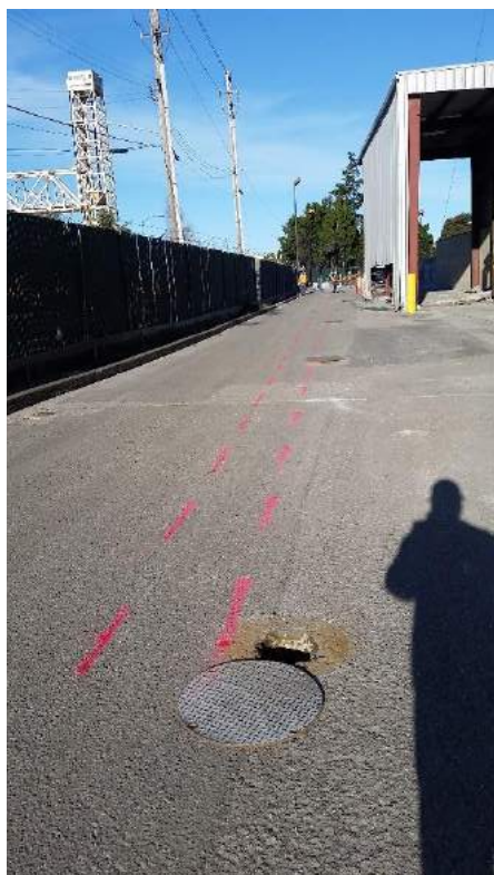
Figure 1: Concrete and Asphalt Area Marked for Sawcutting
