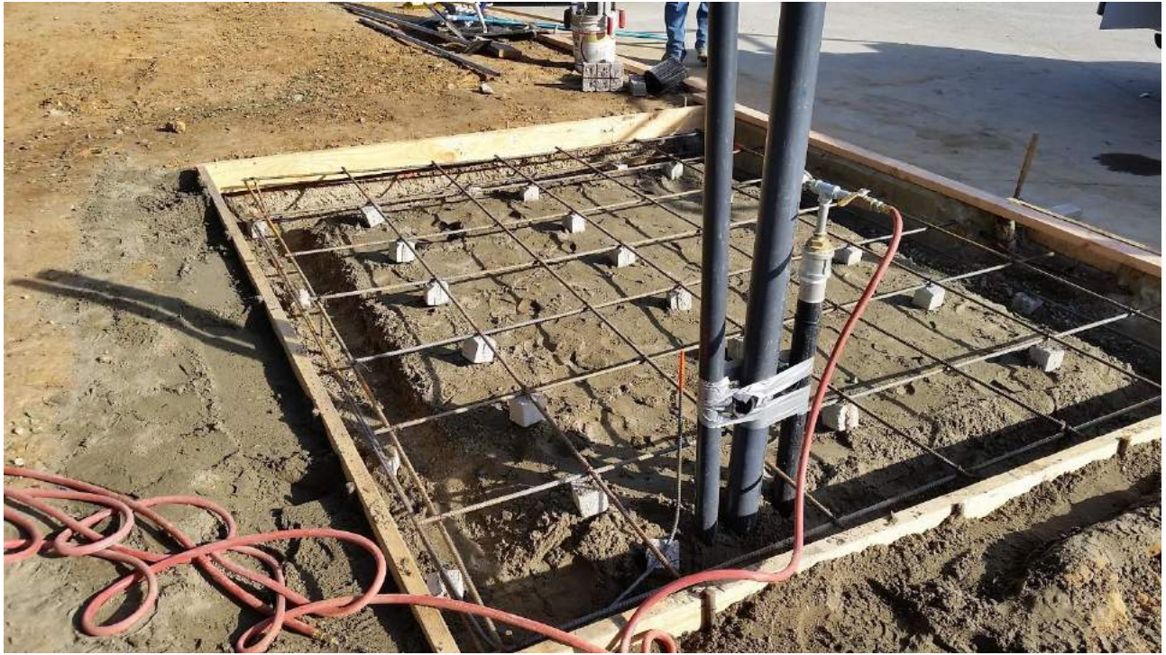
Figure 11: Cargo Shed Foundation with Ufer Prior to Pouring Concrete Slab
