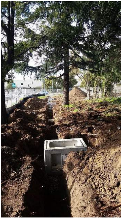
Figures 7 and 8: Placing Well Vaults in Landscaped Area
