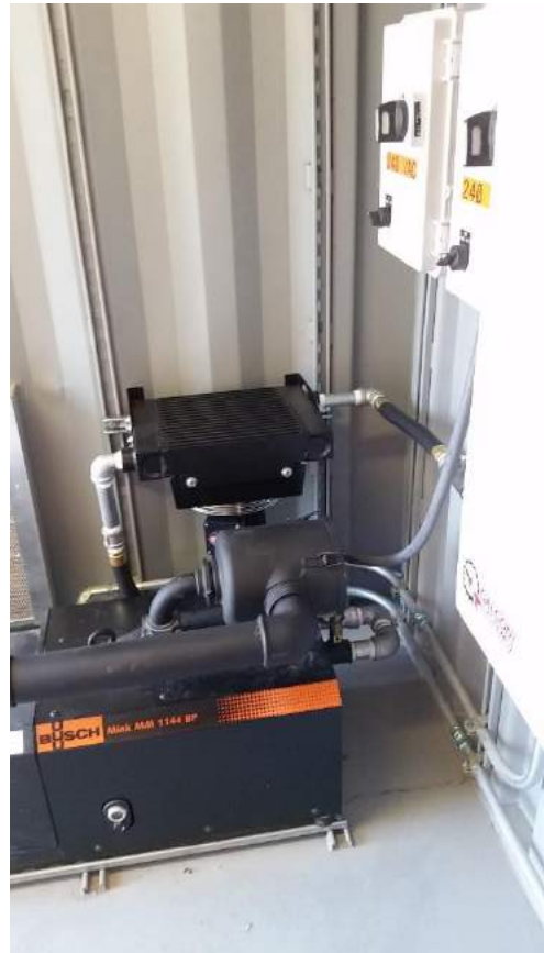
Figure 19 and 20: Heat Exchanger Mounting Position and Connections
