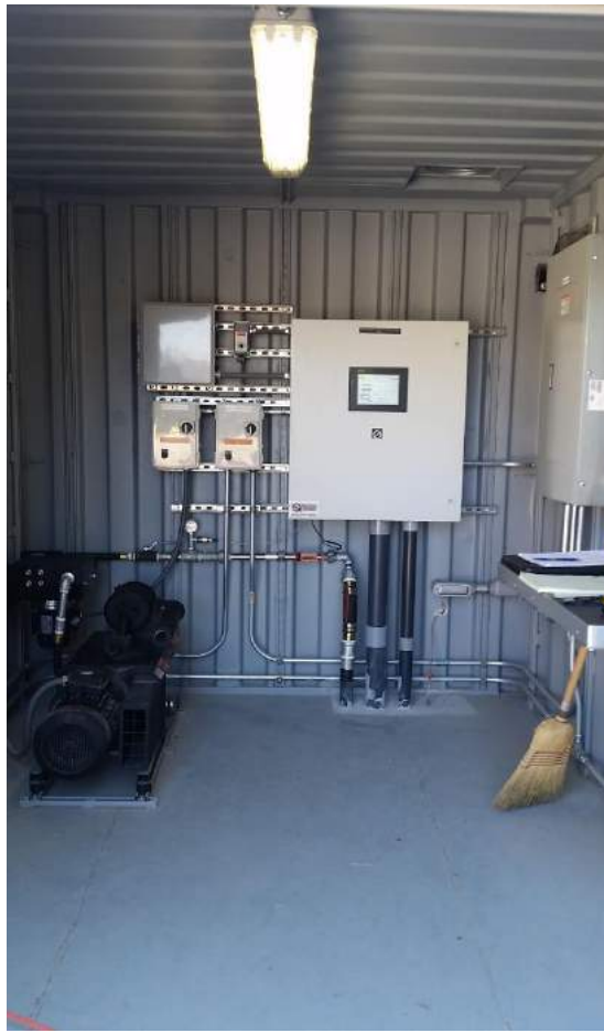
Figure 18: Completed Heat Exchanger Installation
