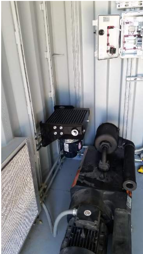
Figure 19 and 20: Heat Exchanger Mounting Position and Connections
