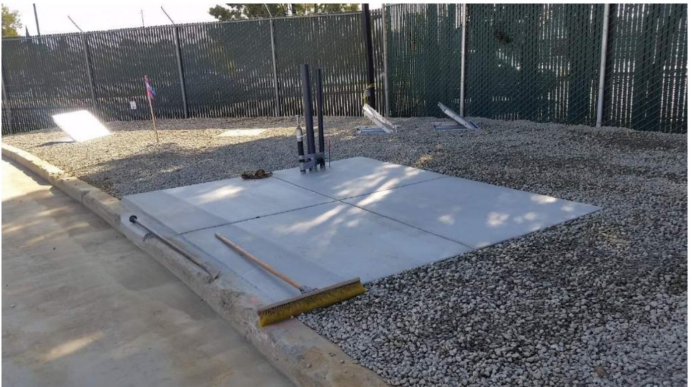
Figure 12: Completed Cargo Shed Foundation
