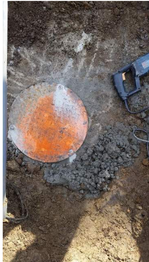
Figure 6: Bolt-Down Steel Plate for Added Protection
