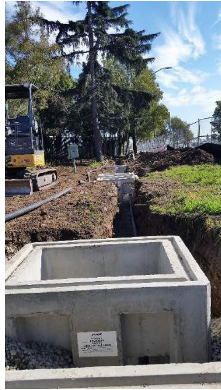
Figures 7 and 8: Placing Well Vaults in Landscaped Area
