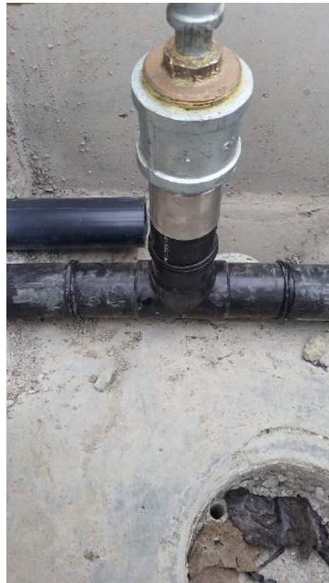
Figure 10: Welded PE Tee with PE to Galvanized Transition Fitting
