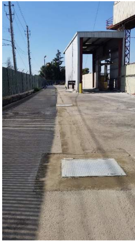
Figure 15: Backfill and Surface Restoration Completed Inside Property
