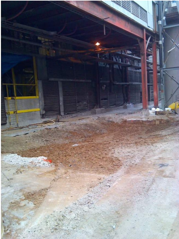
Figure 15: Backfill Compaction Completed @ Ex C
