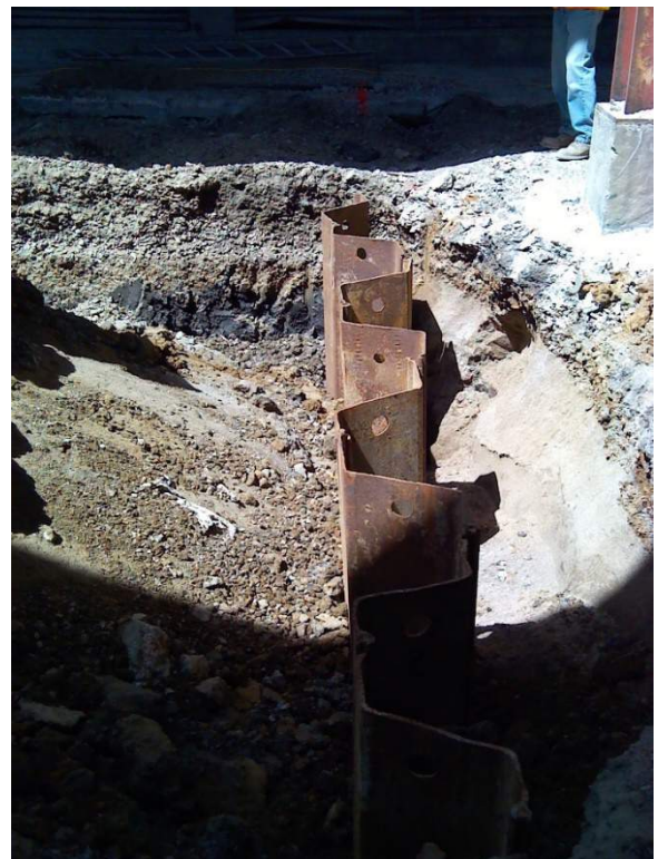
Figure 11: Shoring @ Ex C
