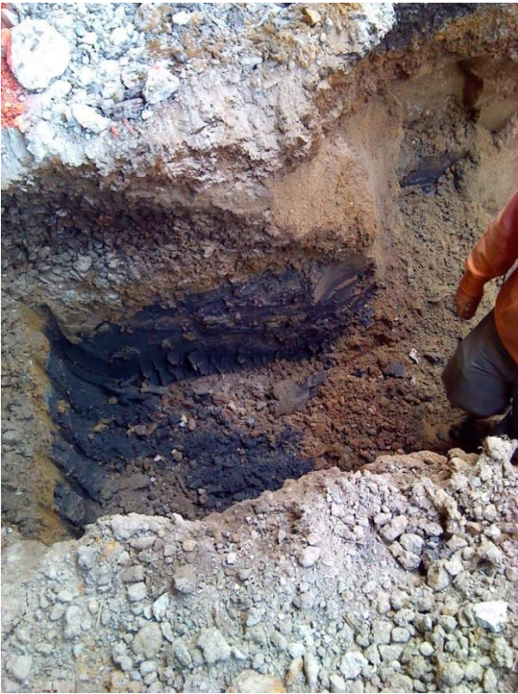
Figure 8: Beginning Excavation @ Ex C
