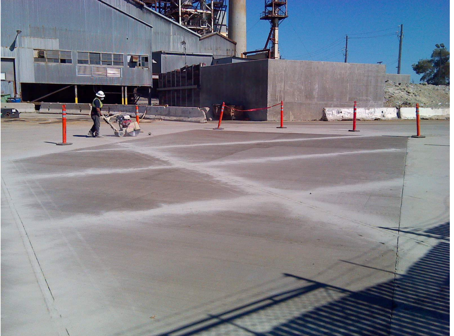
Figure 47: Finishing Touches @ Ex E
