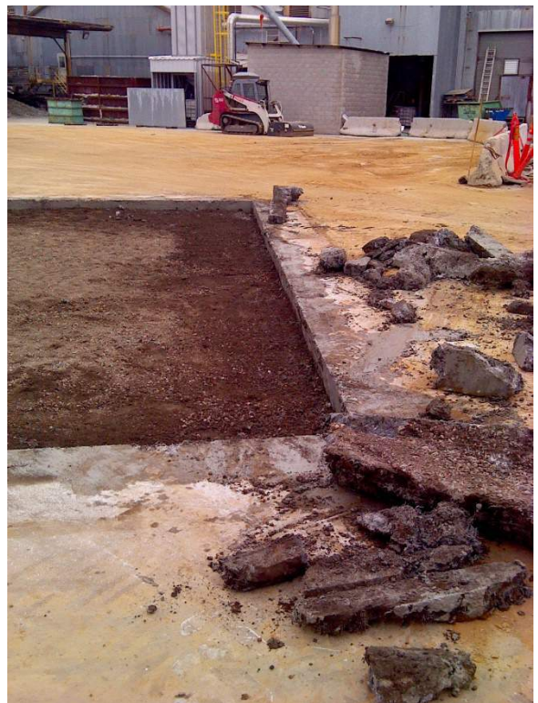
Figure 44: Saw-cut @ Ex E
