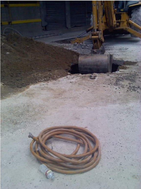
Figure 4: Backfilling Pothole
