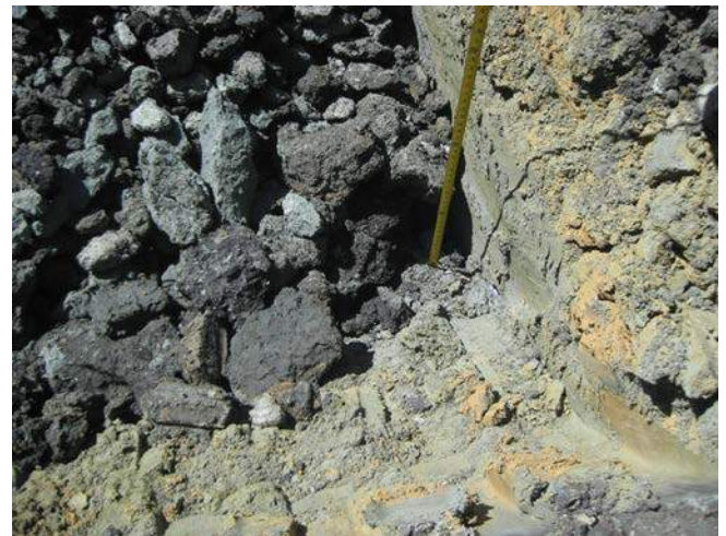
Figure 8 Soil in Excavation B at a depth of 20 feet below grade. No groundwater is visible, but staining is strongly evident.
