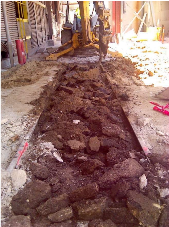
Figure 6: Removing RR Tracks
