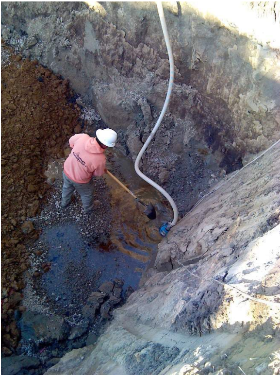
Figure 29: Dewatering Ex E
