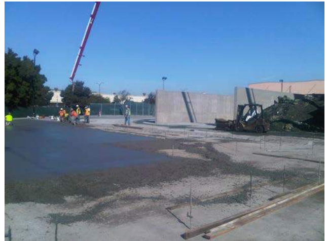
Figure 10 Paving in the Western UST Area, with new cullet bunkers on the right.
