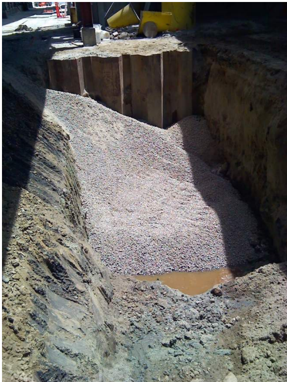
Figure 13: Ramp into Ex C
