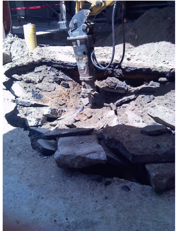
Figure 5: Removing Asphalt Surface
