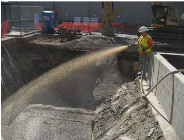
Figure 3 Placing ORC slurry into Excavation D
