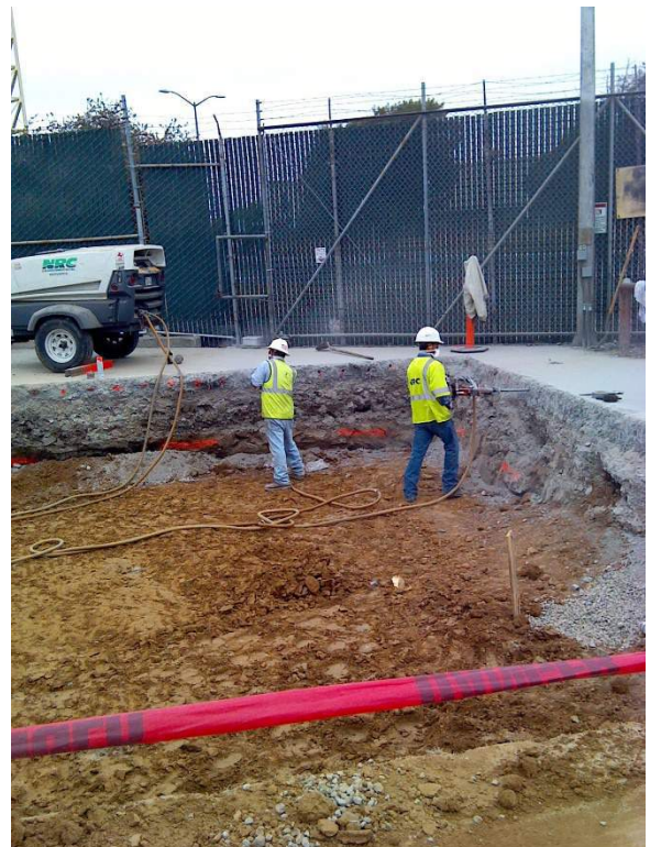
Figure 36: Drilling Dowel Holes @ Ex E
