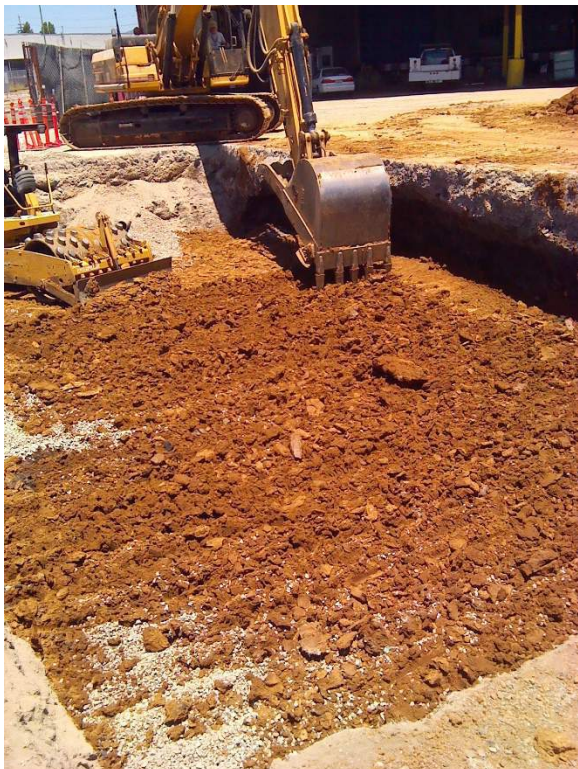
Figure 35: Scraping Backfill Lift @ Ex E
