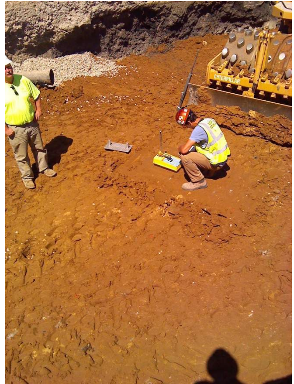
Figure 34: Compaction Test @ Ex E
