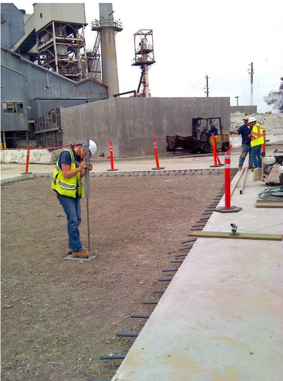
Figure 43: Trench Backfill Compaction Test @ Ex E
