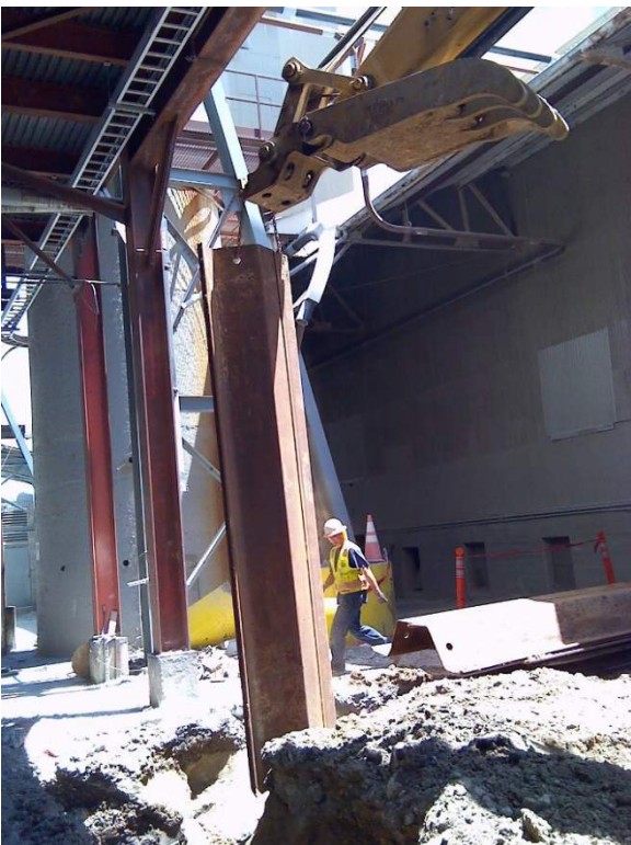
Figure 10: Placing Shoring @ Ex C
