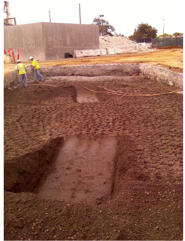
Figure 38: Aggregate Base Compaction Test Locations @ Ex E
