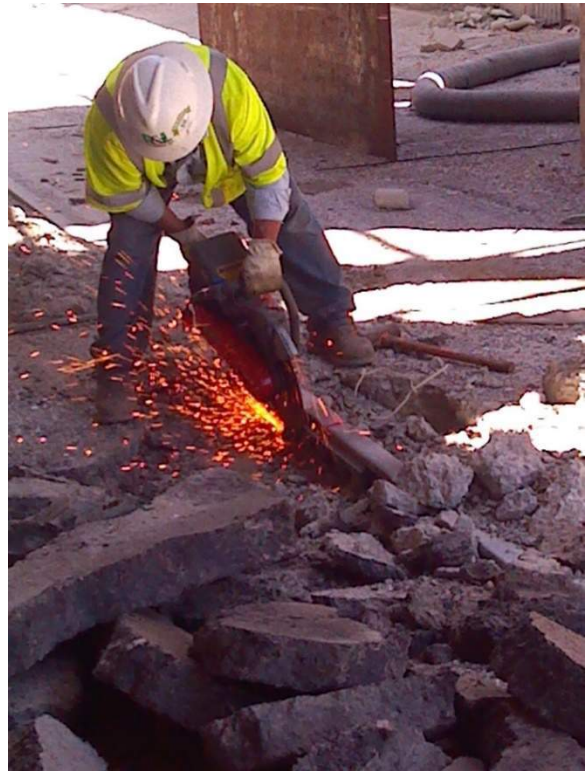
Figure 7: Saw-cutting RR Bolts
