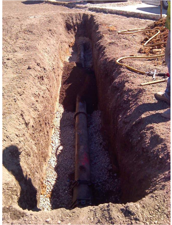
Figure 42: Replaced Water Pipe @ Ex E
