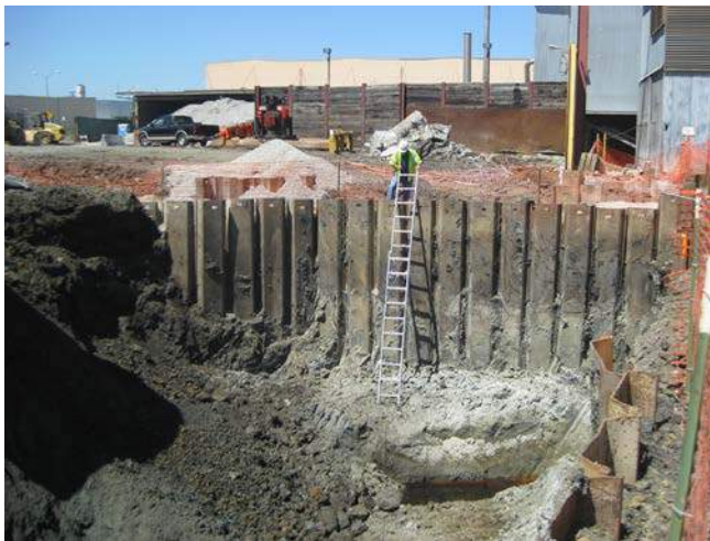
Figure 7 The north side of Excavation B.
