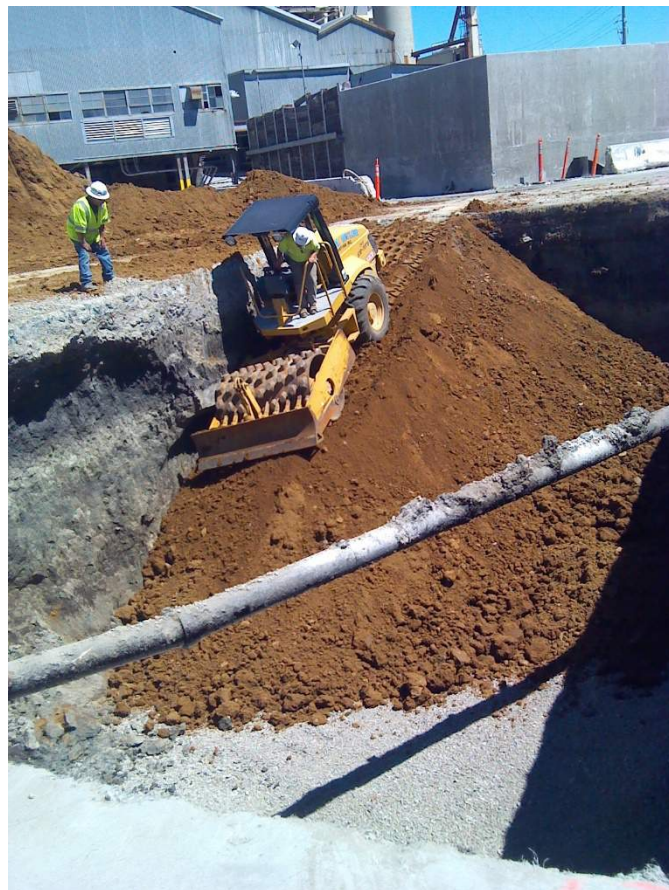
Figure 28: Backfill Ramp Into Ex E
