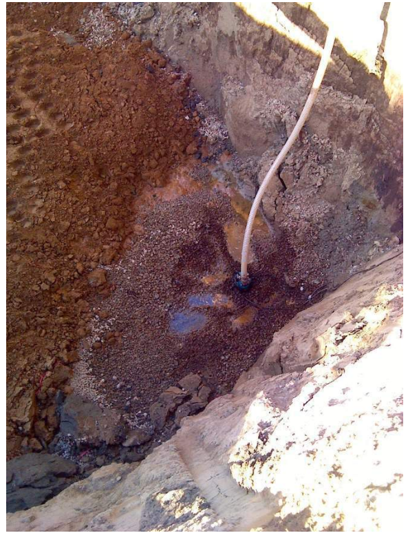
Figure 30: Dewatering Ex E
