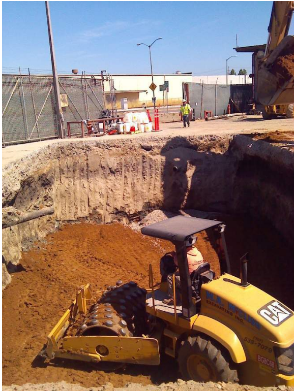
Figure 33: Compacting Backfill @ Ex E
