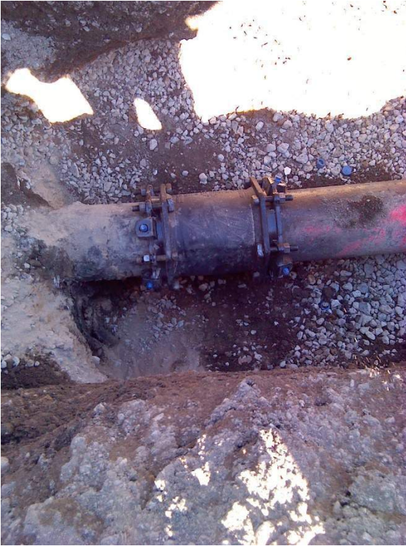
Figure 41: Sleeve Coupling for Water Pipe @ Ex E
