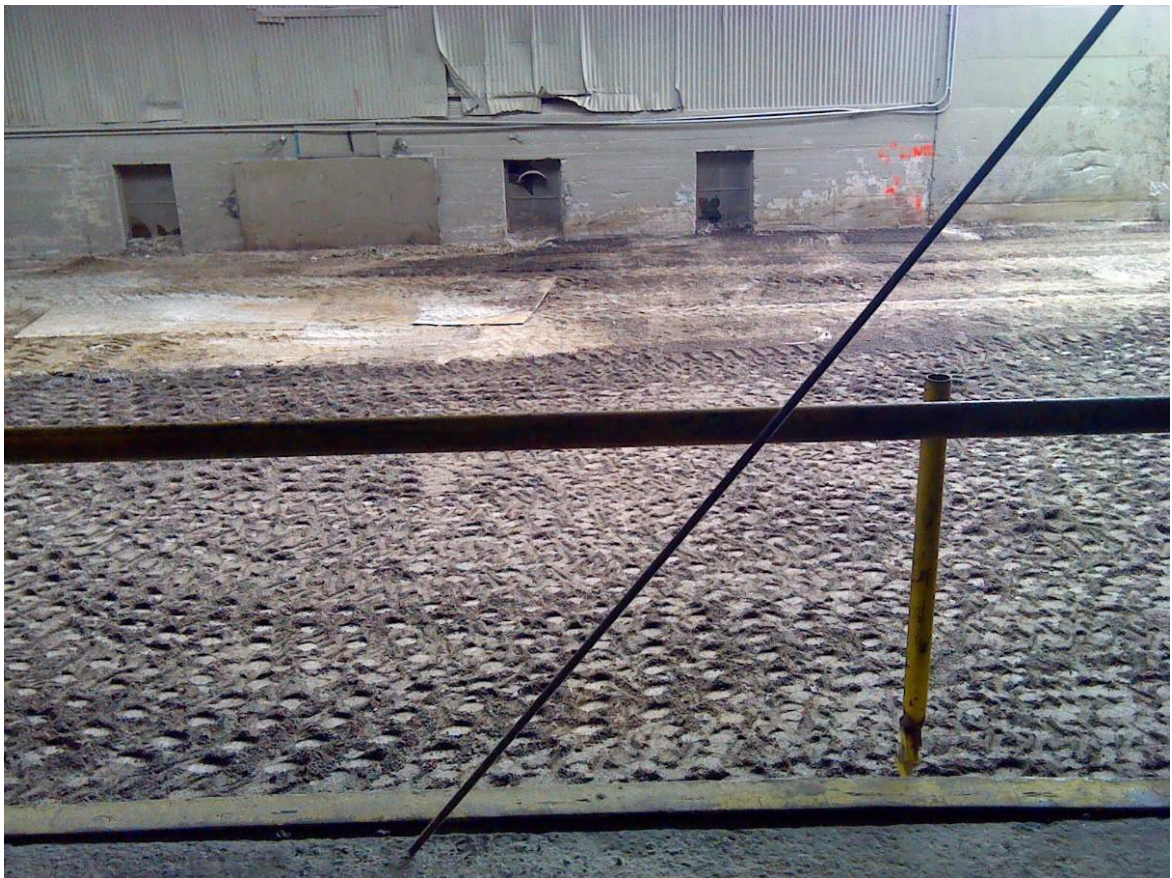
Figure 17: Aggregate Base Compacted @ Ex C
