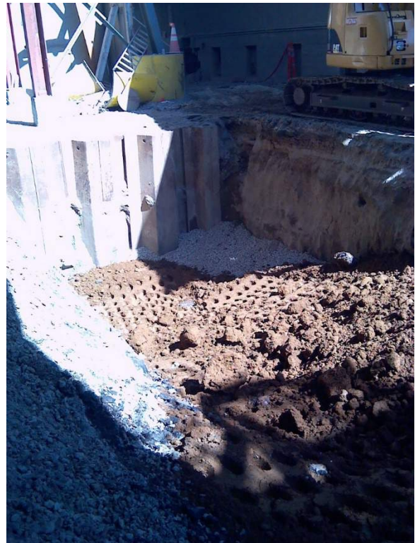
Figure 14: Compacting Backfill @ Ex C
