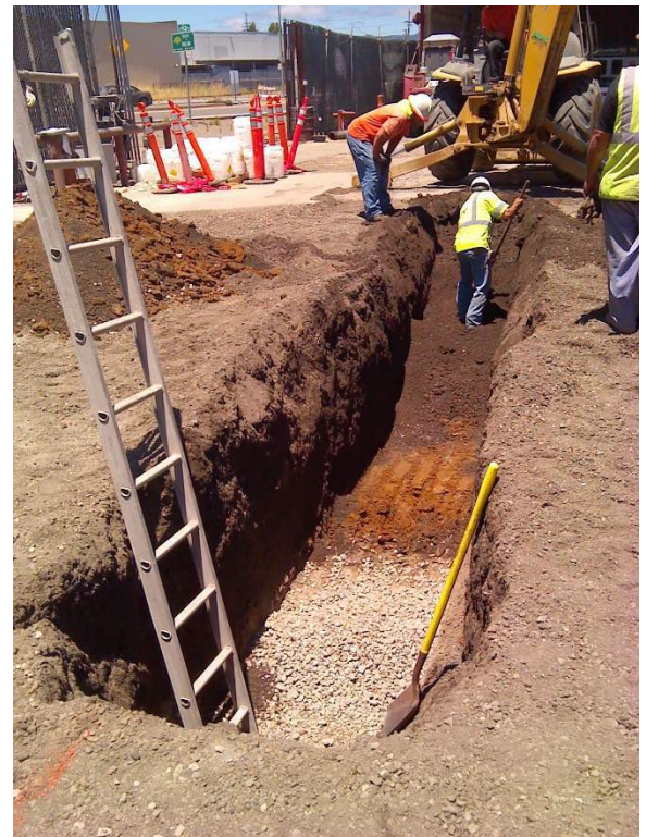
Figure 40: Water Pipe Trench @ Ex E
