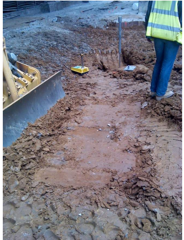
Figure 16: Compaction Tests @ Ex C
