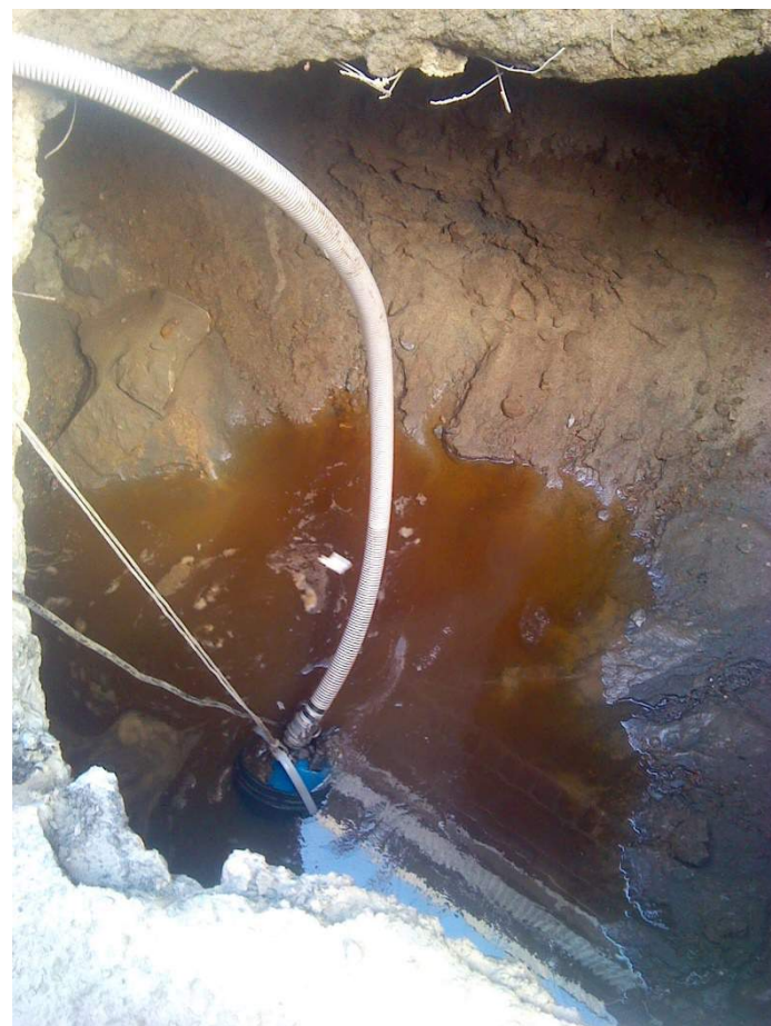
Figure 3: Ex C Dewatering Pothole
