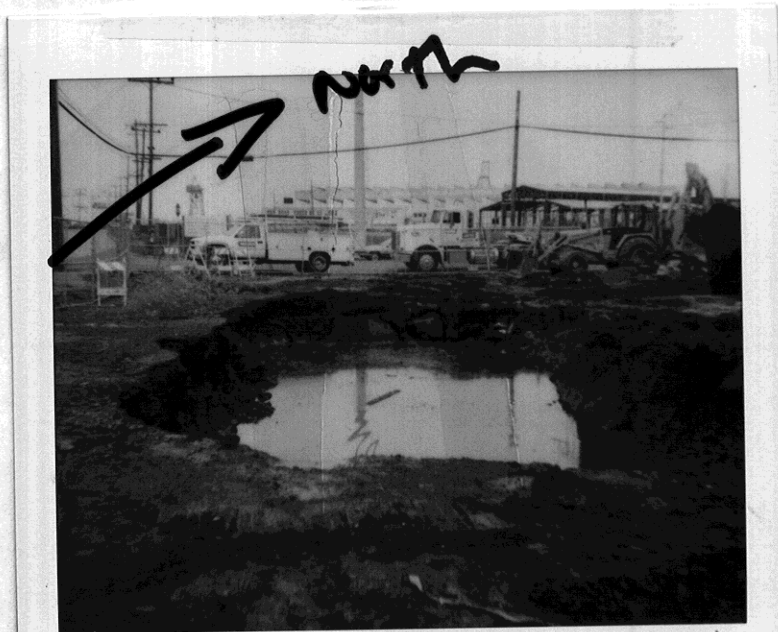
2-6k UST pit // to Main 12/6/99 St. looking North
