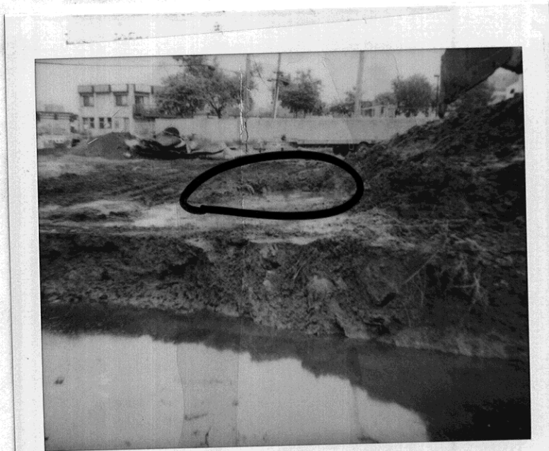
location of sump/septic tank. GW in pit . 12/6/99
