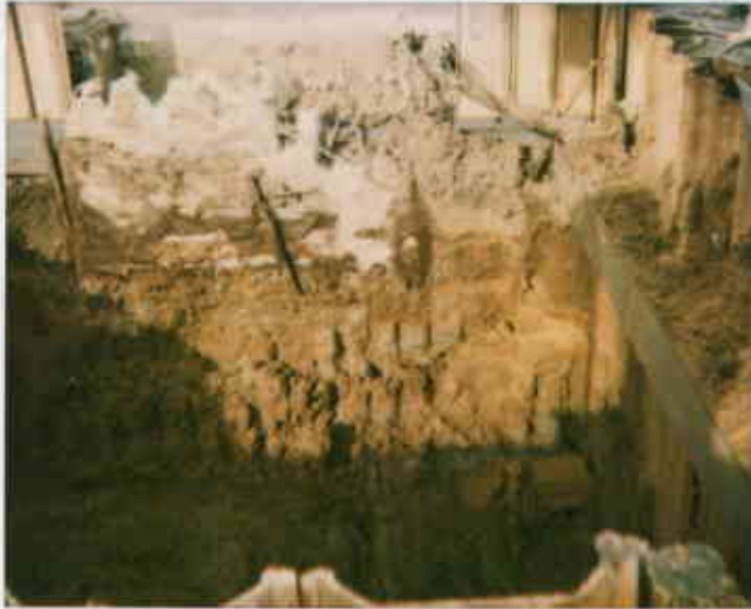
ST10 355 - Overhead excavation 12/29/93 P&E Hollis St
