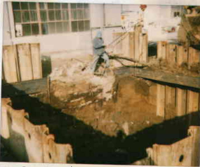
ST10 355 Overhead excavation 12/29/93 P&E Hollis St
