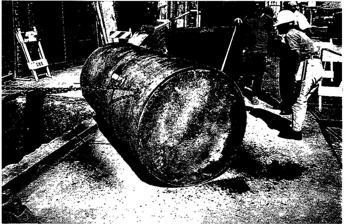
Photograph 1: Gasoline UST (facing northwest).
