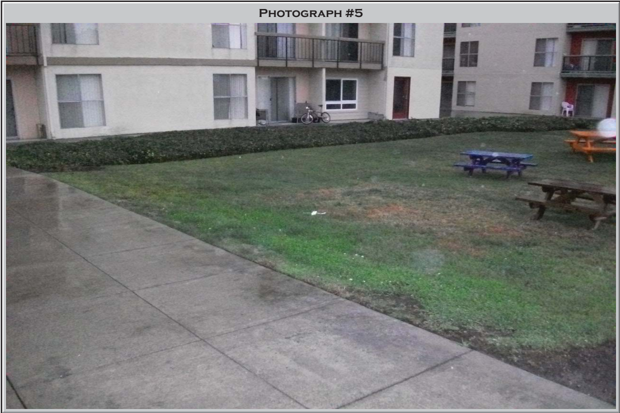
Soil boring B-5 located in the center of the subject property to the south of the leasing office structure
