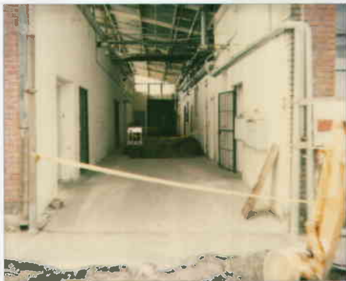
Hallway w/ at least 1 UST assumed Bunker @ 4/30/92
