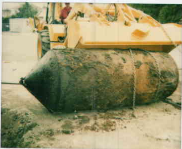
5427 Telegraph Ave. Oakland 94609 1000 waste oil tank outside bldg. 1 tip - had help 5/11/92
