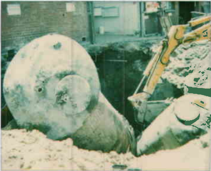
5427 Telegraph Ave. 94609 Tanks IV G & H 5/21/92
