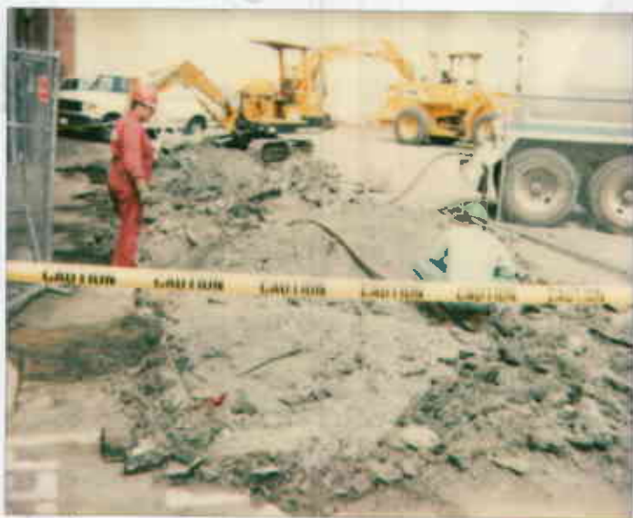
Area of n10 Stoddard Tank Tanks are covered assumed BK 4/30/92
