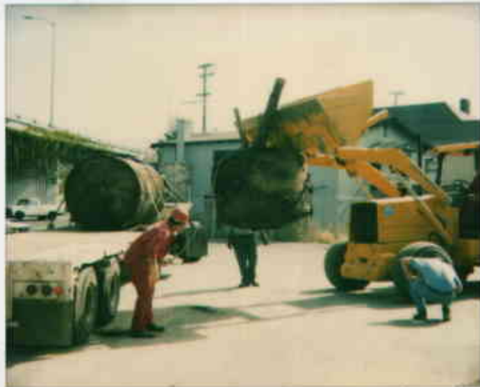
5427 Telegraph Ave. Oakland Front Tank #2. provide Bldg 94609 5/10/92
