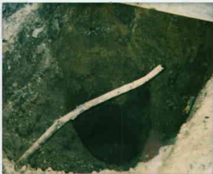
5427 Telegraph Ave Oakland 94609 oil tank pit.
