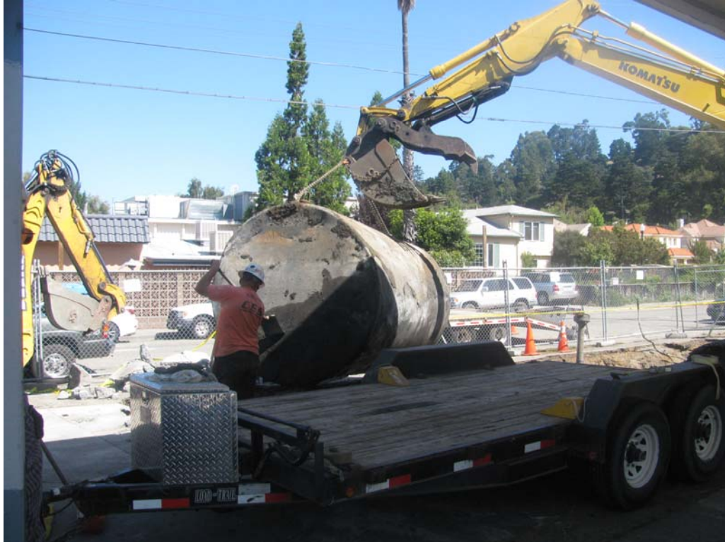
Plate 10. Lifting the smaller UST (3,000-gallons) out of the ground
