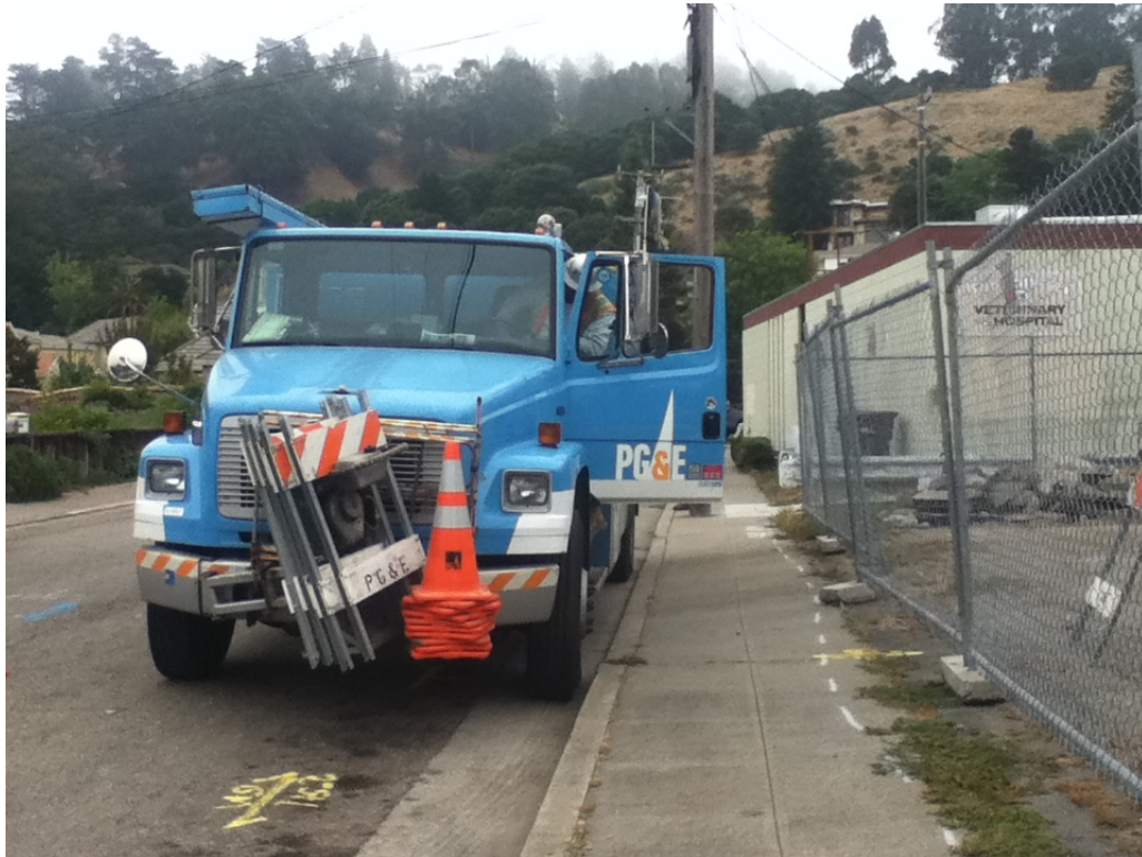
Plate 5. PG&E arrived for gas line disconnection
