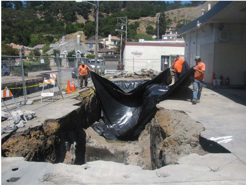
Plate 15. Layering the bottom of excavation with visqueen
