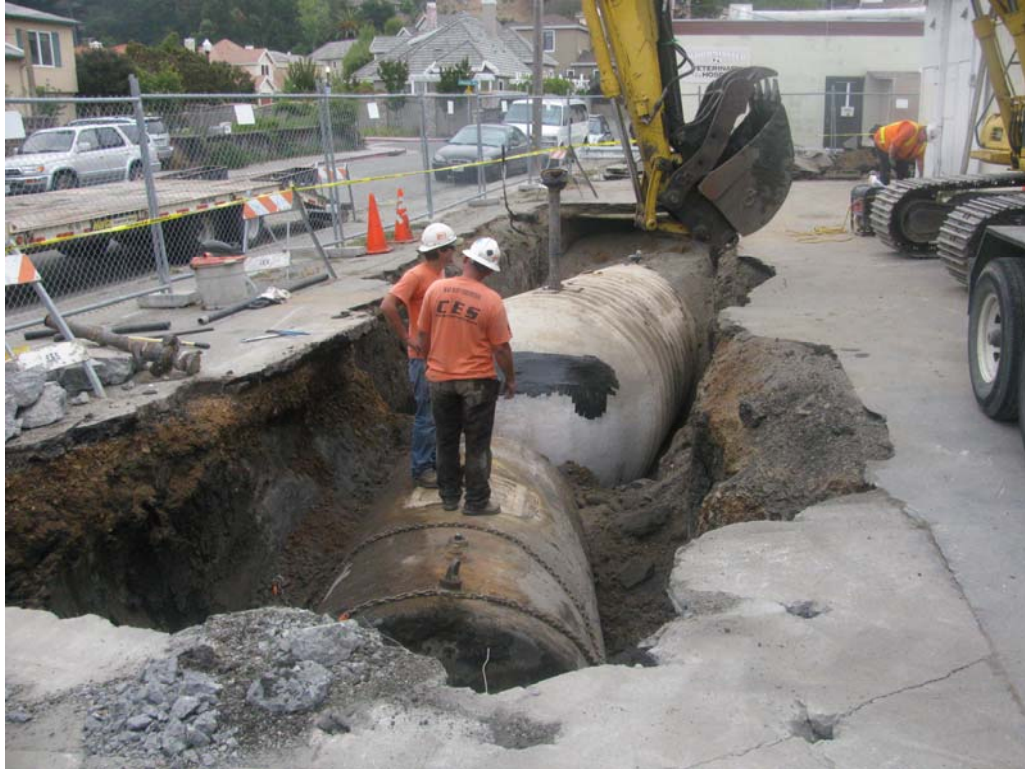
Plate 9. UST pit with tanks still in place
