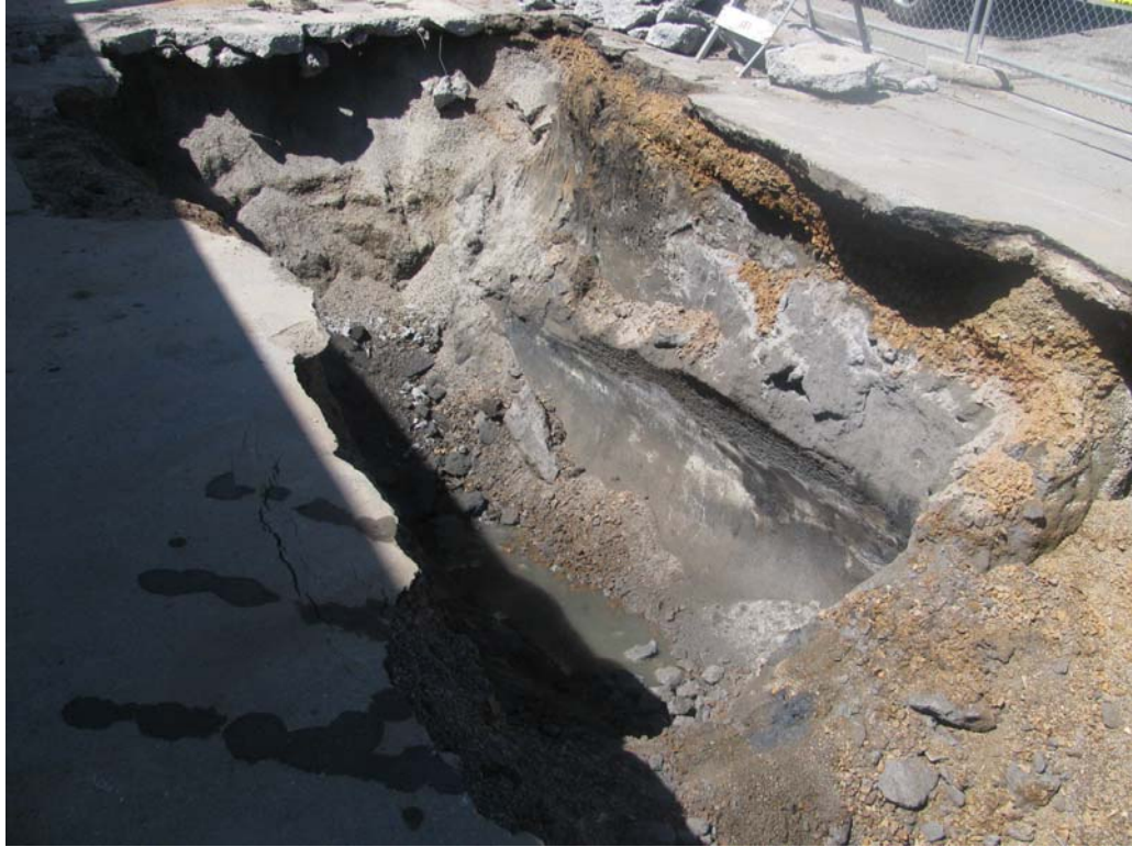
Plate 13. UST pit upon removal of second UST
