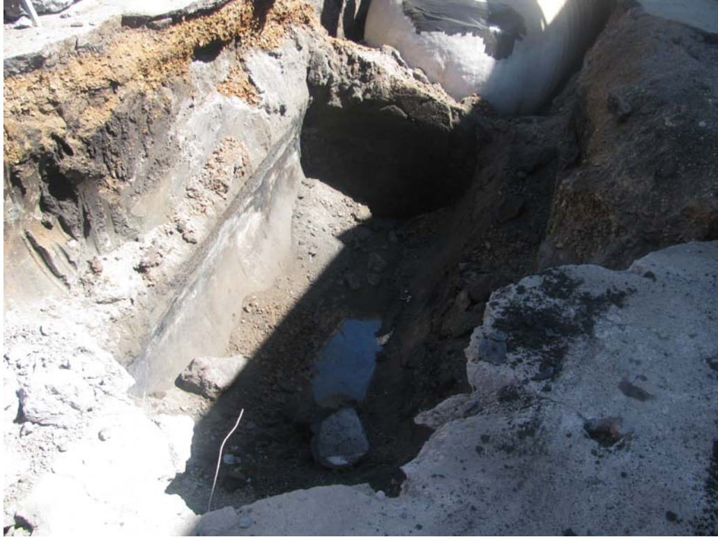
Plate 11. UST pit upon removal of first UST
