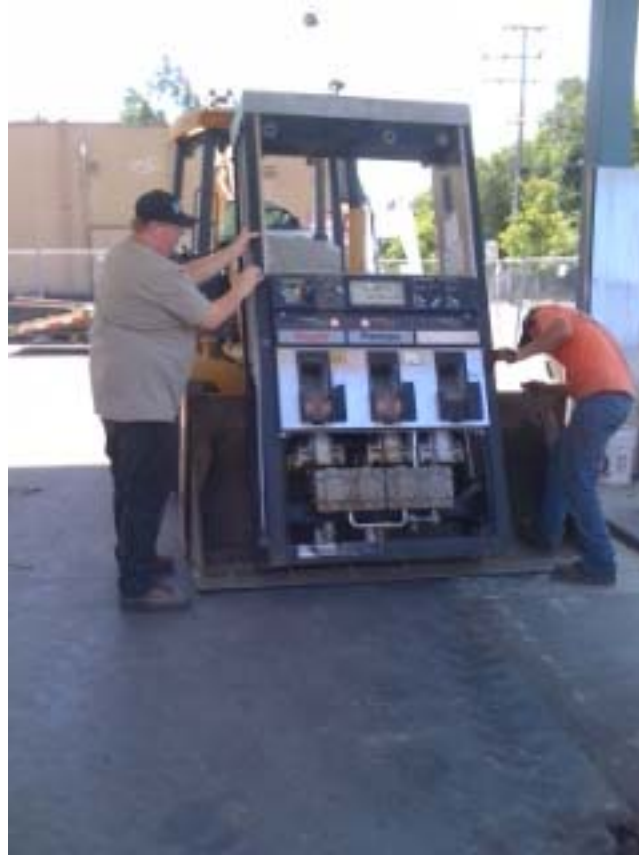
Plate 1. Removing pumps
