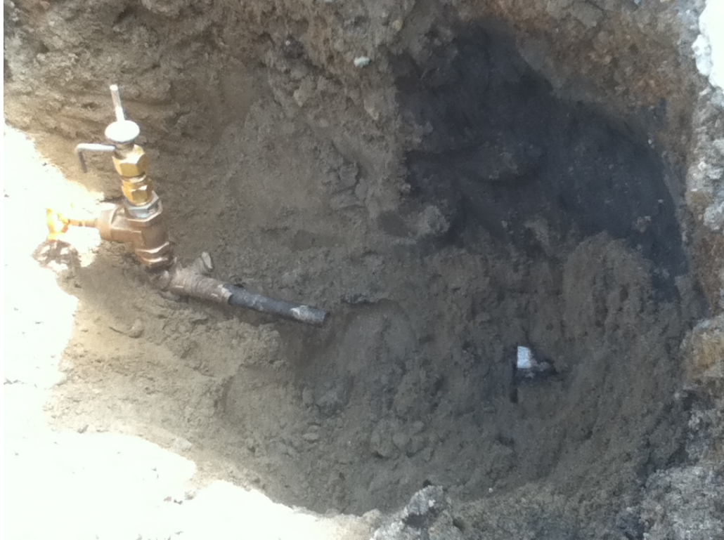
Plate 7. PG&E excavation showing the disconnected line
