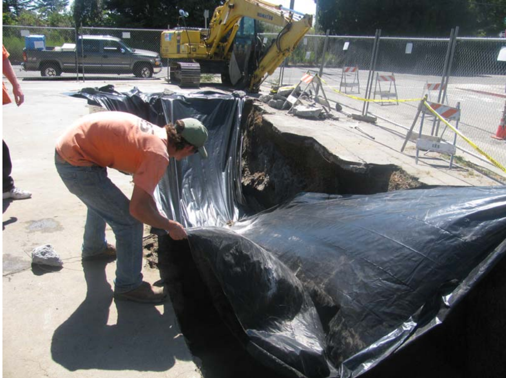
Plate 14. Layering the bottom of excavation with visqueen
