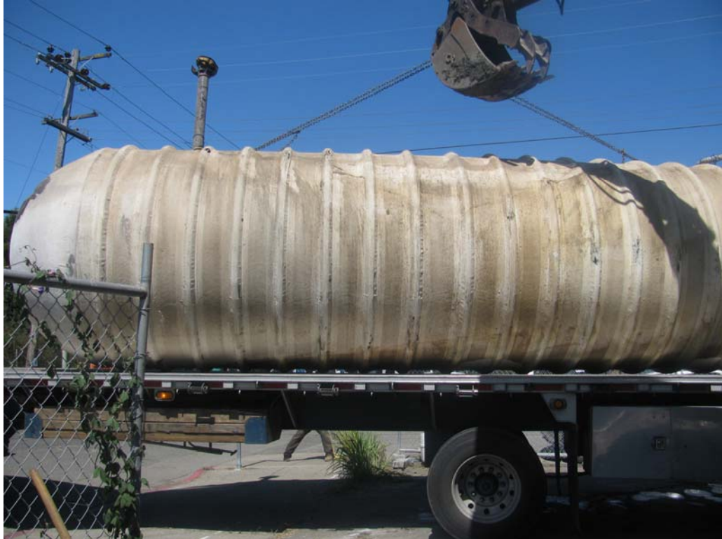
Plate 12. Larger UST removed (10,000-gallons)
