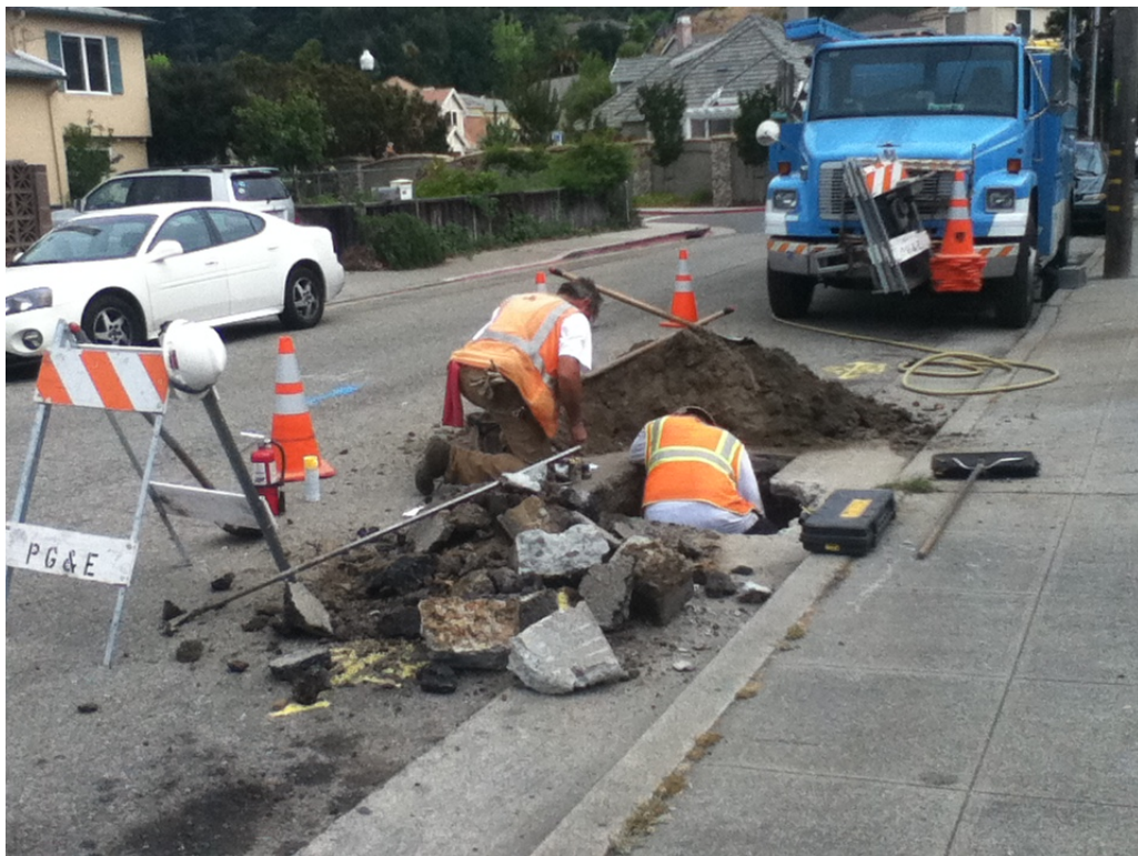
Plate 6. PG&E excavating in order to reach the gas line
