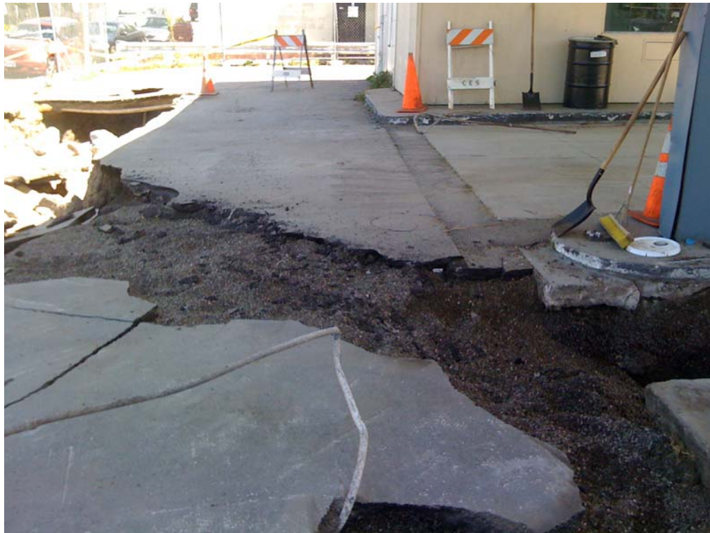
Plate 18. Backfilled fuel trenches
