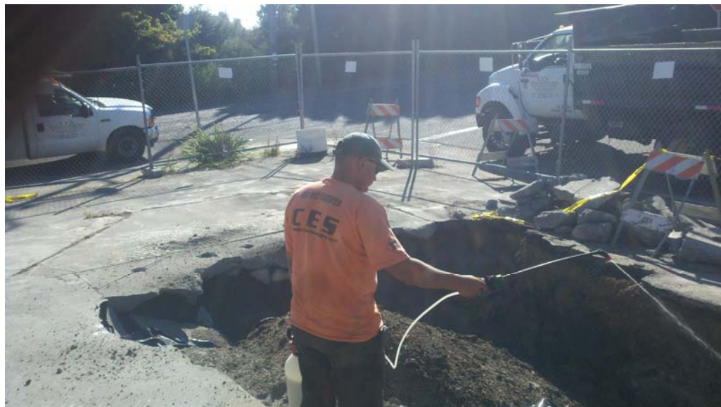
Plate 4. Application of vapor suppressant during excavation
