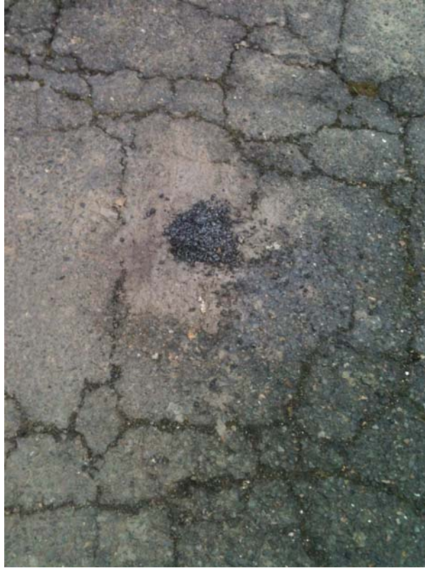
Plate 7. DPT-4 grouted to grade, finished to surface with asphalt patch
