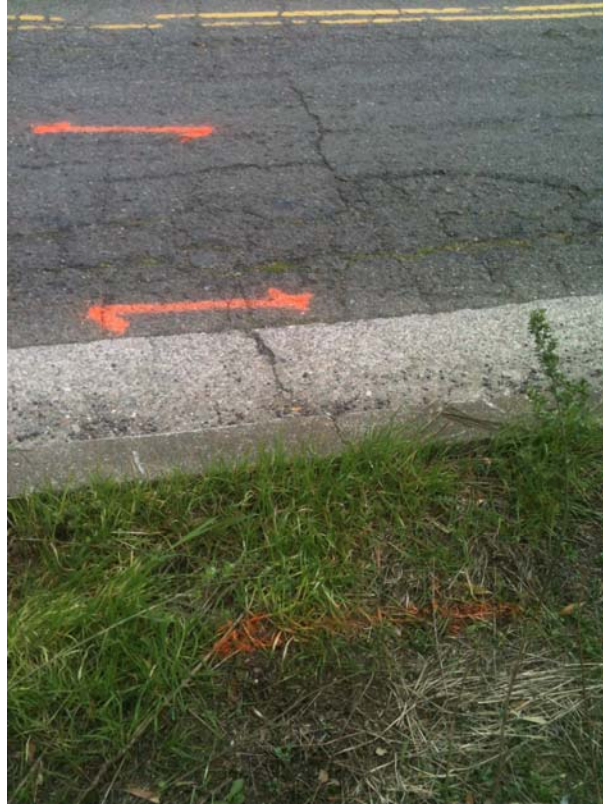
Plate 5. Utility clearance markings on Mountain Blvd.
