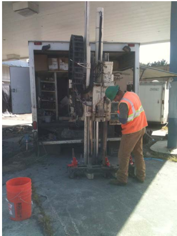
Plate 4. Fisch Drilling set up for CPT/MIP on CPT-1, view facing east
