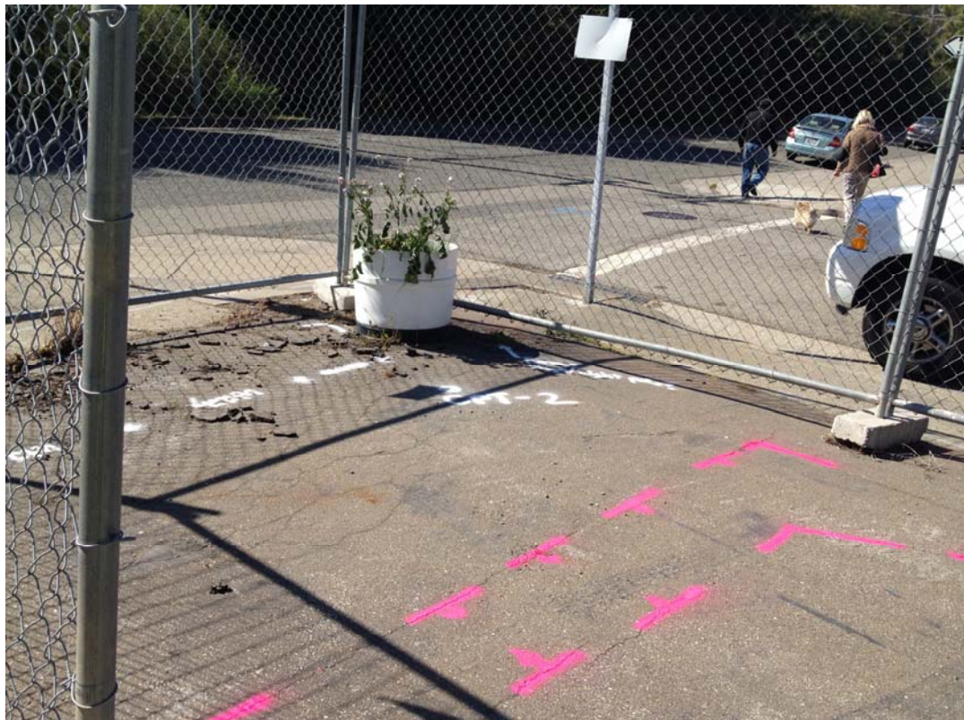
Plate 2. Utility clearance markings next to CPT-2
