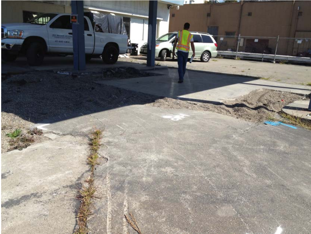
Plate 1. Cruz Bros. Utility Locators onsite for utility clearance
