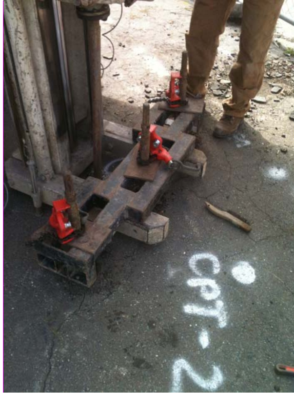
Plate 3. Bracing system for CPT/MIP
