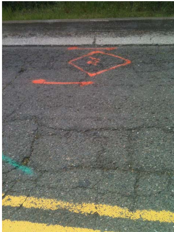
Plate 4. Utility clearance markings on Mountain Blvd.
