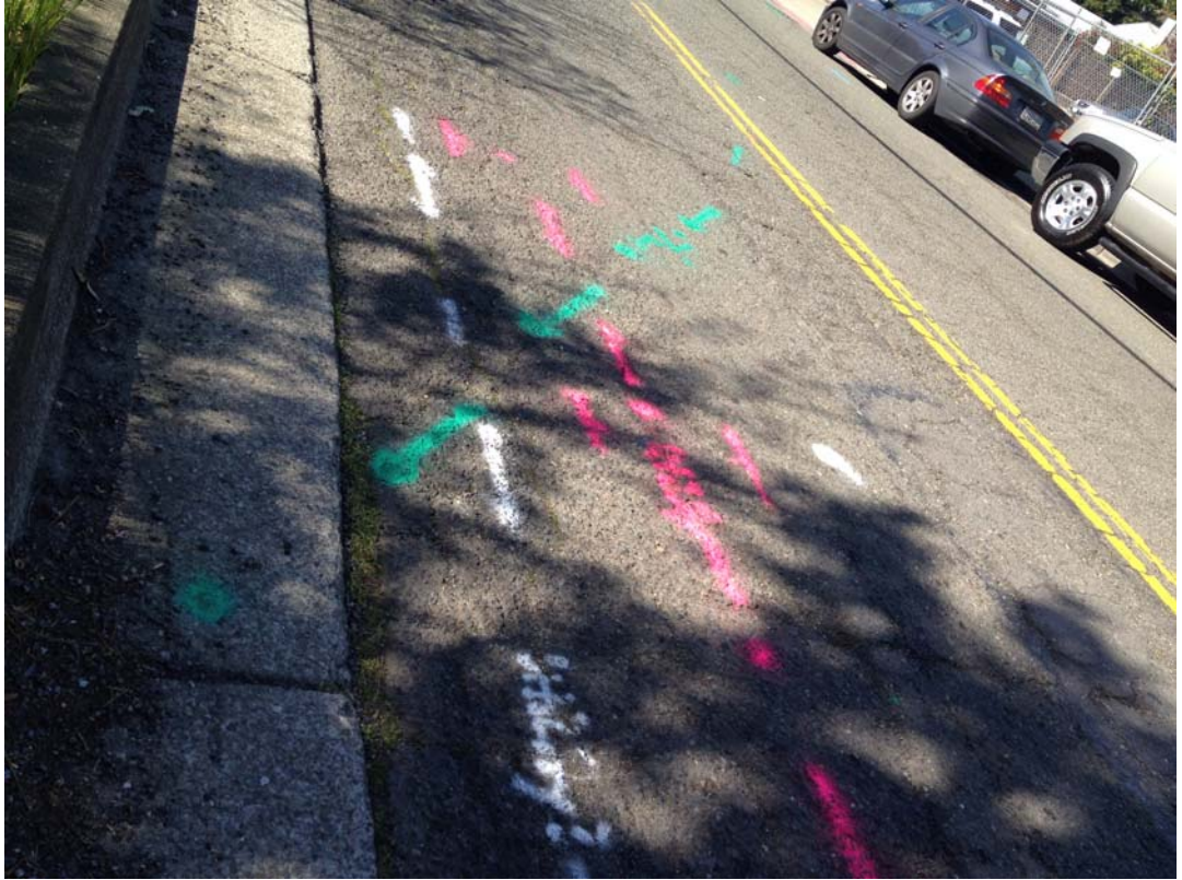
Plate 3. Utility clearance markings on Mountain Blvd.
