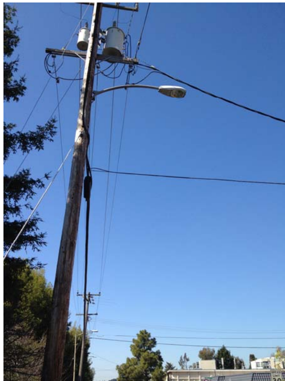
Plate 10. Overhead utilities along Mountain Blvd
