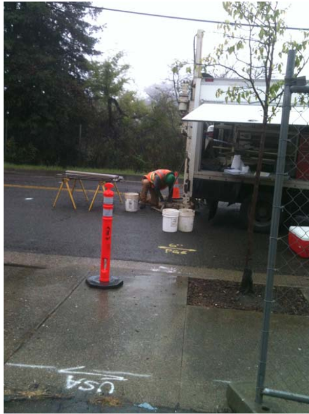
Plate 5. Fisch drilling set up on DPT-4, view facing southwest
