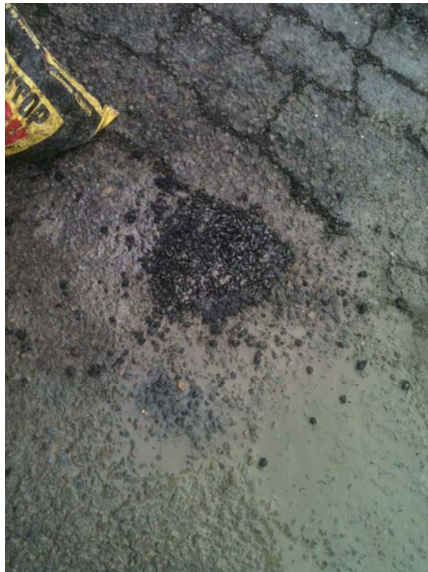
Plate 8. DPT-3 grouted to grade, finished to surface with asphalt patch
