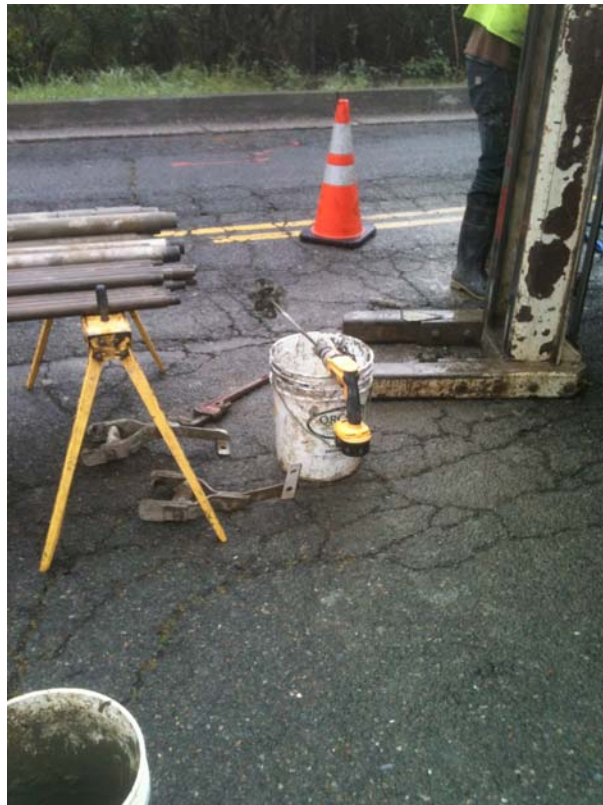
Plate 6. Fisch Drilling preparing to grout DPT-4
