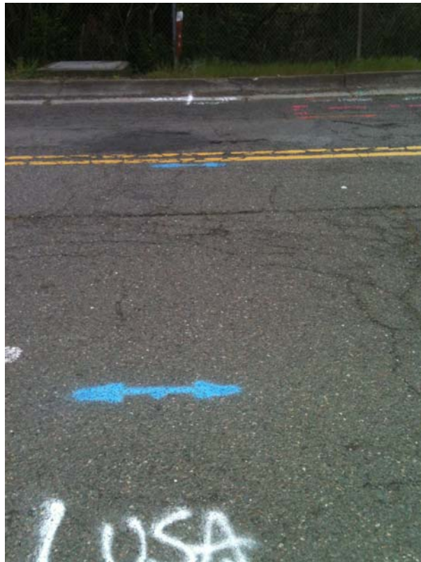
Plate 6. Utility clearance markings on Mountain Blvd.
