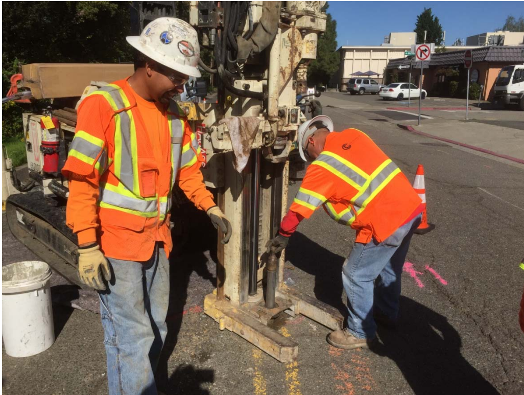
Drilling along the Mountain Blvd
