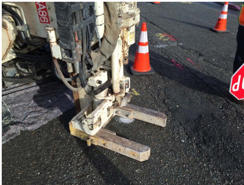
DPT rig is getting ready to drill first boring
