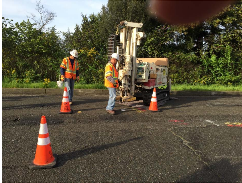
Drilling operation along Mountain Blvd
