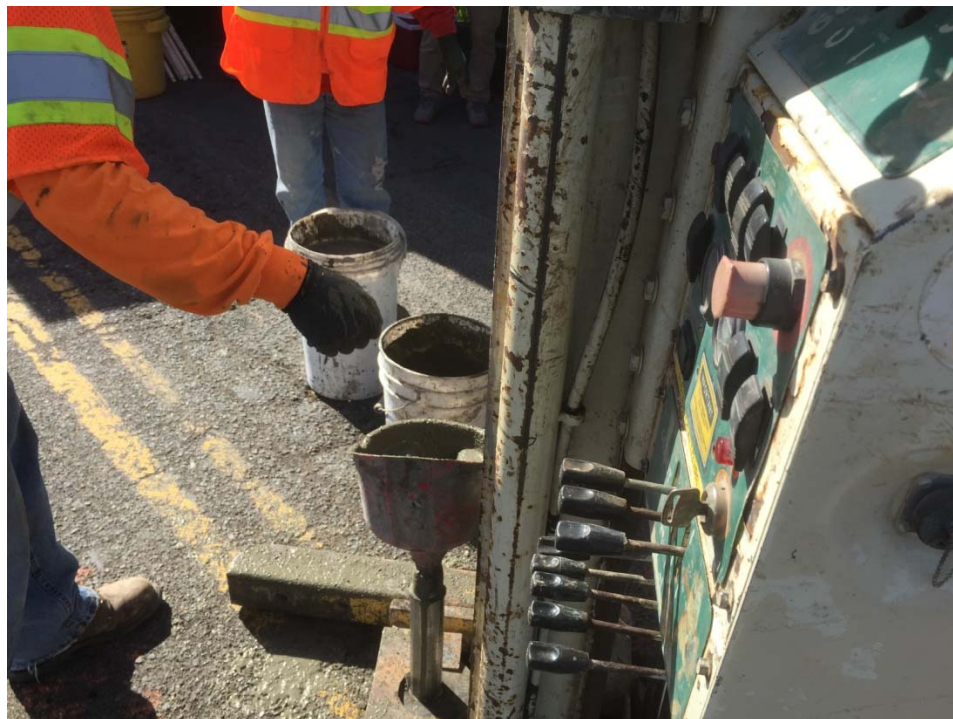
Grouting one of the DPT boreholes
