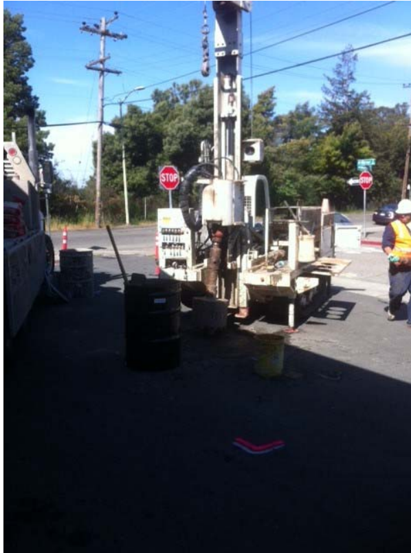
Plate 1. Gregg Drilling setting up on MW-3
