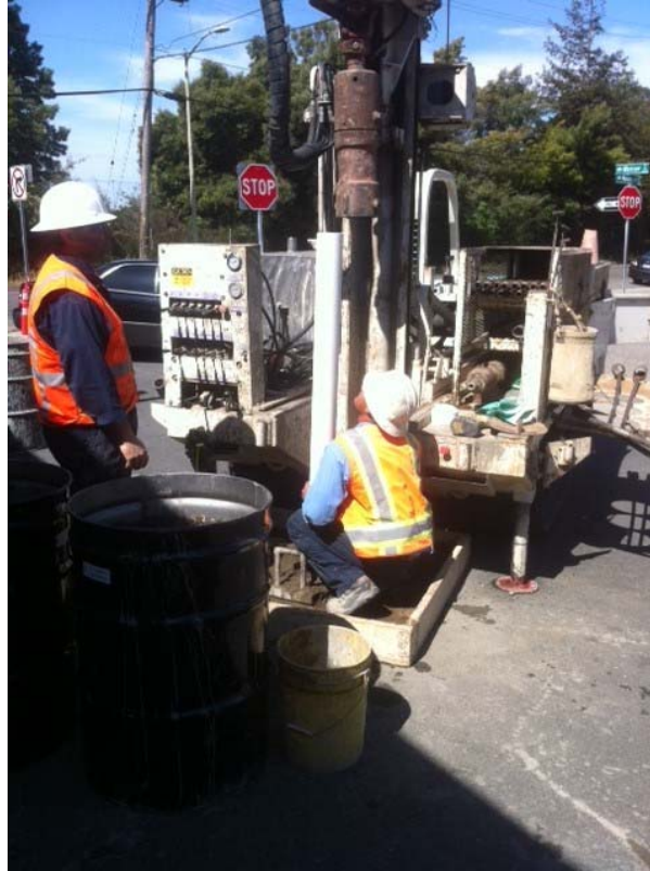
Plate 3. Gregg Drilling putting PVC casing into MW-3
