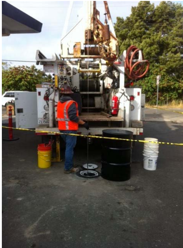
Plate 7. Gregg Drilling bailing & surging MW-3
