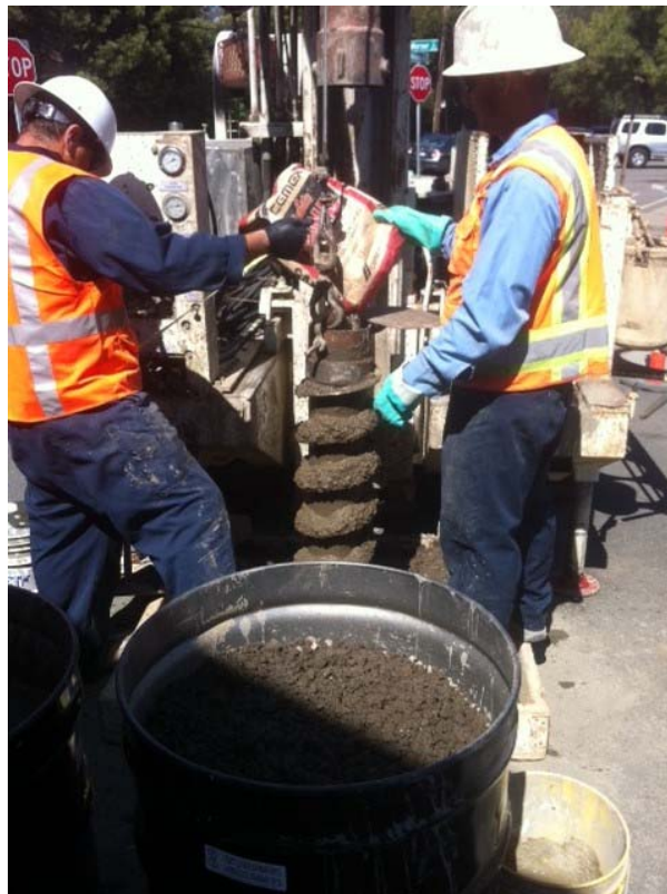
Plate 4. Gregg Drilling adding sand to MW-3
