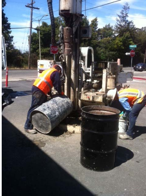
Plate 5. Gregg Drilling pouring grout into MW-3
