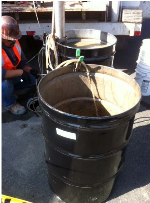
Plate 8. Gregg Drilling pumping groundwater from MW-3
