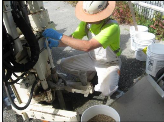
Shallow soil vapor point installation via GeoProbe drill rig
