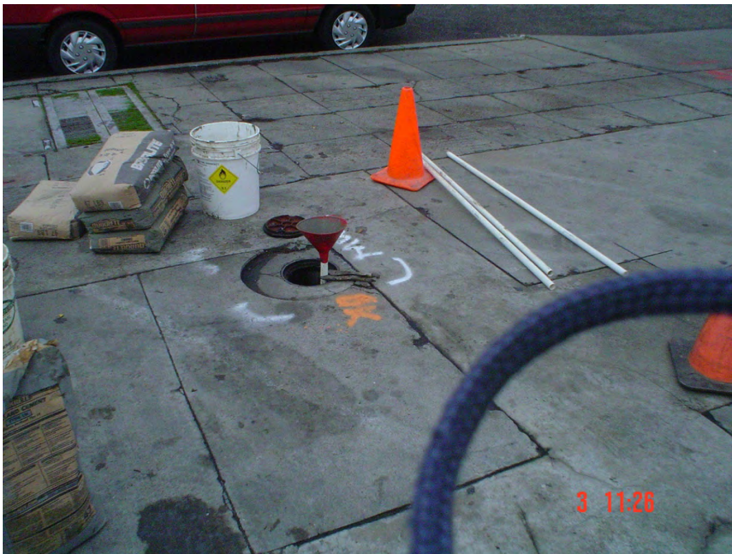
Plate 9. View of MW-7 set to be tremie grouted
