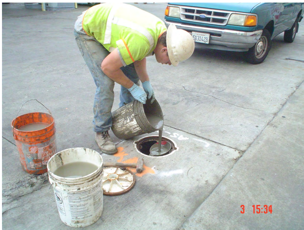
Plate 22. View of Fisch tremie grouting AS-5
