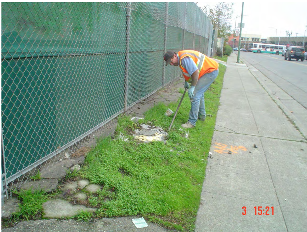
Plate 19. View of Fisch removing concrete from MW-10
