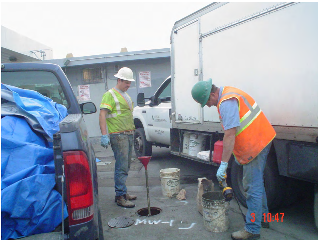
Plate 7. View of Fisch tremie grouting MW-1
