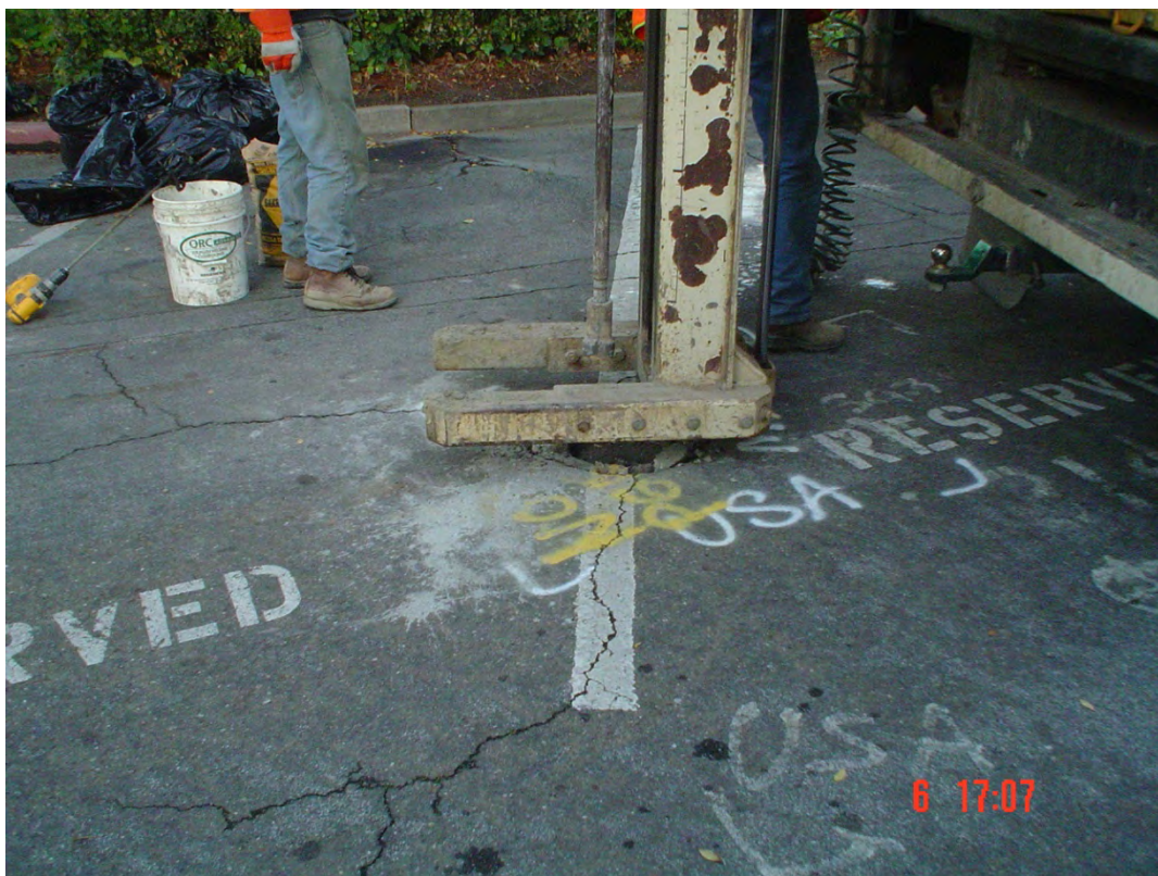
Plate 47. View of Fisch set up to remove MW-12 well box
