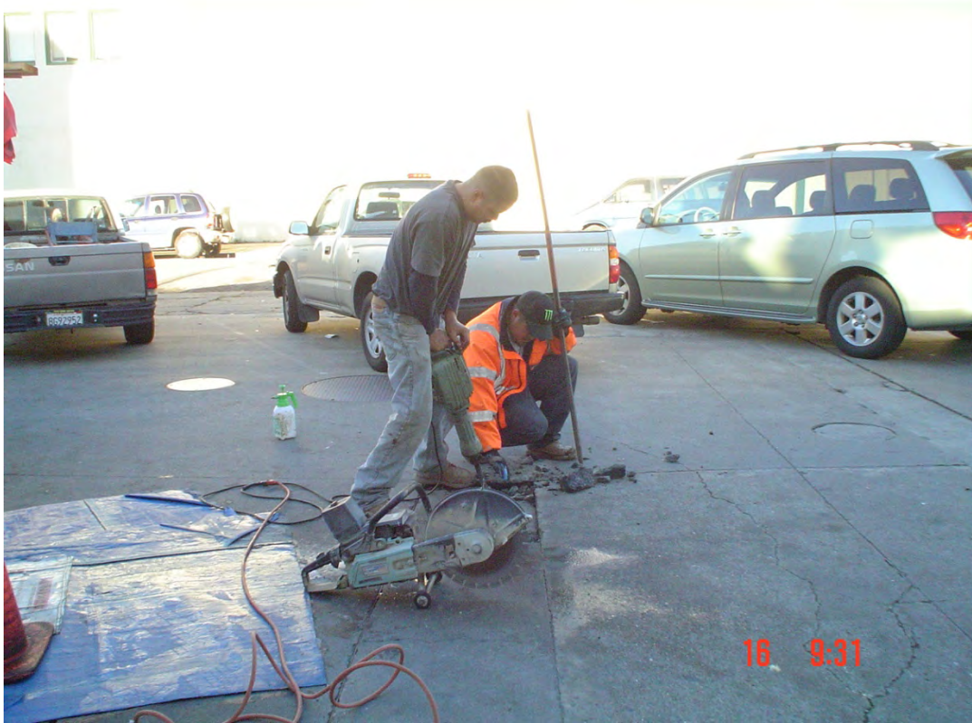
Plate 53. View of Jim's Quality Paving removing broken concrete
