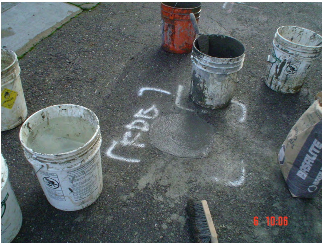
Plate 30. View of FDE finished to grade
