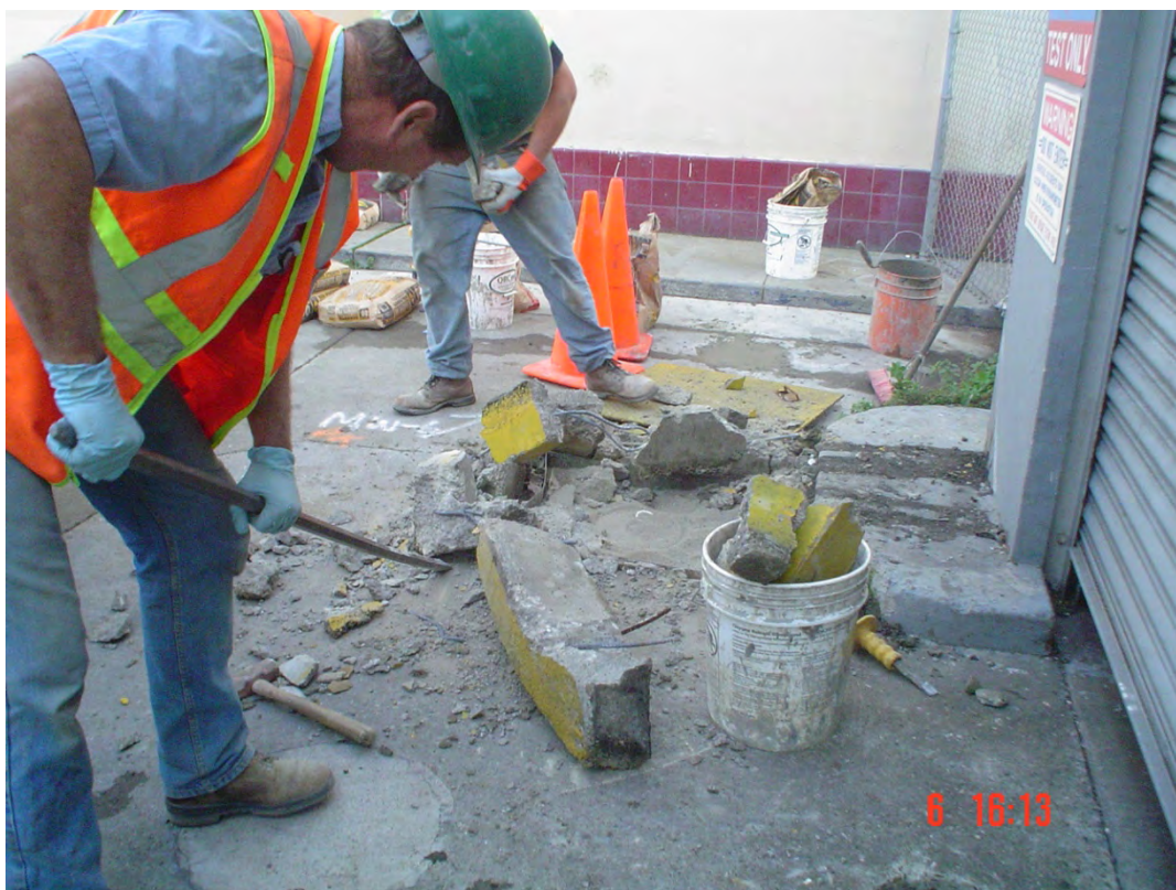
Plate 46. View of Fisch removing well box for manifold
