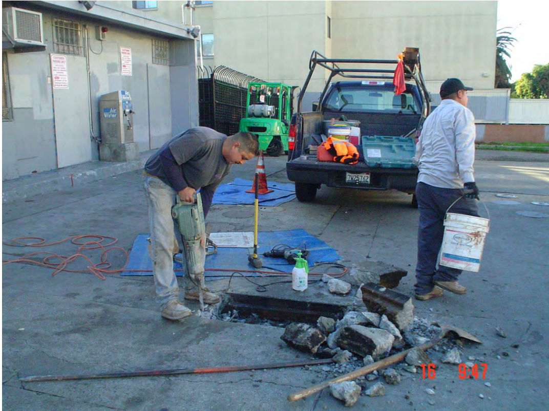
Plate 55. View of concrete removal and edge finishing
