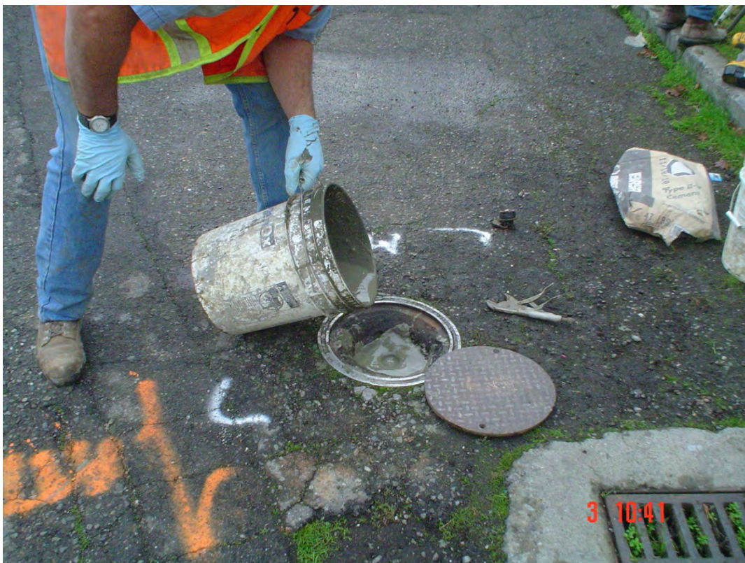
Plate 6. View of MW-8 grouted to top of casing
