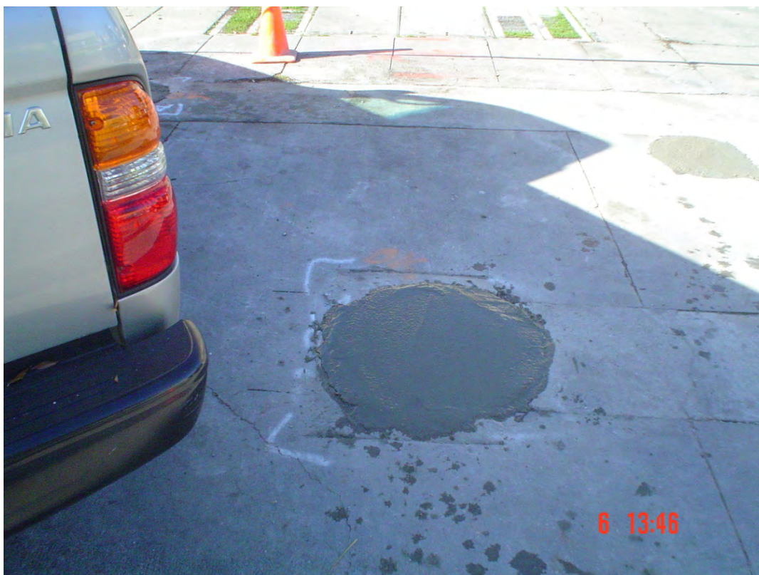
Plate 38. View SVE-2 finished to grade
