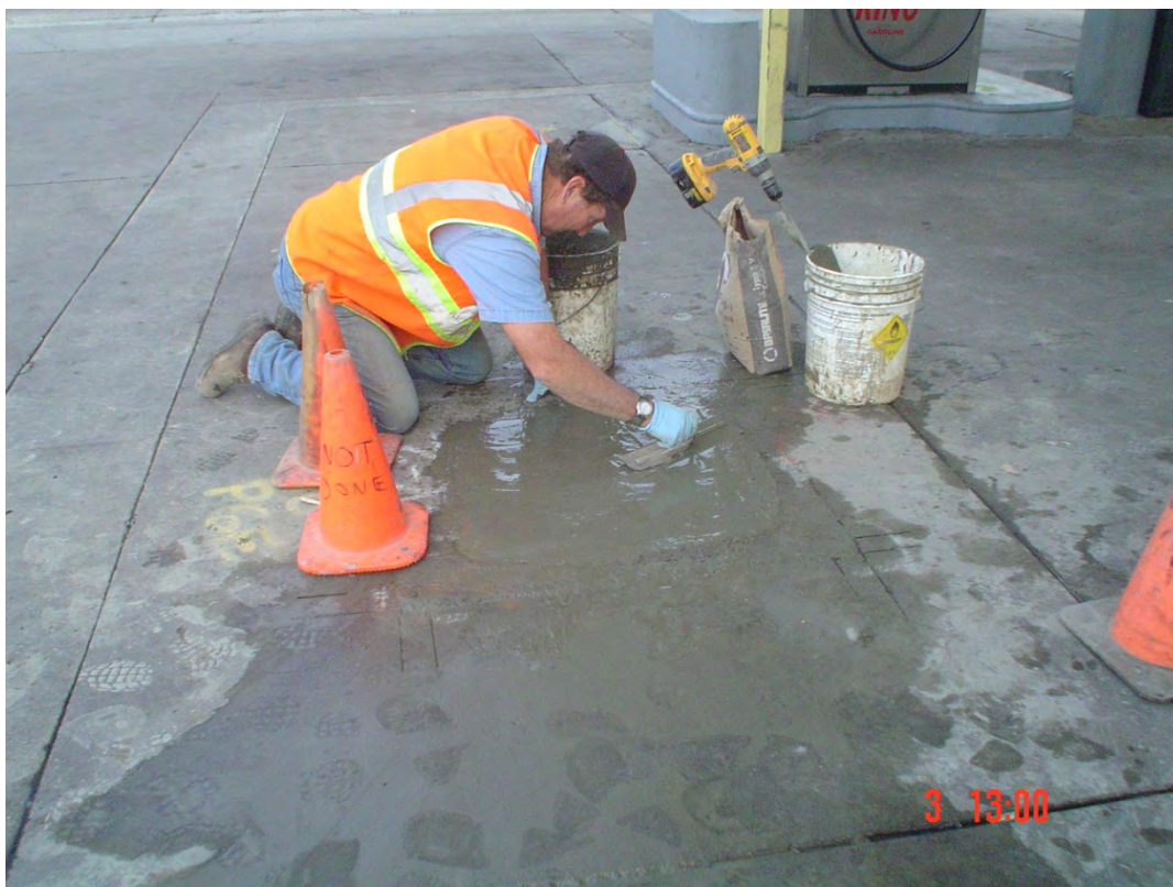
Plate 13. View of MW-2 finished to grade
