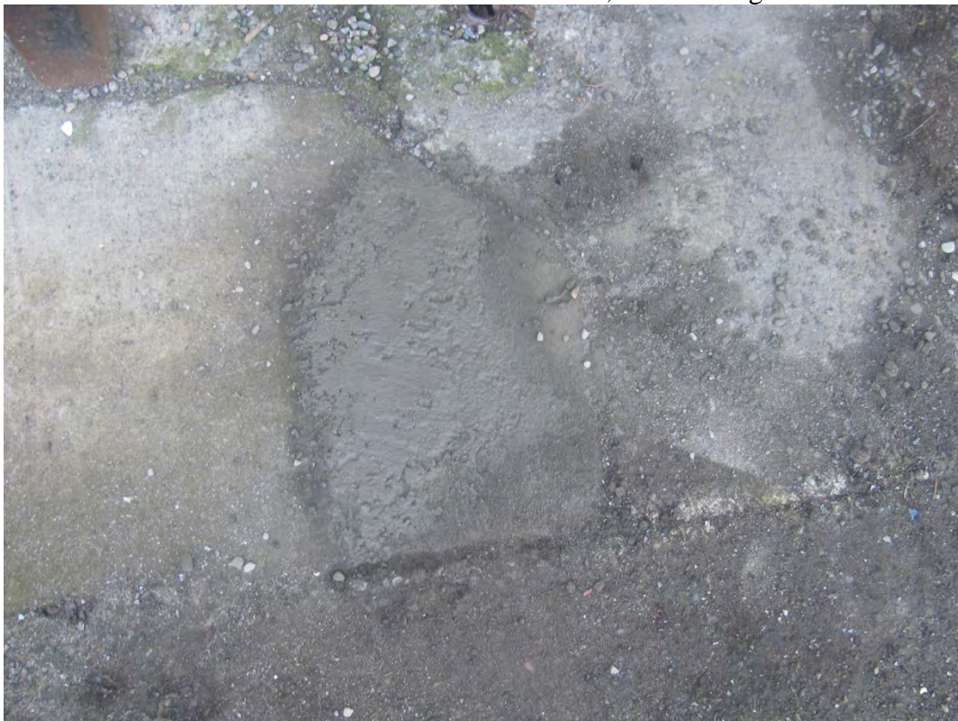
Plate 58. Repaired area of former treatment system piping
