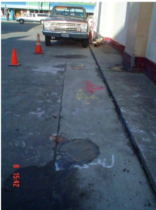
Plate 44. View of AS-4 and AS-5 finished to grade
