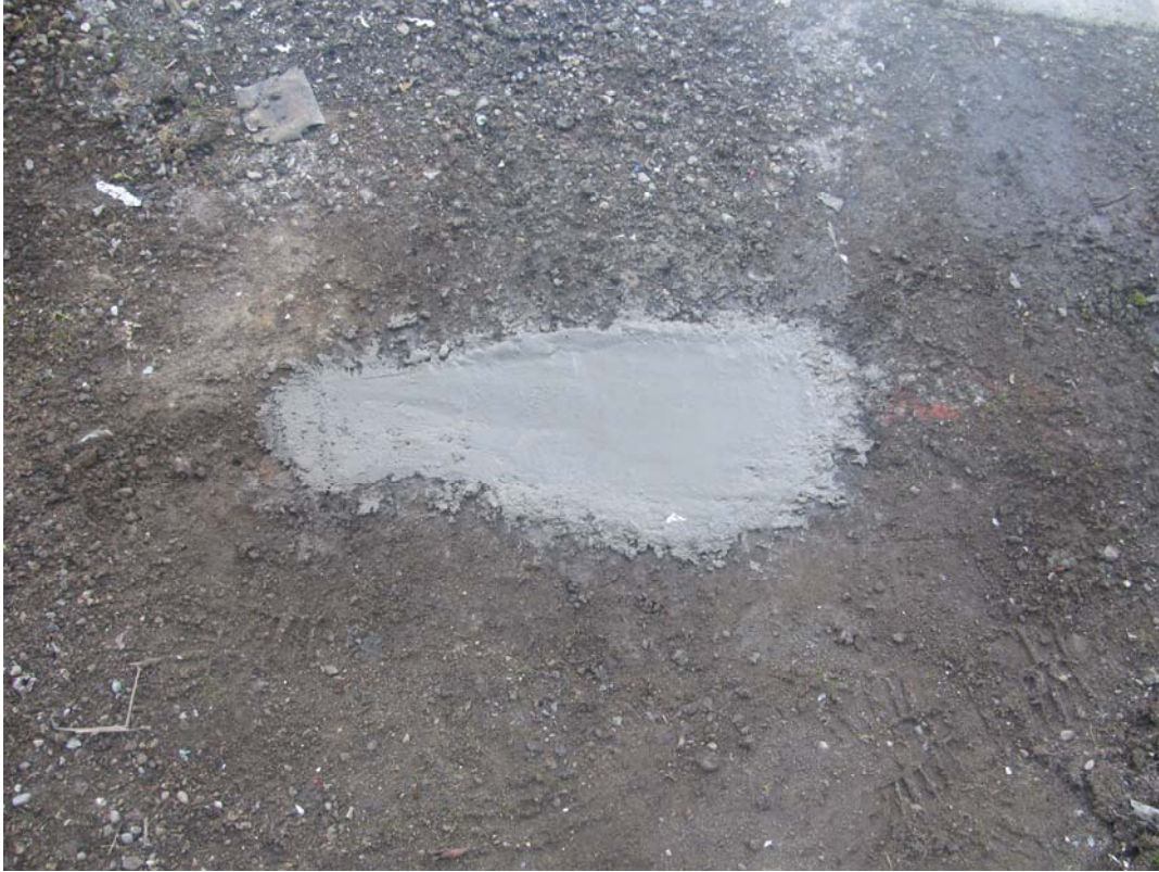
Plate 59. Repaired area of former treatment system piping
