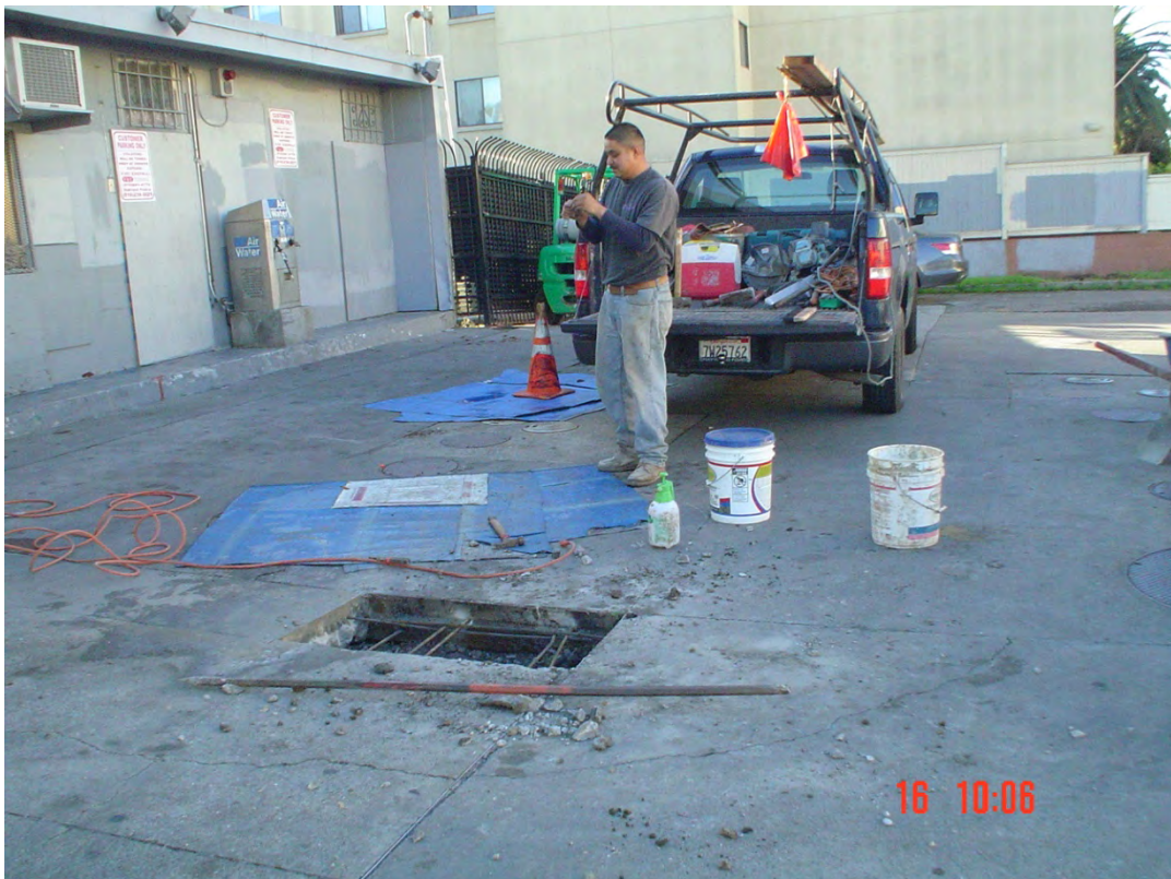
Plate 56. View of rebar in concrete prior to finishing
