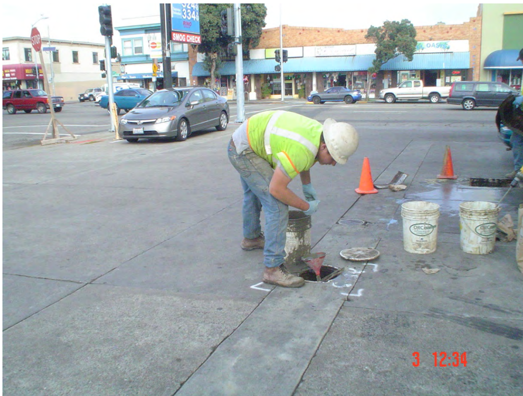
Plate 14. View of Fisch tremie grouting AS-3
