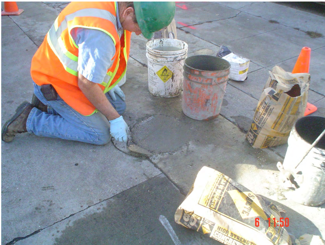
Plate 34. View of AS-1 finished to grade
