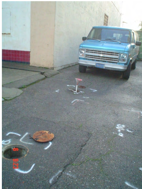
Plate 26. View of Fisch set up to tremie grout MW-4R
