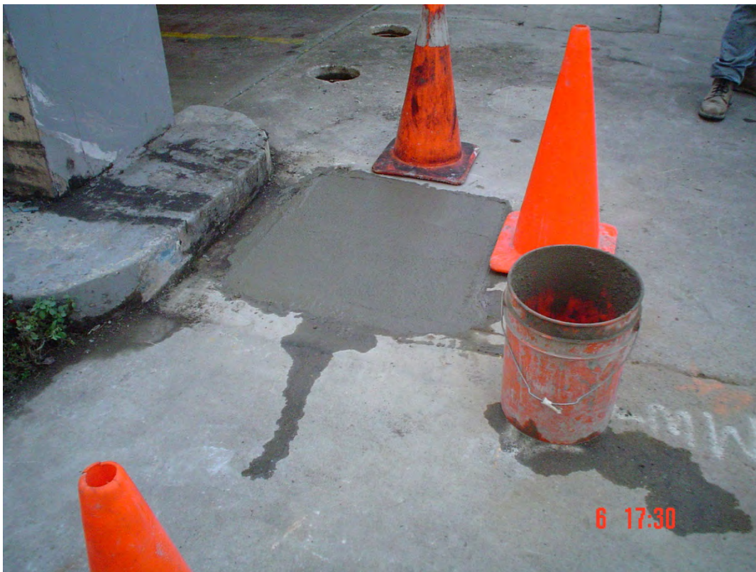
Plate 49. View of manifold box finished to grade
