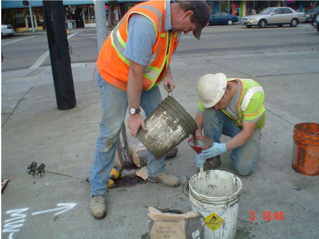
Plate 25. View of Fisch tremie grouting MW-5
