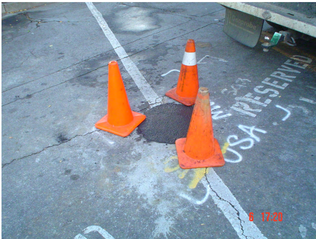
Plate 48. View of MW-12 finished to grade
