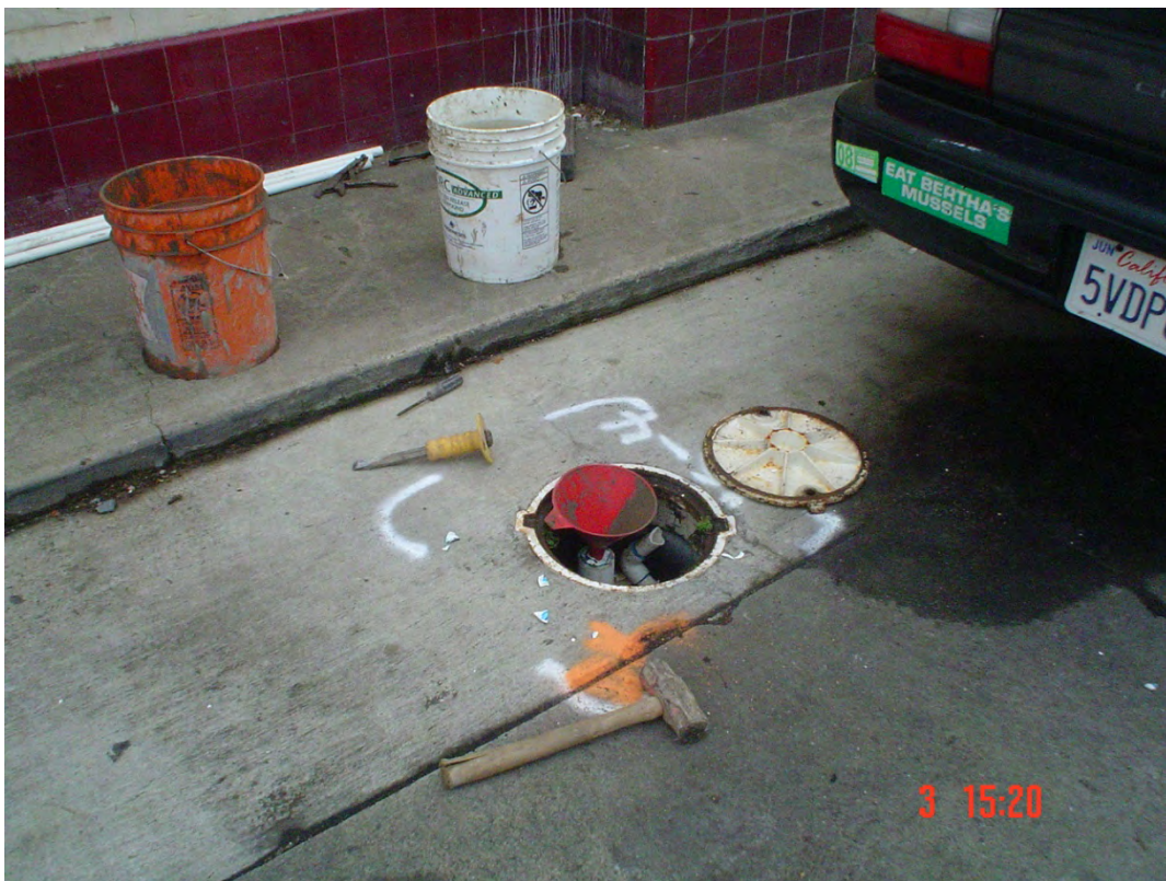
Plate 18. View of Fisch set up on AS-4 to tremie grout
