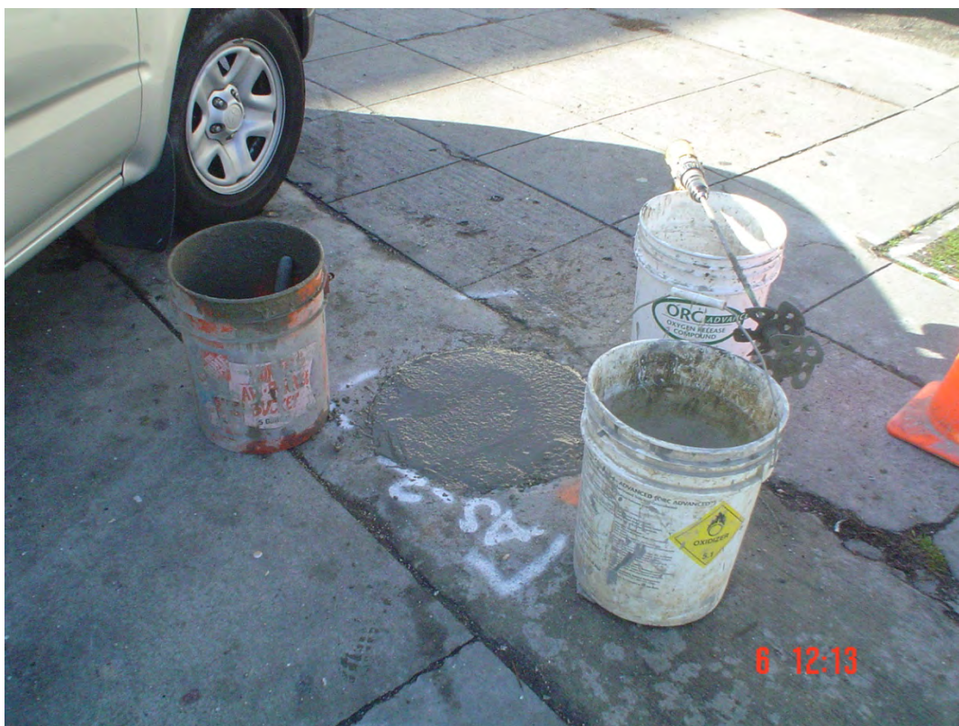
Plate 36. View of AS-2 finished to grade
