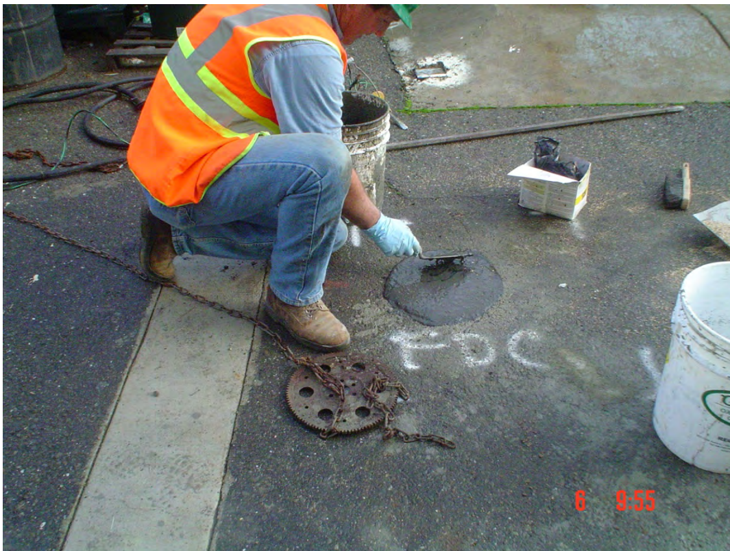
Plate 29. View of FDC finished to grade
