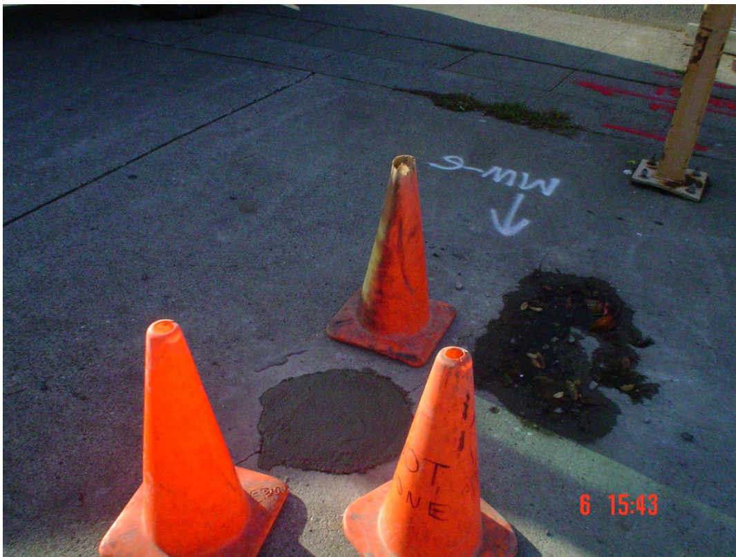
Plate 43. View of MW-6 finished to grade
