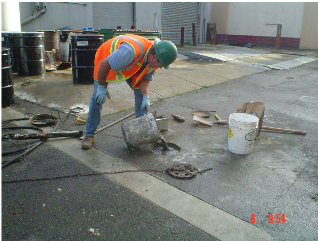
Plate 28. View of Fisch cementing FDC to surface
