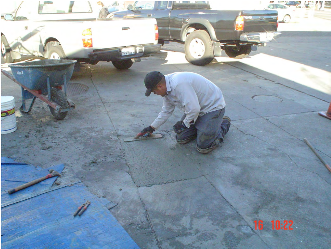
Plate 57. View of concrete restoration, finished to grade
