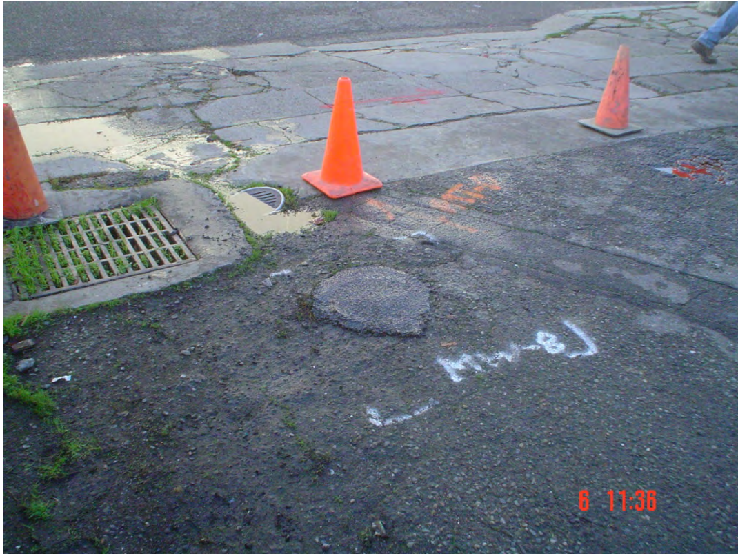
Plate 33. View of MW-8 finished to grade
