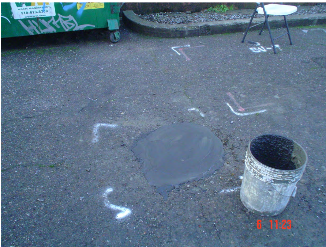
Plate 31. View of MW-4R finished to grade
