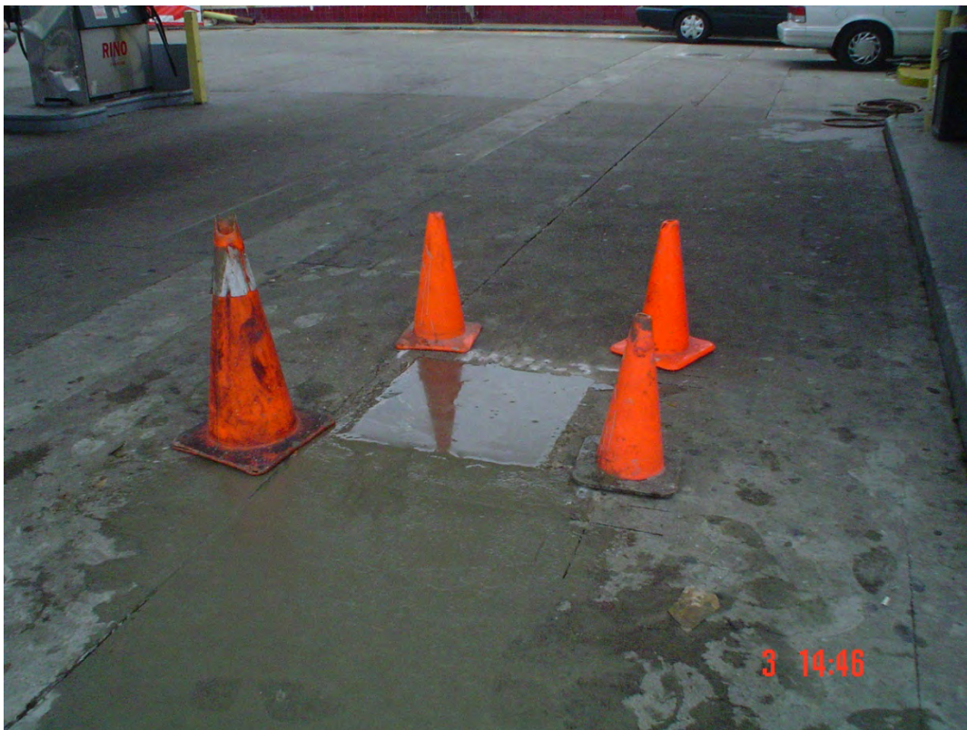
Plate 17. View of MW-3 finished to grade
