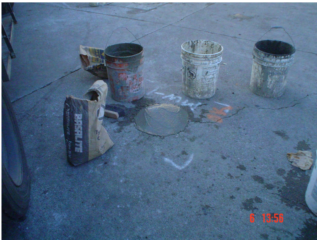
Plate 39. View of MW-1 finished to grade
