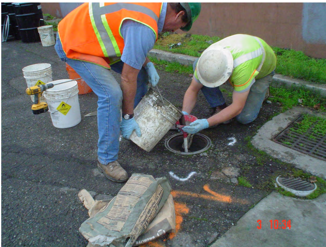
Plate 5. View of Fisch tremie grouting MW-8
