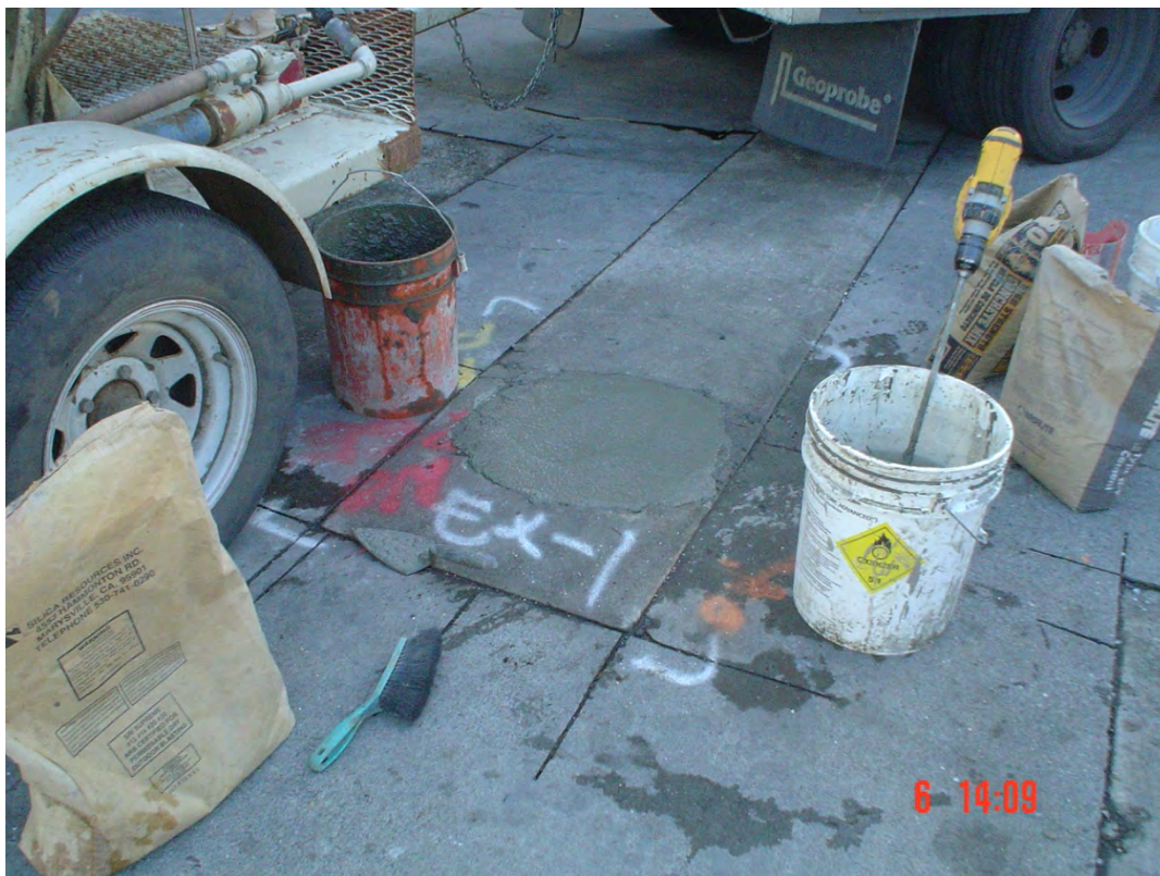
Plate 40. View of EX-1 finished to grade
