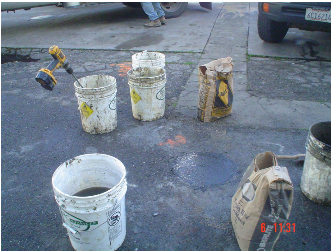
Plate 32. View of FDW finished to grade
