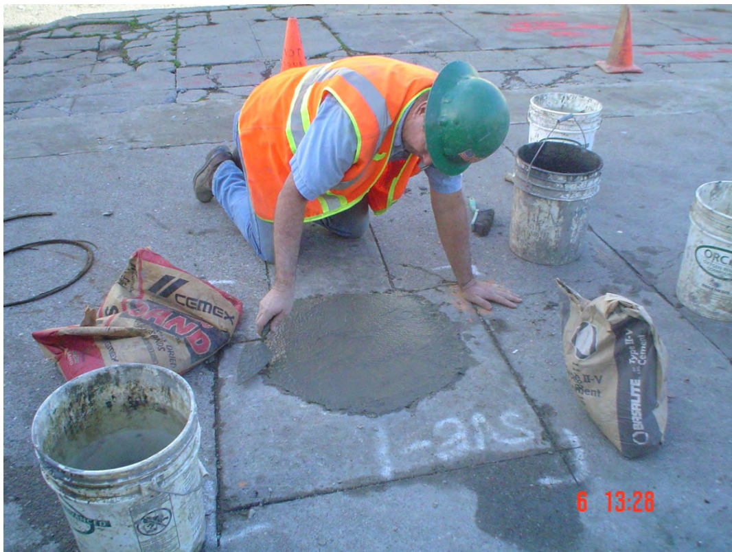
Plate 37. View of SVE-1 finished to grade
