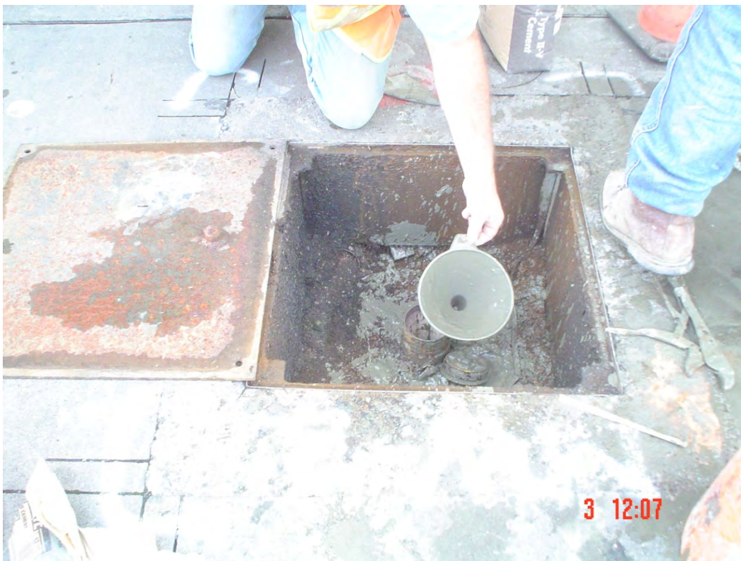
Plate 10. View of Fisch tremie grouting MW-2
