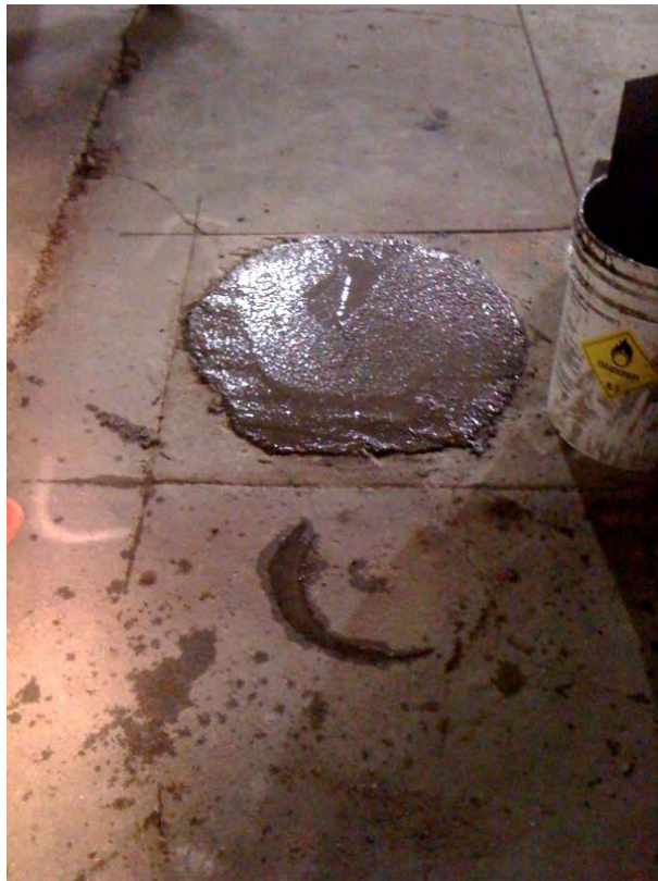
Plate 51. View of SVE-3 finished to grade
