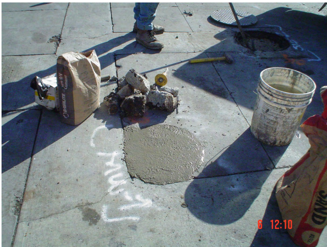
Plate 35. View of MW-7 finished to grade
