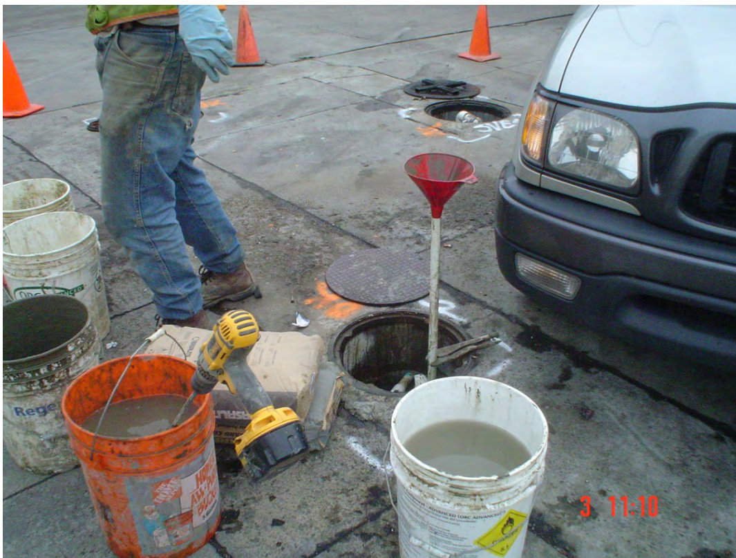
Plate 8. View of Fisch set up to tremie grout AS-2
