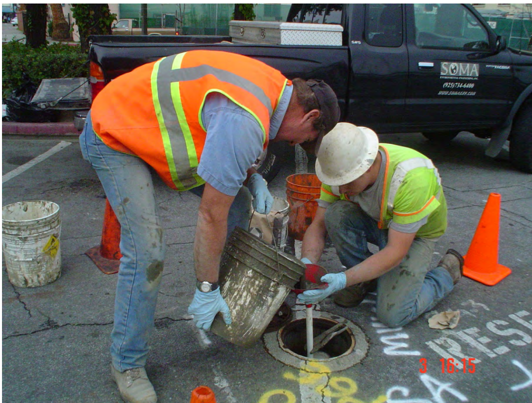
Plate 24. View of Fisch tremie grouting MW-12
