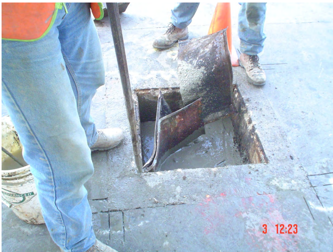
Plate 11. View of Fisch removing well box from MW-2
