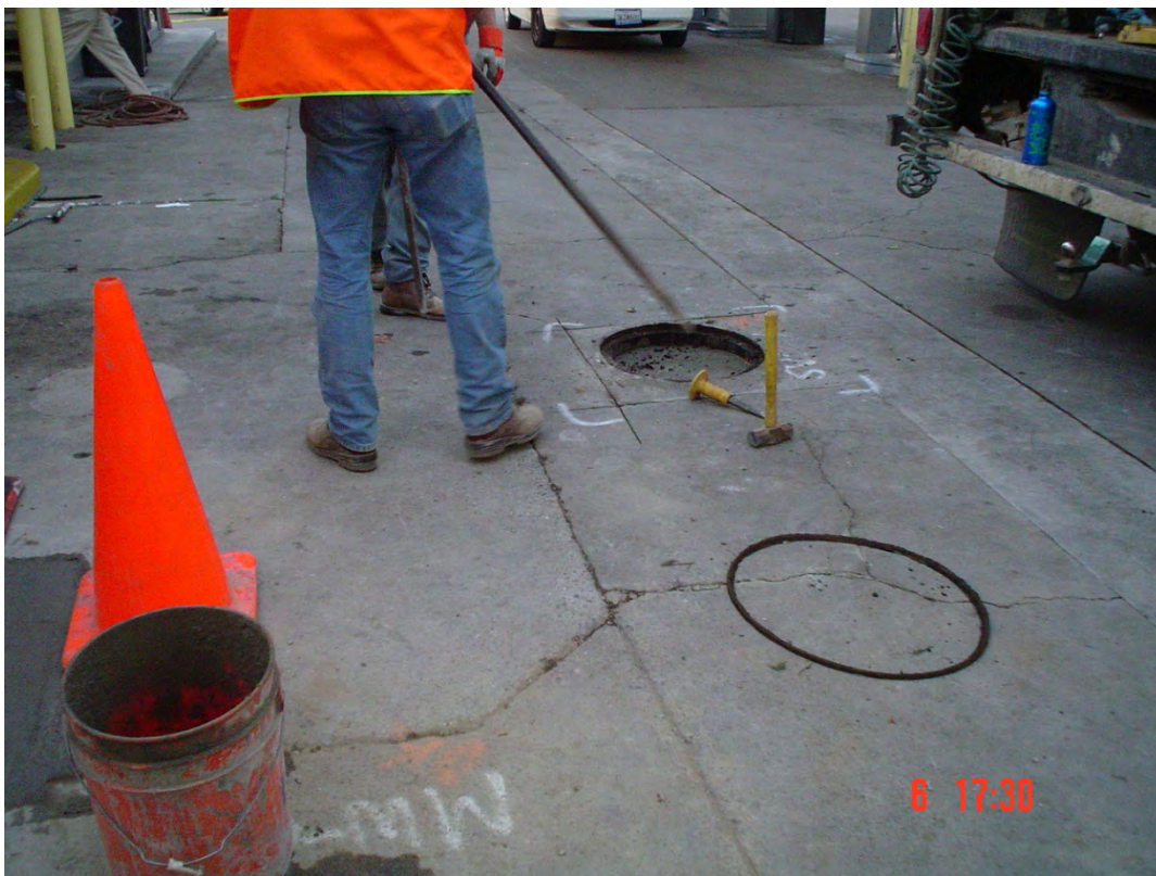
Plate 50. View of Fisch removing well box from SVE-3
