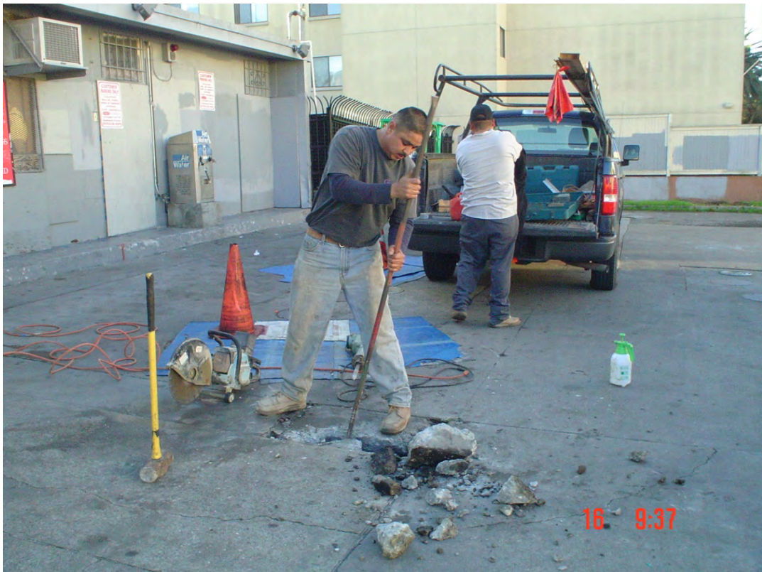
Plate 54. View of concrete removal
