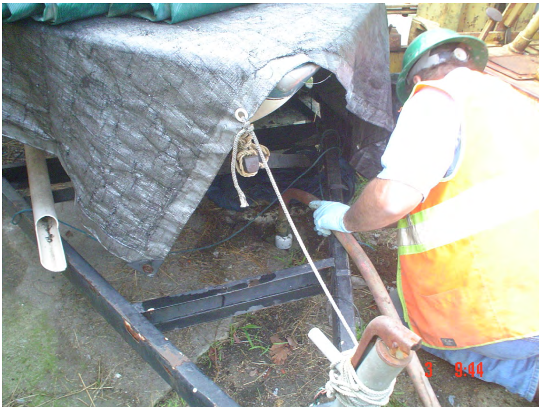
Plate 3. View of Fisch pressure grouting MW-11, 25 PSI held for 5 minutes
