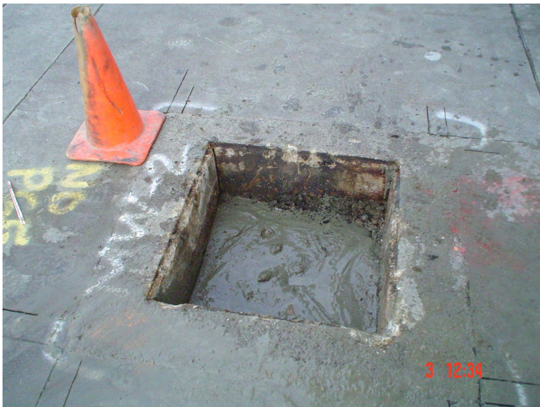
Plate 12. View of MW-2 with well box removed and well grouted
