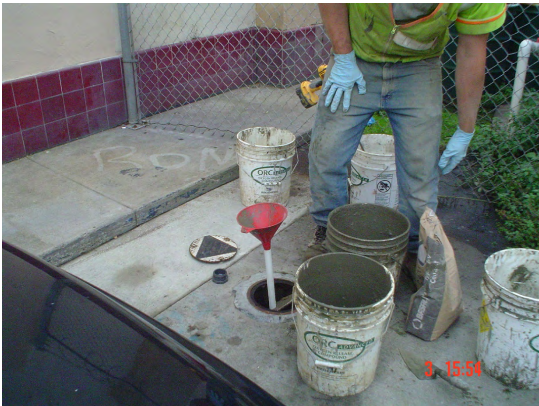
Plate 23. View of Fisch tremie grouting MW-6
