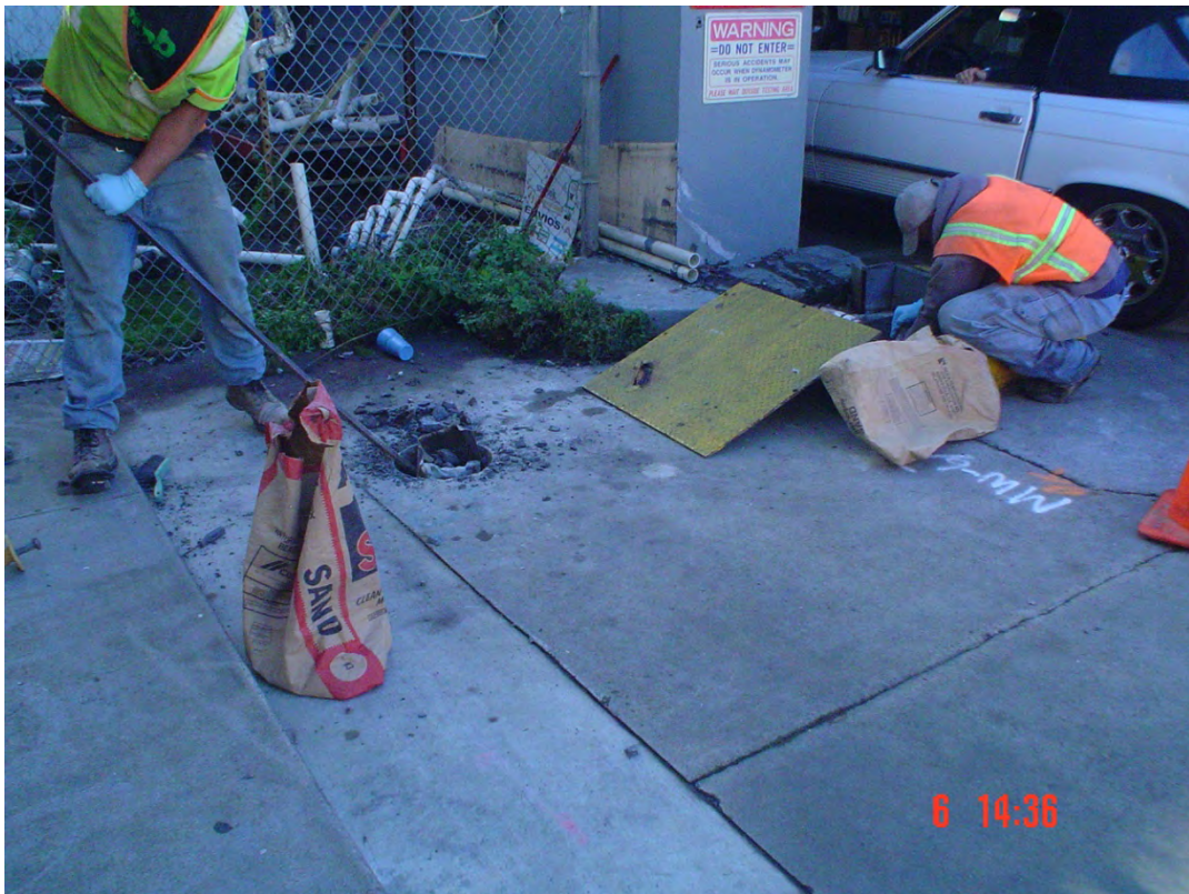
Plate 42. View of Fisch removing well box from MW-6
