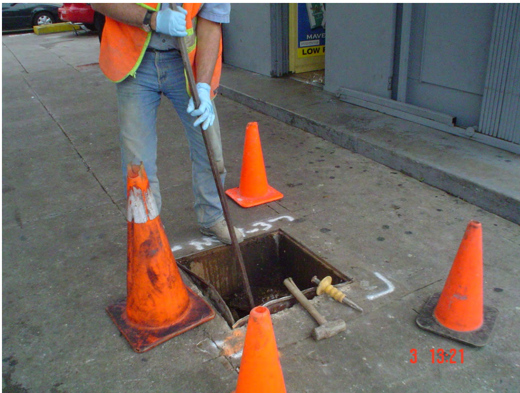
Plate 15. View of Fisch removing well box from MW-3 after tremie grouting
