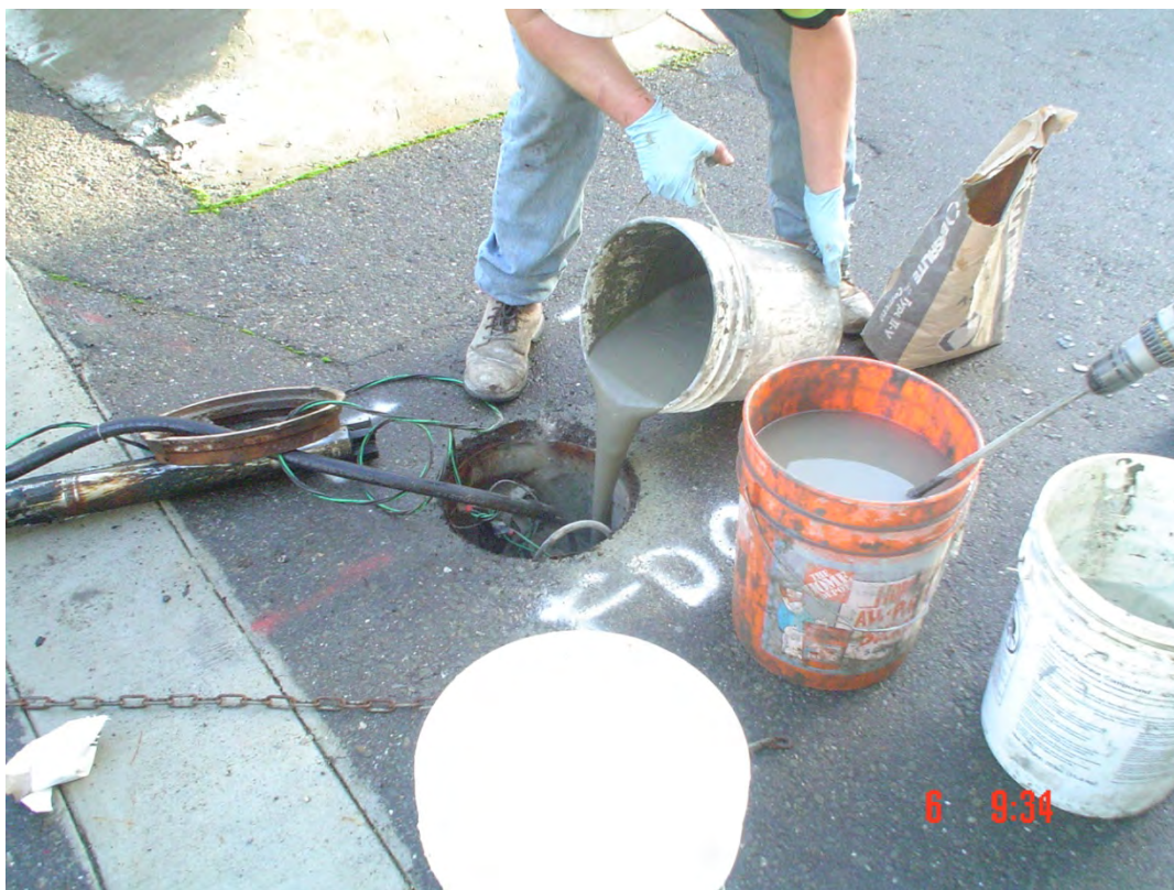
Plate 27. View of Fisch grouting top of FDC
