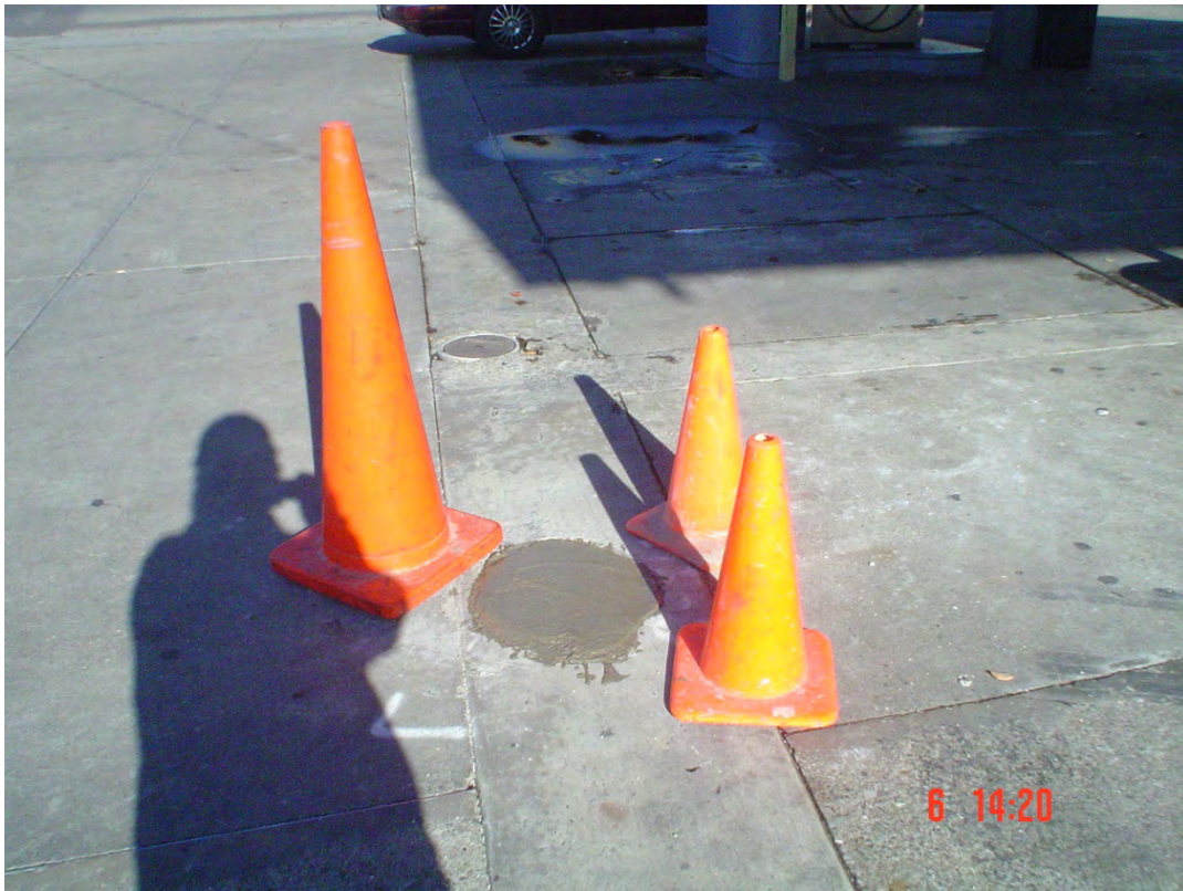
Plate 41. View of AS-3 finished to grade
