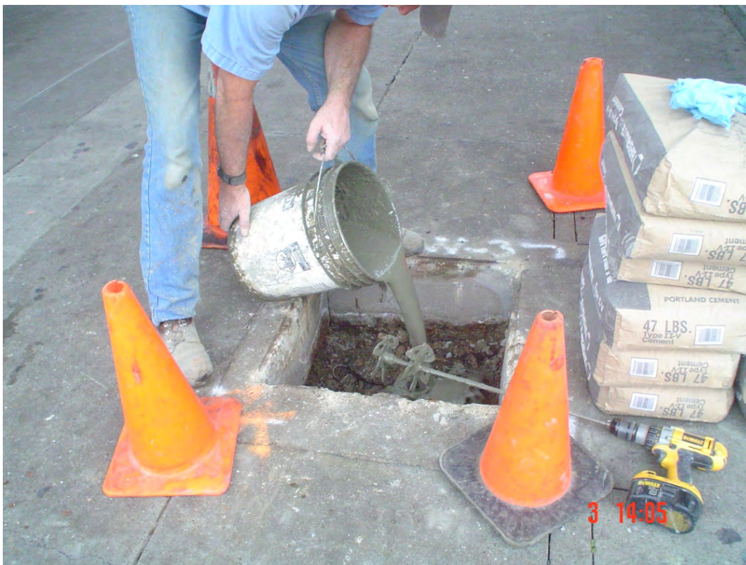
Plate 16. View of Fisch grouting MW-3 at top of casing
