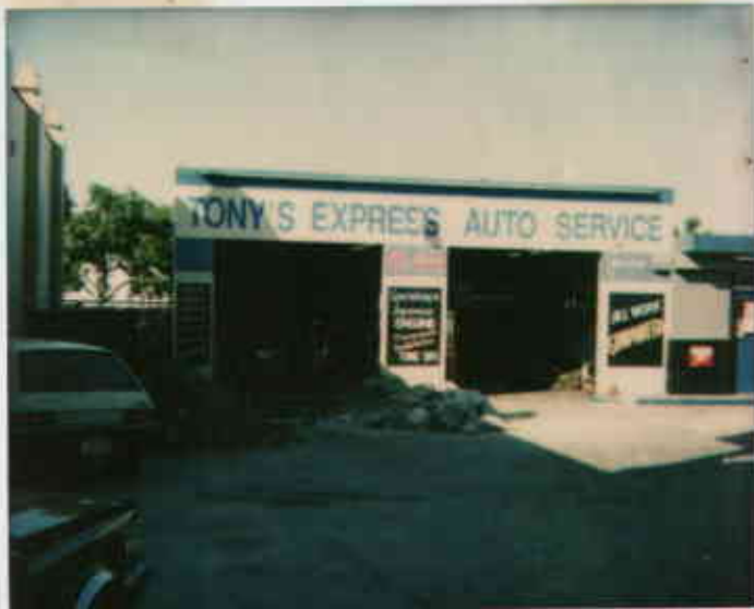
7/11/93 - waste oil tank pit in front of service bay
