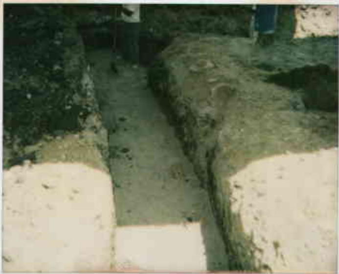
Overexcavating preparing area 3609 E 14th 7/13/93
