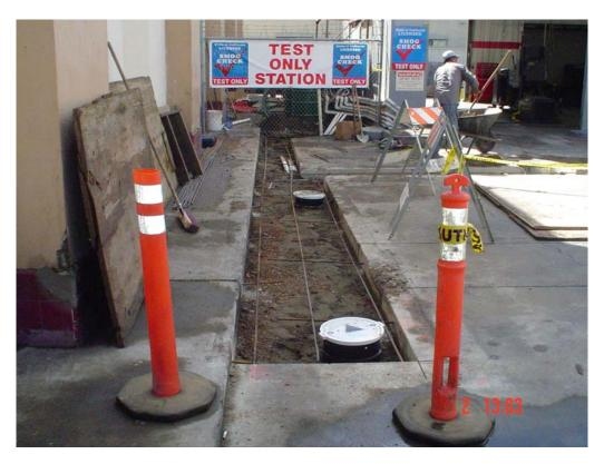
Rebar Placed in Trench for Concrete Pour
