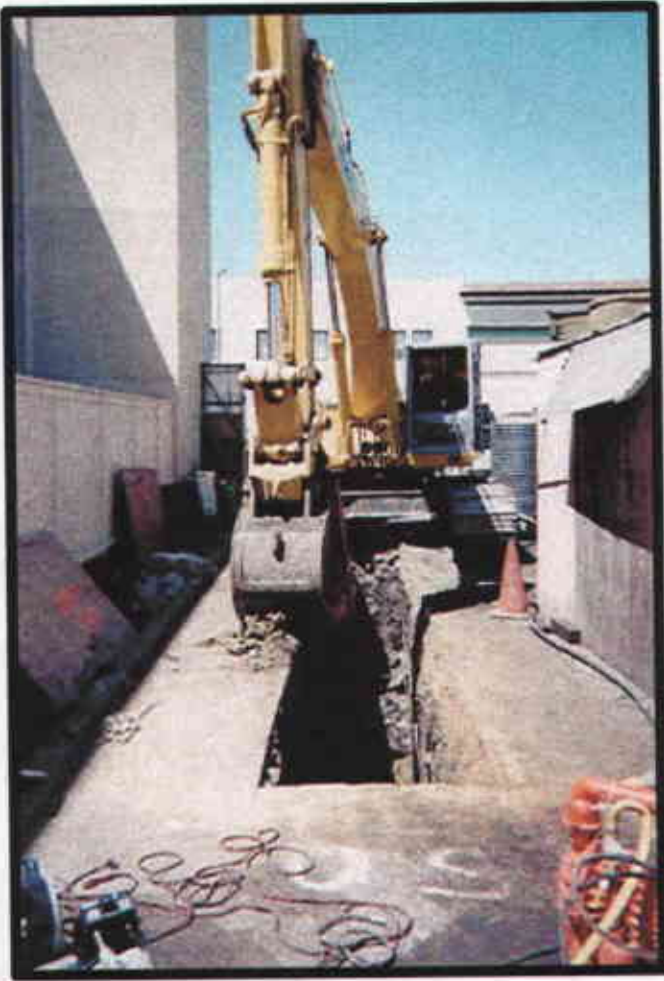
A-1: Beginning French Drain Excavation
