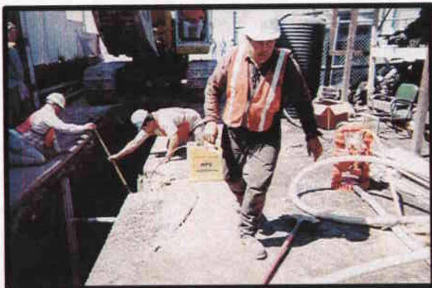
A-10: Setting the Trench Shoring
