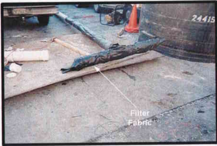
A-4: Filter Fabric Wrapped Over Riser
