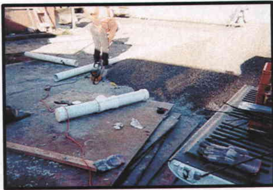
A-3: Constructing a Riser
