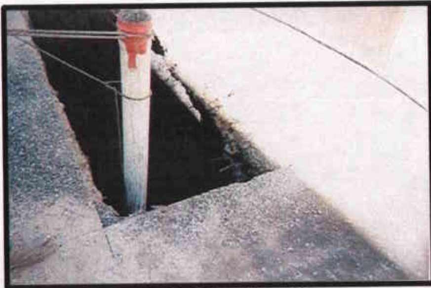
A-6: East Riser Being Set
