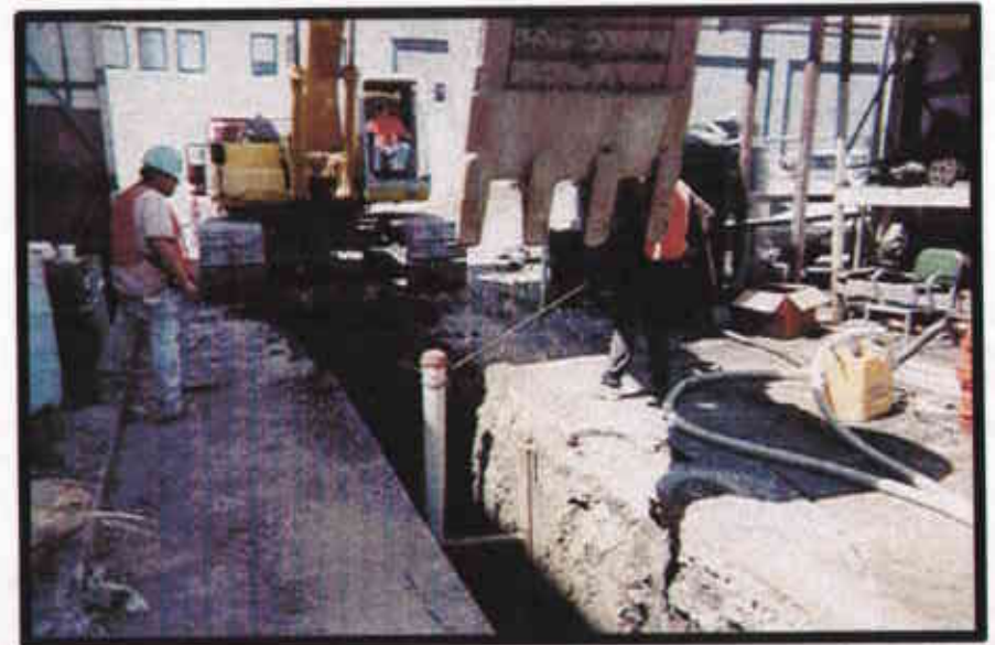
A-11: Backfilling French Drain at the Center Riser
