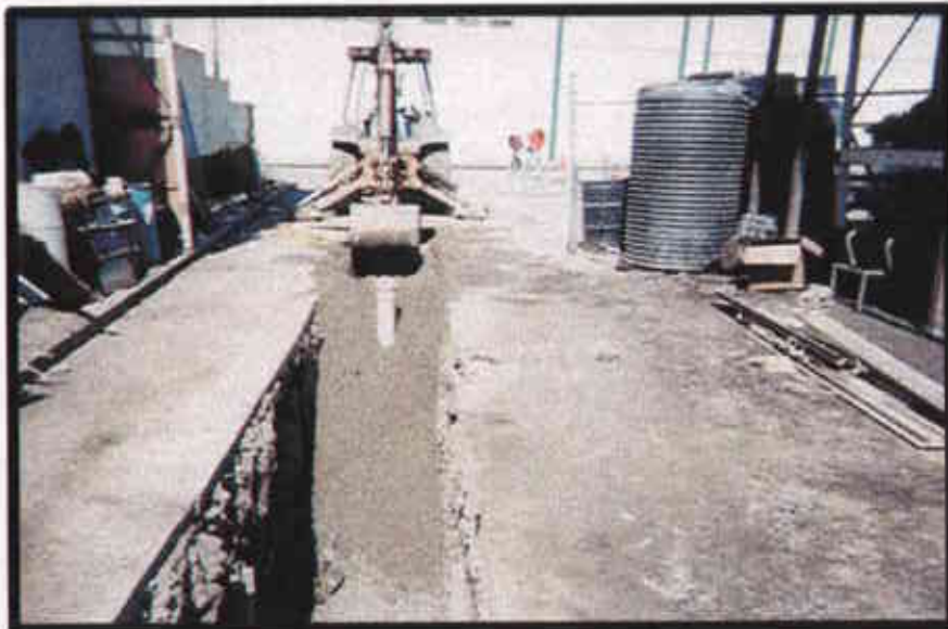
A-14: Pea Gravel Backfill from West to East
