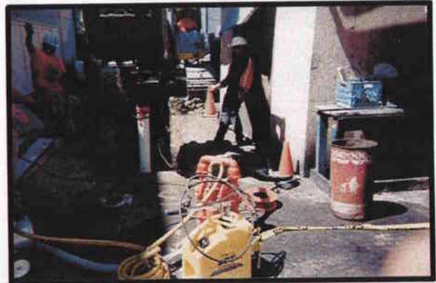
A-7: Backfilling East End with Pea Gravel
