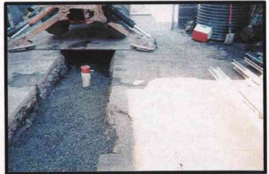
A-15: Leveling the Backfill 2 Feet Below the Surface
