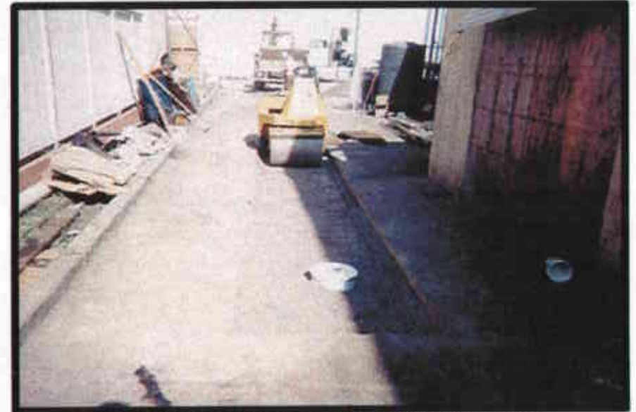
A-17: Compacting Base Rock Prior to Paving
