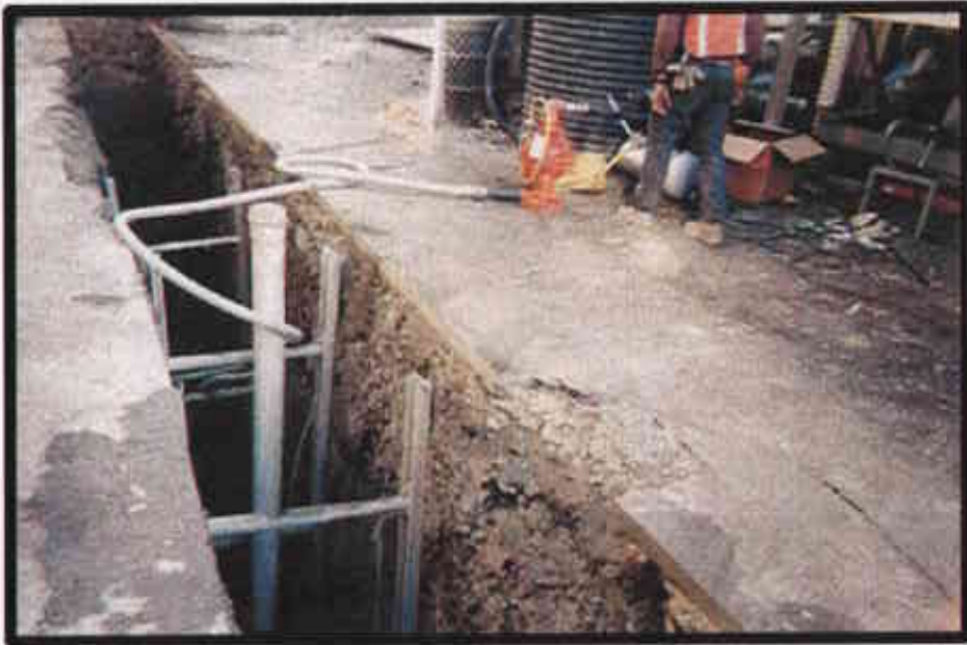
A-12: Pumping Water from the Excavation
