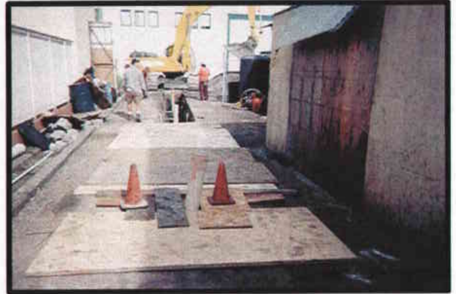
A-13: Beginning Backfill at the West End
