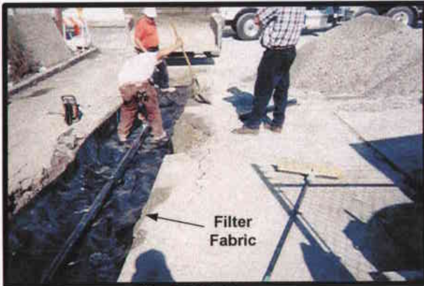
A-16: Filter Fabric On Top of Backfill
