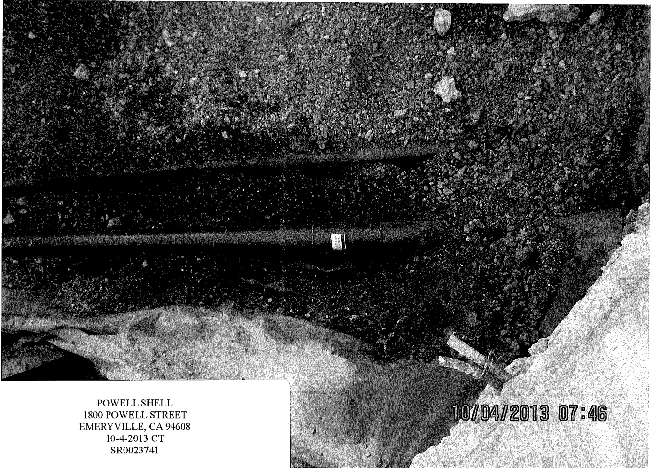
EXCAVATION AND PIPING REPAIR ON DIESEL PRODUCT LINE
