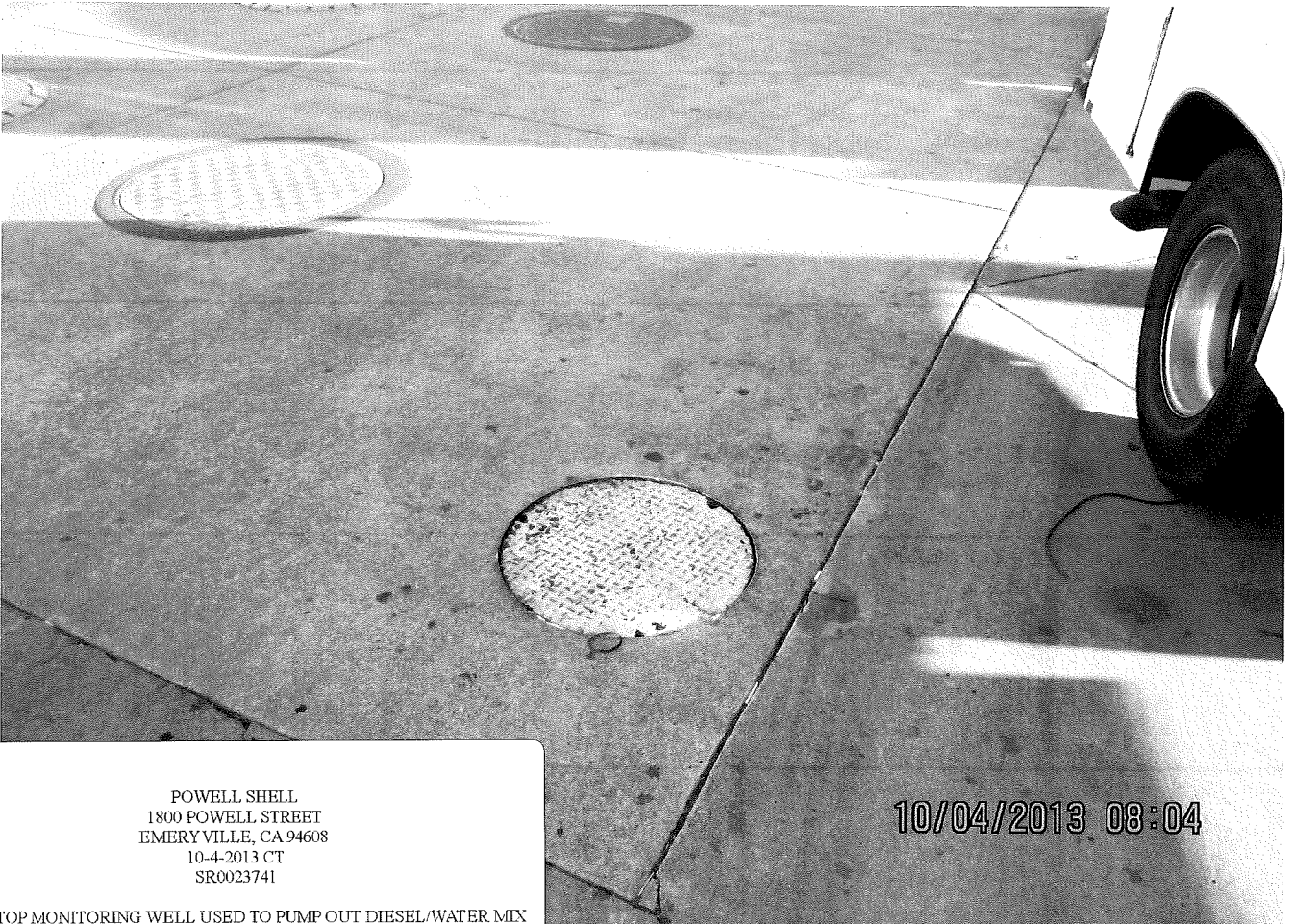
TANK TOP MONITORING WELL USED TO PUMP OUT DIESEL/WATER MIX
