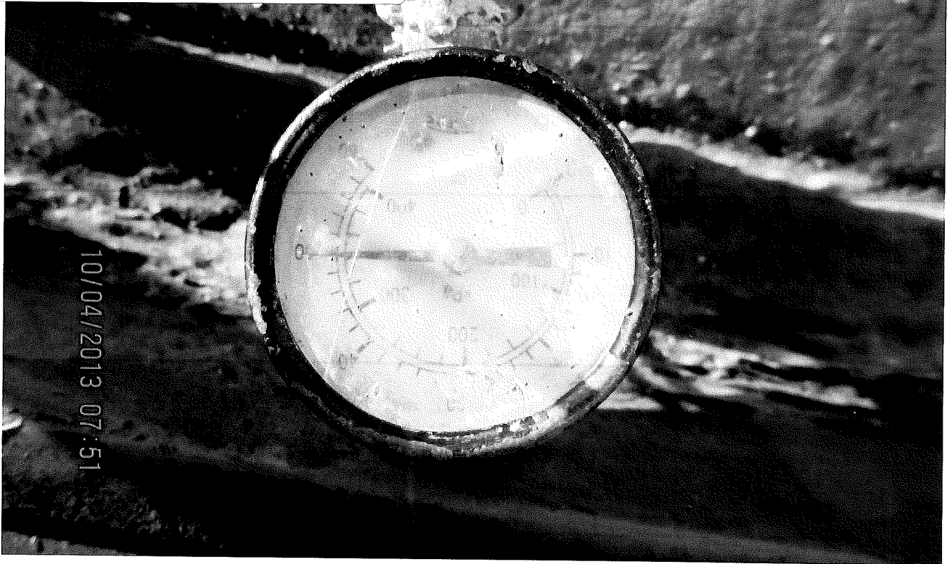
REPAIRED DIESEL PRODUCT PIPING UNDER 50 PSI TEST
