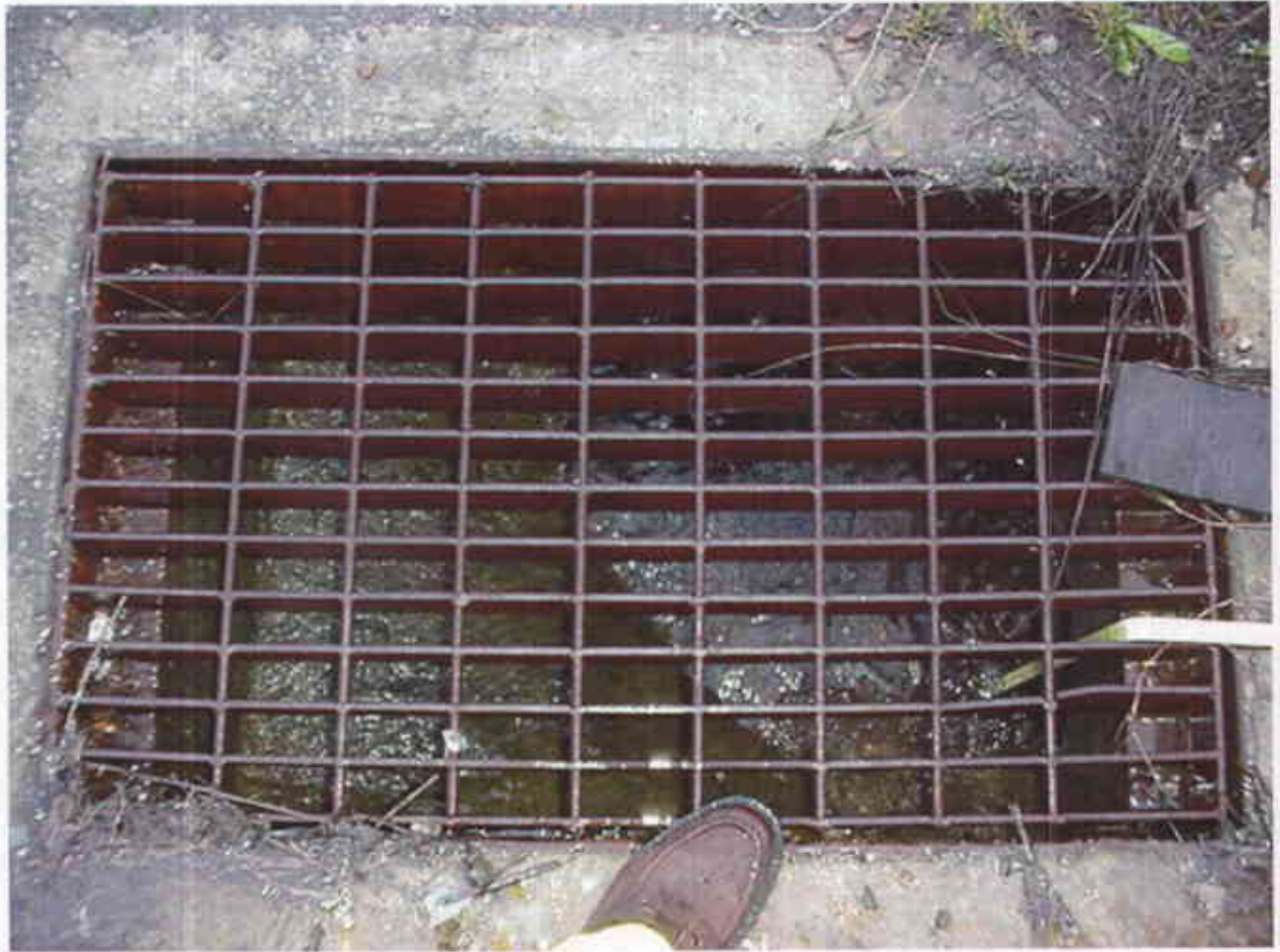
VIEW FROM ABOVE STORM DRAIN
