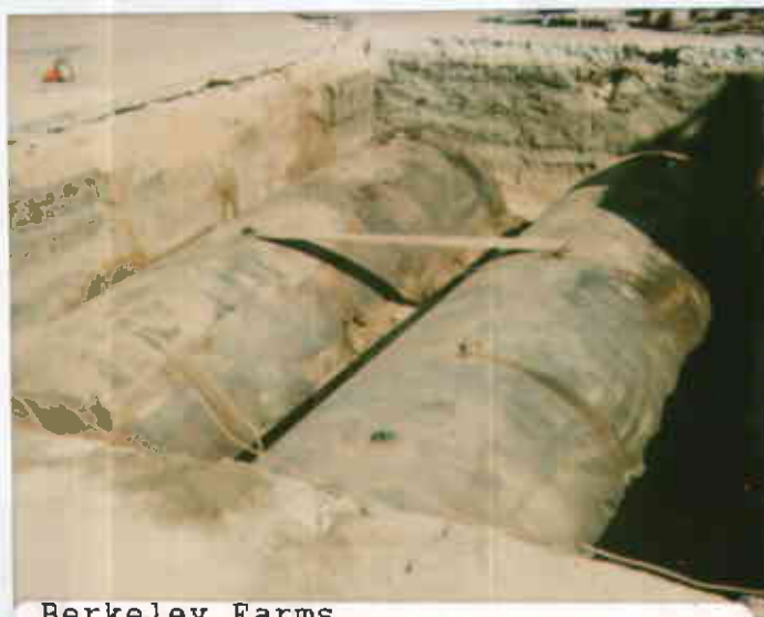
Berkeley Farms 4550 San Pablo Avenue Emeryville 9/11/98 RWeston Removal of 2 USTs
