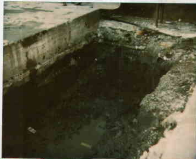
2 2/4/99 STID IRK4 EXCAVATION 10617123909-2W 1359 6909 HEATING FUEL COPIES & ENLARGEMENTS CALL 800-421-1030 TANK REMOVAL
