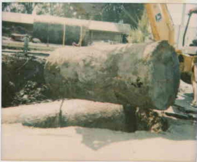
OK tank #1, tubes on entire bottom liquid draining from tank. 9/22/94 BC
