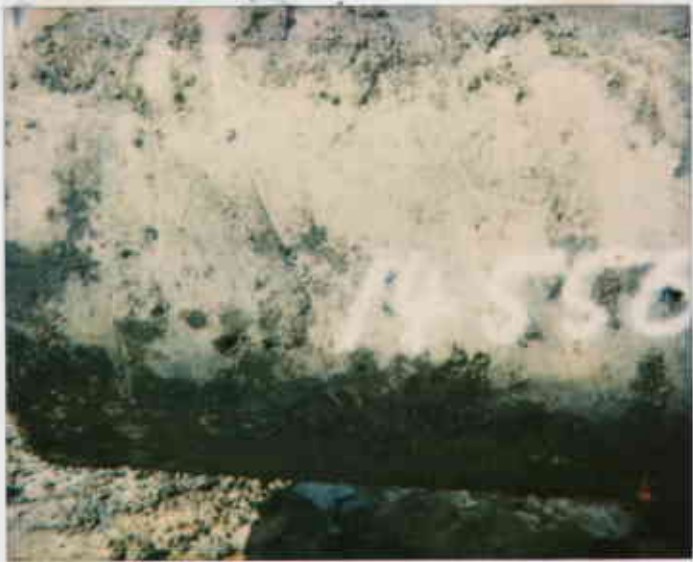
South end Tank #4 CalTrane reddled w/holes 9/22/94 R
