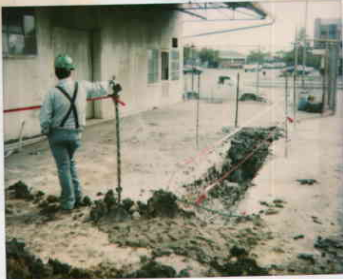
Repairing trench at Cal Trans STJ Heg, Rd 9/22/94 BC
