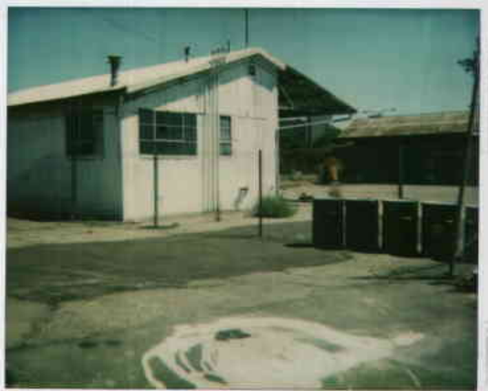
Next to Cal Trans bldg 8/5/93 see vicinity
