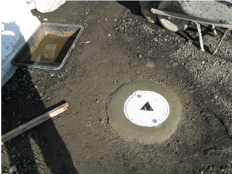
View of the completed well box of MW-5.
