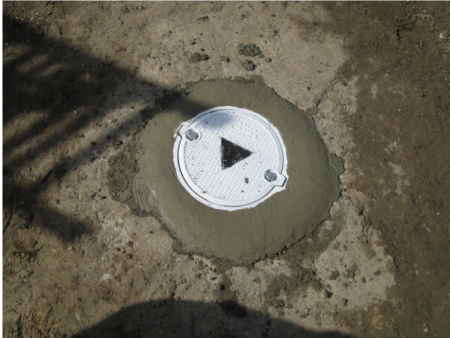
View of the completed well box of MW-2.
