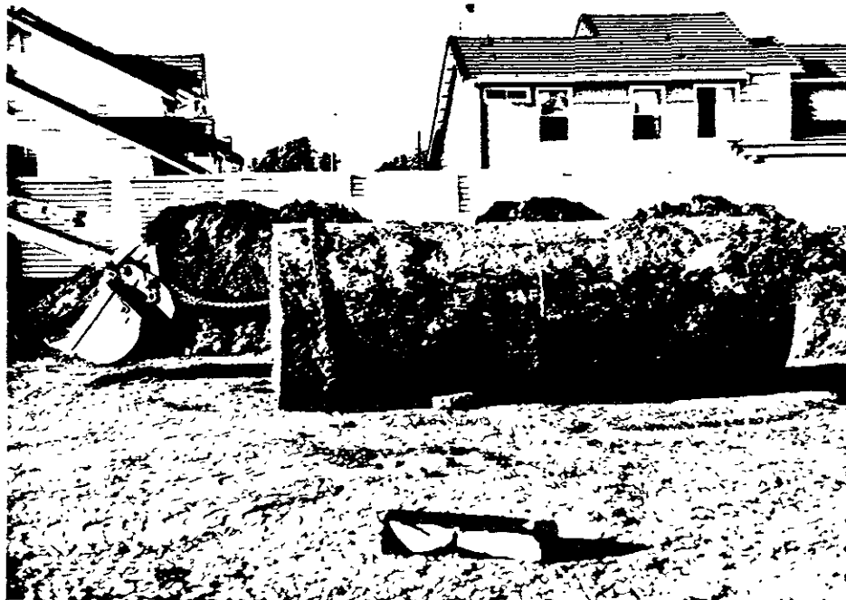
FUEL OIL TANK AFTER REMOVAL FROM EXCAVATION
