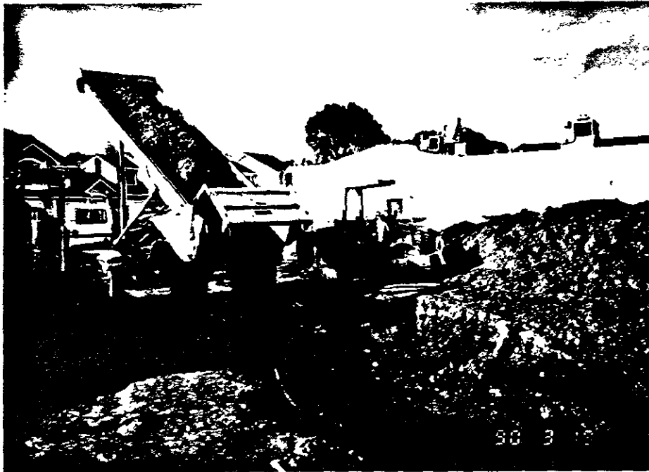
BACKFILL MATERIAL BEING UNLOADED AT SITE
