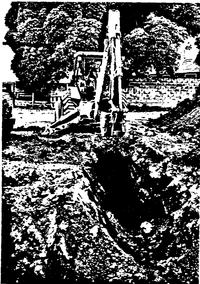
STOCKPILE AREA FOR SOIL/OILY WATER MIXTURE FROM FUEL OIL TANK EXCAVATION NOVEMBER 8, 1989
