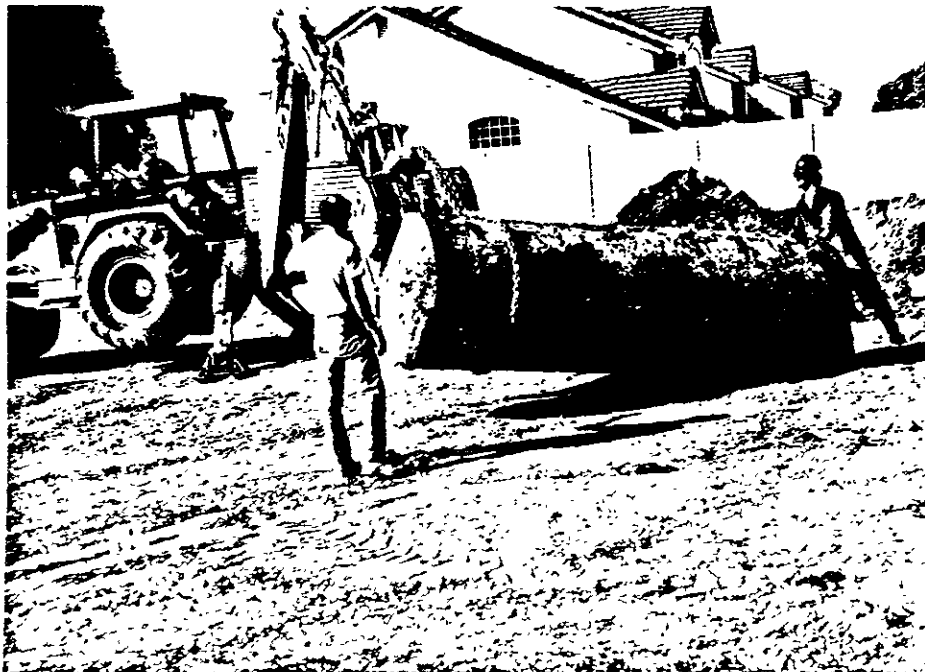
GASOLINE TANK AFTER REMOVAL FROM EXCAVATION NOVEMBER 8, 1989
