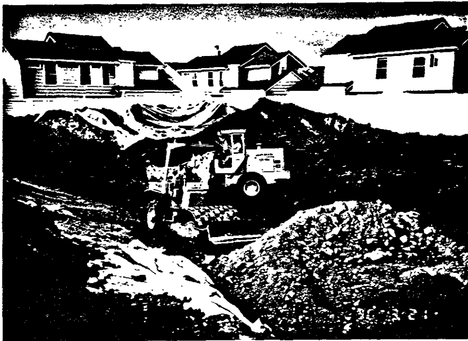
TOP LAYERS OF "CLEAN" MATERIAL FROM FUEL OIL EXCAVATION BEING SPREAD AND COMPACTED IN GASOLINE TANK EXCAVATION
