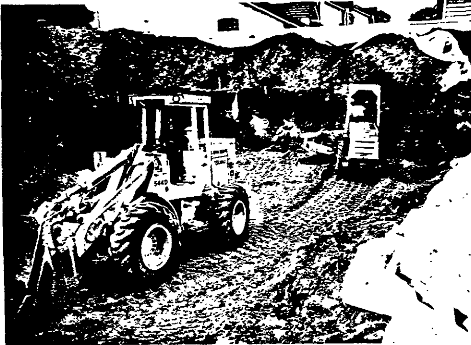
FRONT-END LOADER AND TAMPING FOOT COMPACTOR
