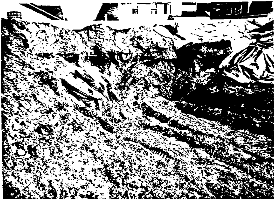
INITIAL BACKFILL LAYERS AFTER BEING SPREAD IN EXCAVATION
