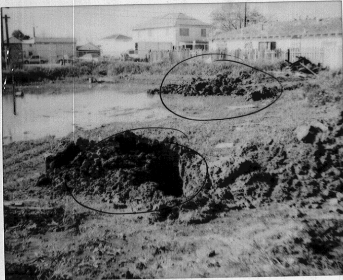
4/2/91 342 105th Ave 2 pits dug ~20' on east + south side
