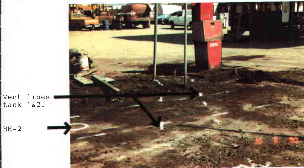
Figure 3B. View North, N. side of tank 1, S. side of tank 2. BH-2 at extreme left, vent lines are dashed.
