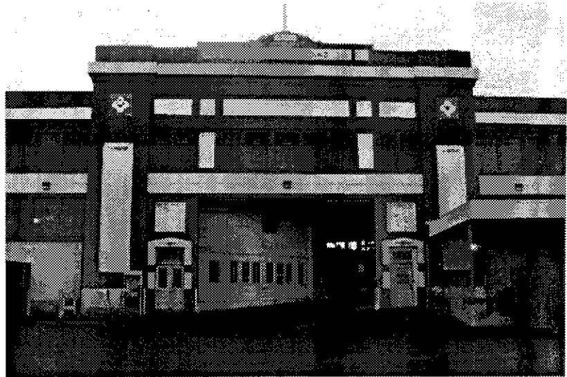
5. Detail of front of transit shed, looking south.
