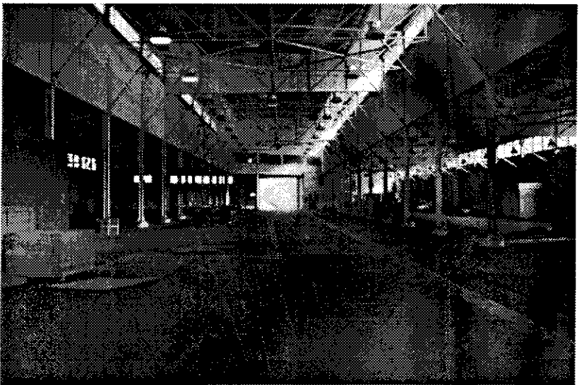
6. Interior of transit shed, looking north from back to front.
