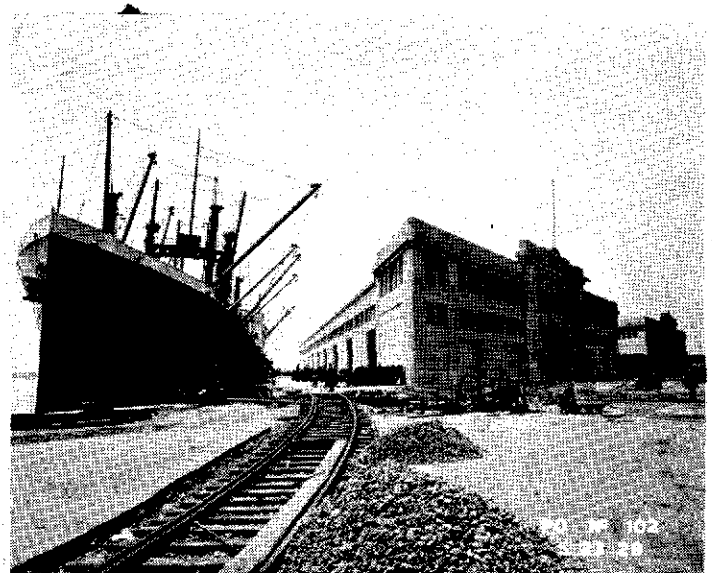
4. Grove Street Pier (Howard Terminal), ship moored, railroad tracks under construction. View looking southwest, 23 May 1928.
