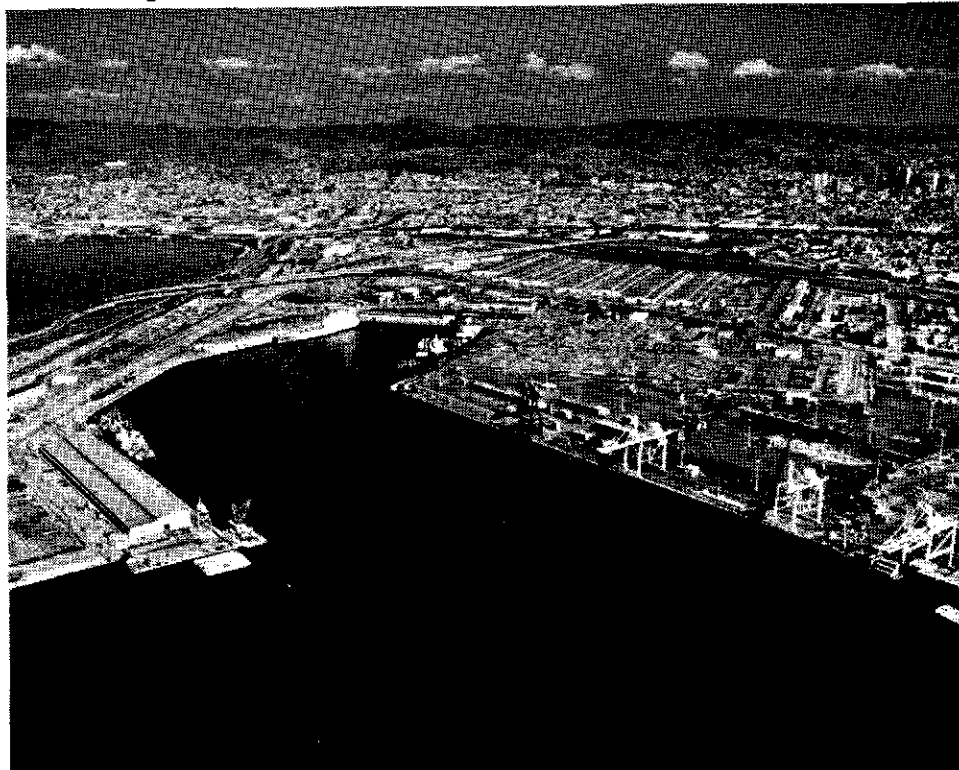
2. 1981: Fourteenth Street Unit has been totally demolished for expansion of Sea-Land Terminal; additional container facilities extend to south.
