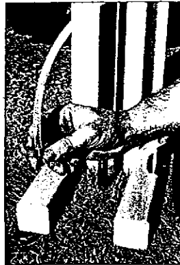
Figure 8. Tubing Bottom Check Valve and Check Ball are installed onto Tubing . . .
