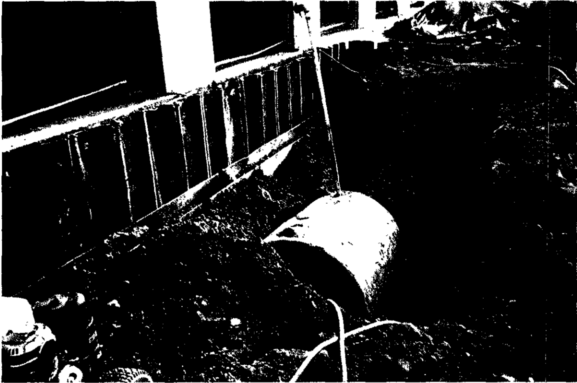
Uncovered USTs CF-19 in Foreground and CF-20 in Background
