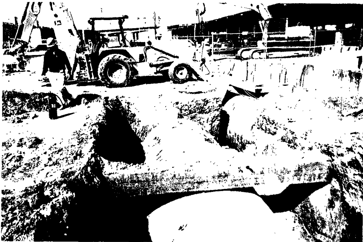
Uncovered USTs CF-18 in Foreground and CF-17 in Background
