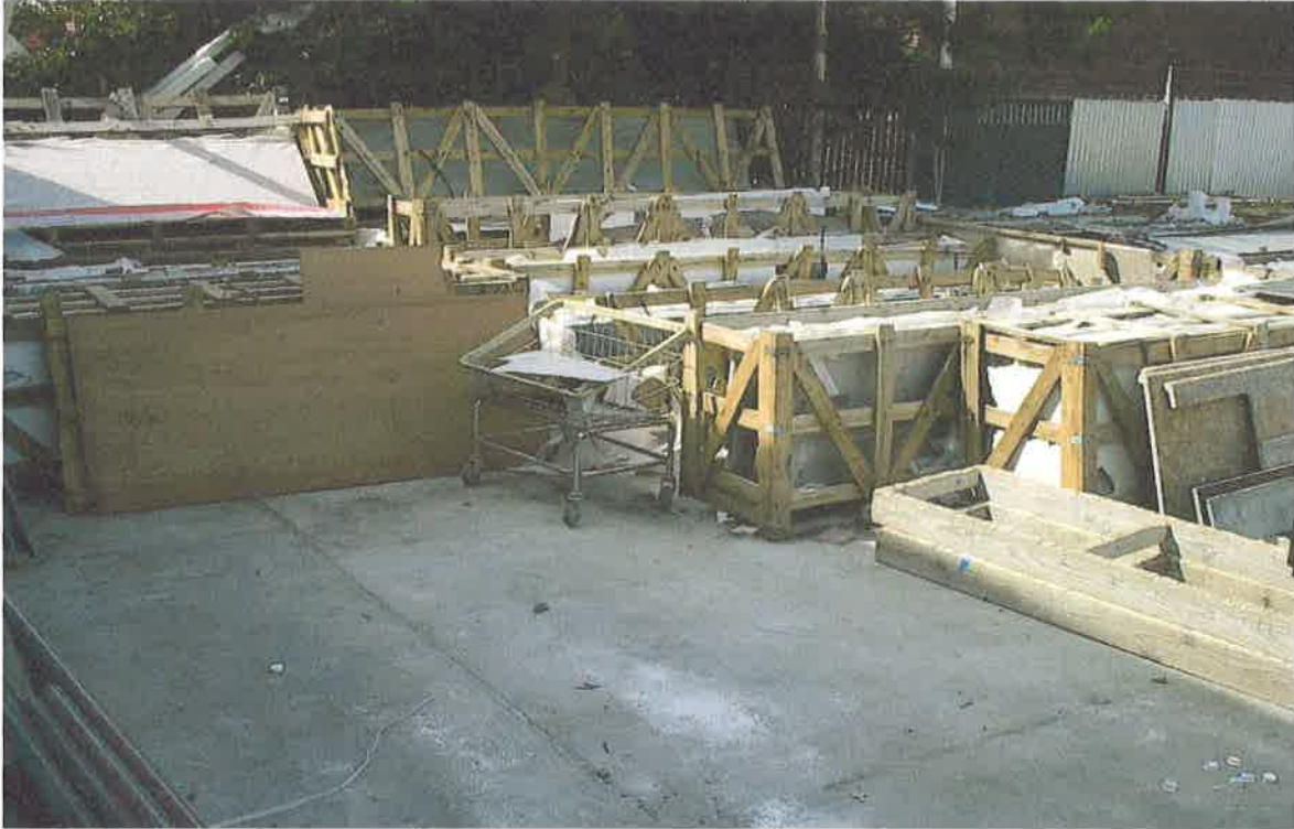
3. Former hoist area.
