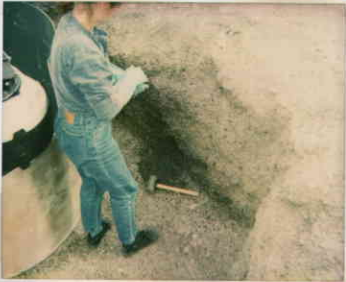
7/6/93 - Photo taken by 2215117976-B Ron Owsatz at Bansal shell, 2120 Montana Ave, Oak. Shown is Allison Watts taking soil sample in side wall of pit where cont. was found at old piping node. (R)
