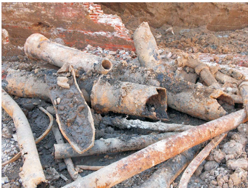
Storm drain and sewer piping removed during redevelopment of the Site.
