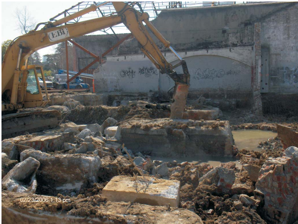
Buried concrete structures to be removed.
