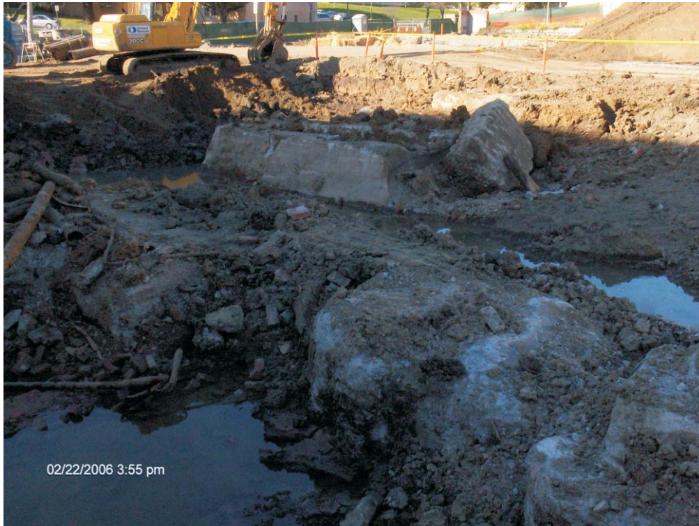
Buried concrete structures.
