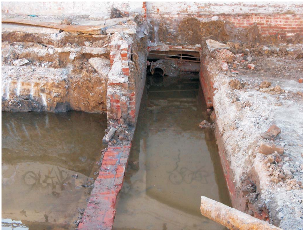
Concrete and brick structures removed from the Site during redevelopment.
