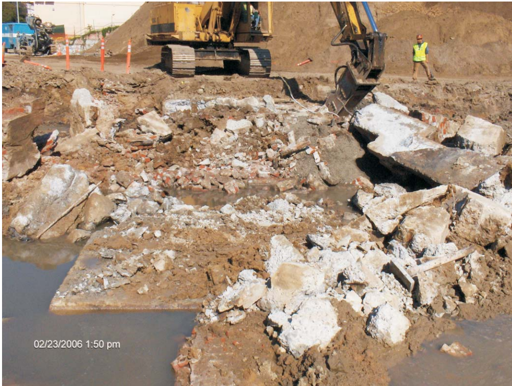
Buried concrete and brick being removed.
