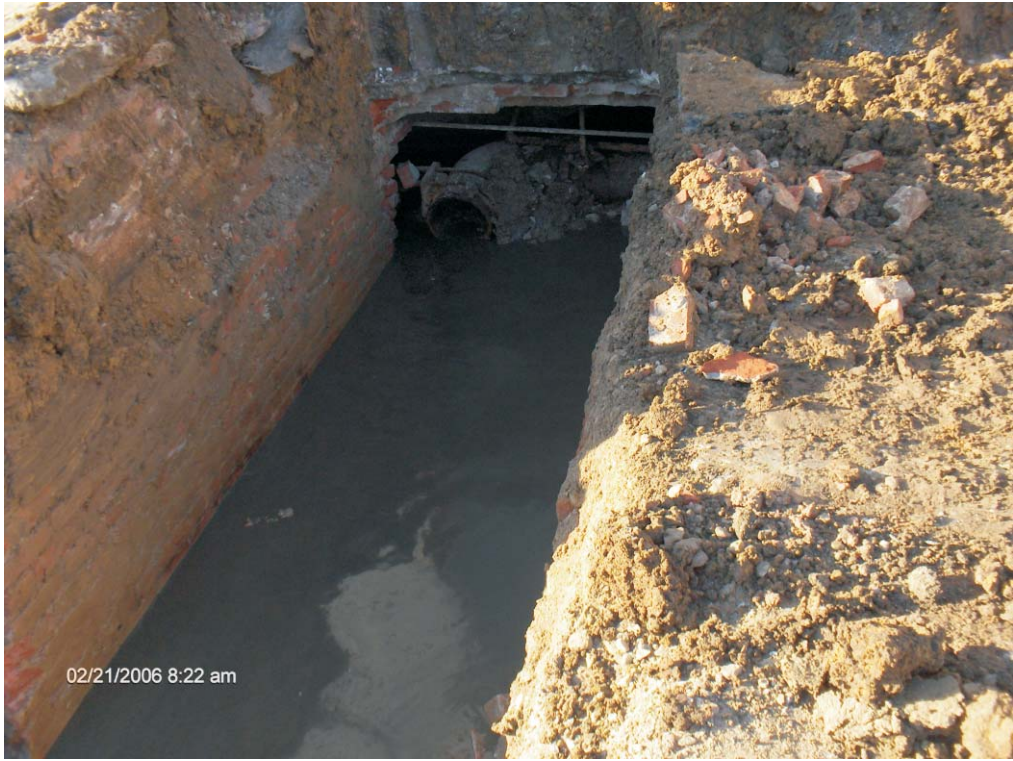
Typical trench filled with water.
