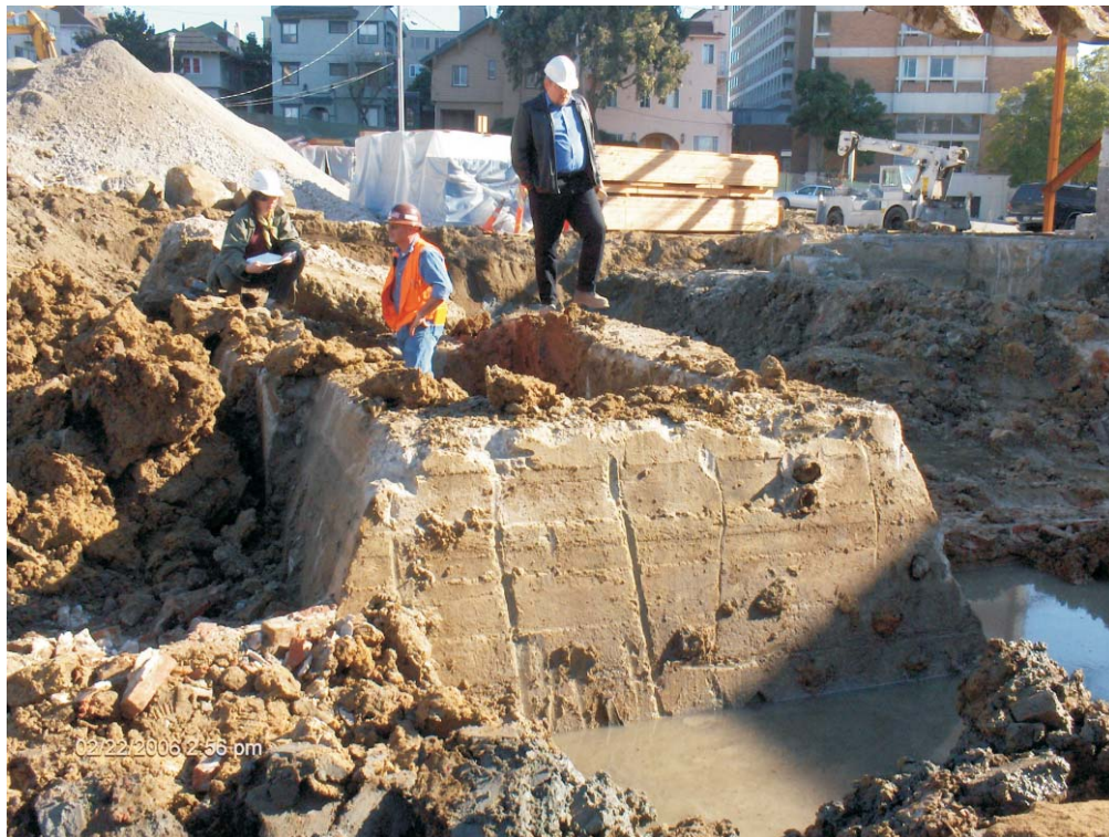
Typical buried concrete structure.
