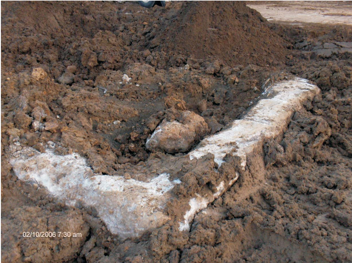
Typical buried concrete structure - in place.
