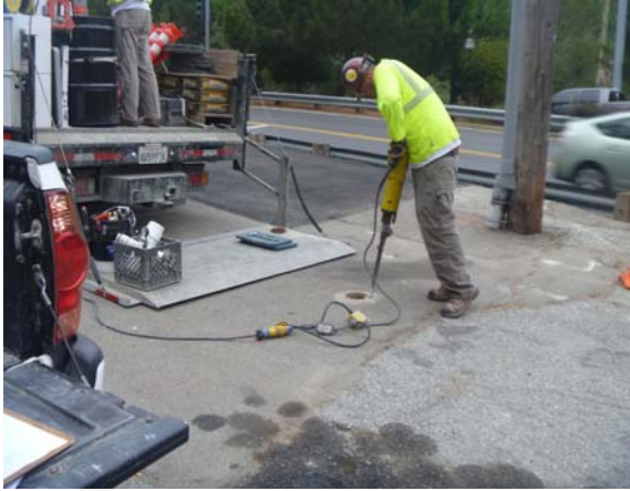
View of the well box being removed.
