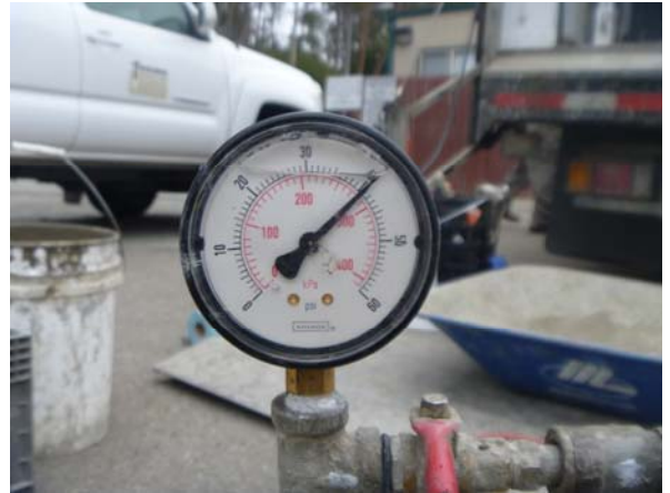
View of pressure gauge at start of pressure grout.
