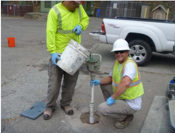
View of tremie grout.
