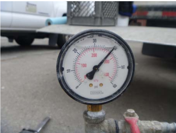
View of pressure gauge at end of pressure grout.
