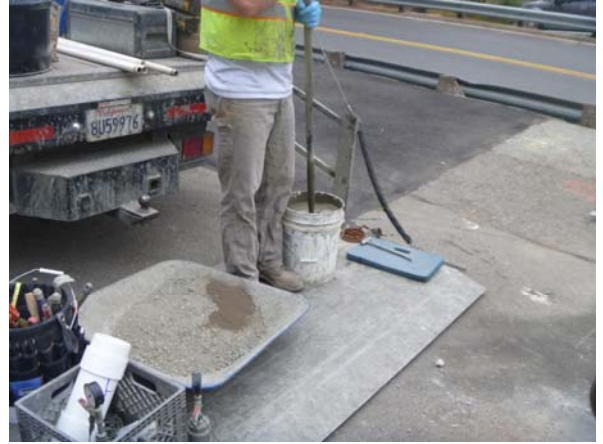
View of grout being mixed.
