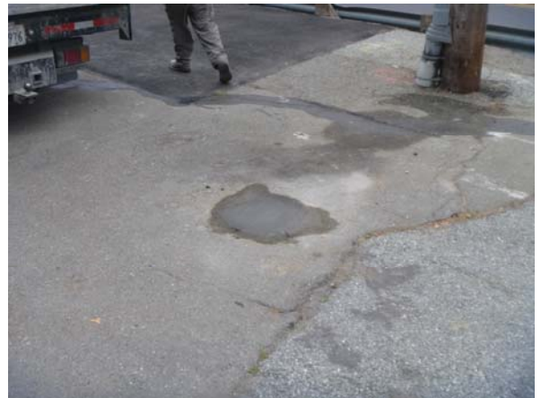
View of finished grade.
