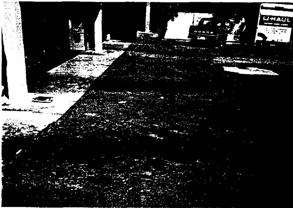
2740 98th Avenue - Staining on Pavement of Property
