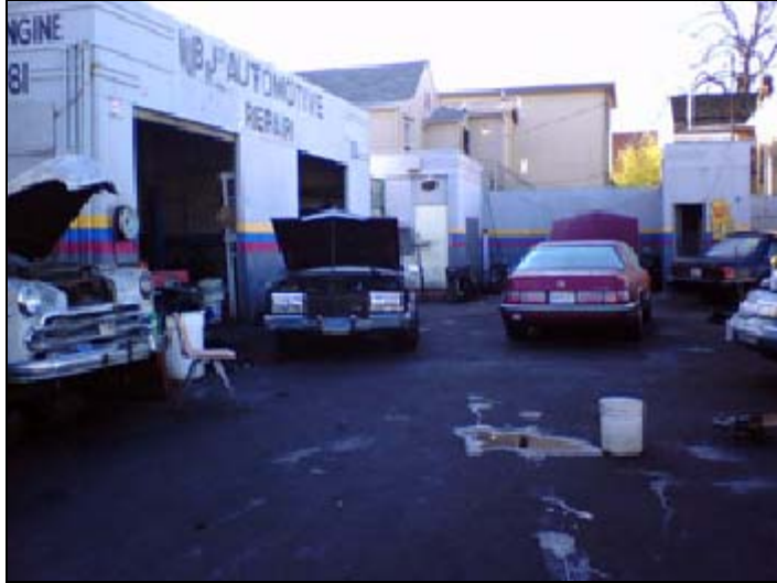
Photograph No. 1 - view southward of subject property and auto repair building from driveway at 16th Street. LBJ's Automotive Repair building to left of photo. Residences adjoin property at south boundary. Small building to right is bathroom with adjacent wash pad area. Small storage building at rear boundary.
