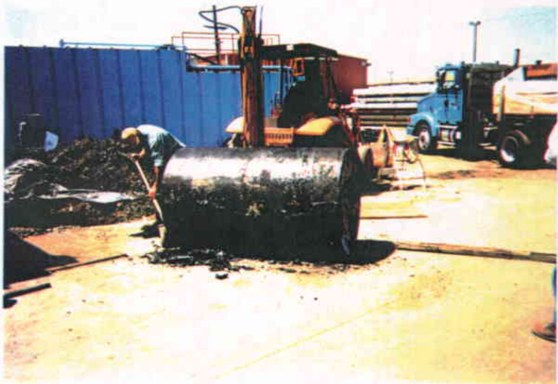
Figure 8: Photographs Showing the Removed Underground Storage Tank
