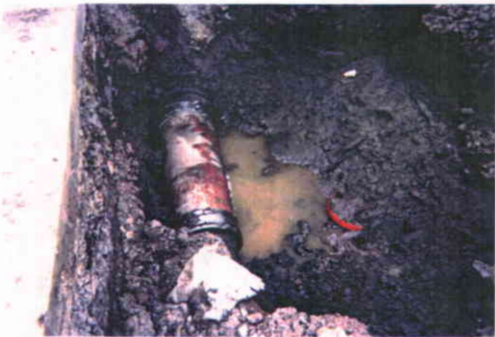
Figure 7: Photograph Showing Repaired Lateral Loop Section
