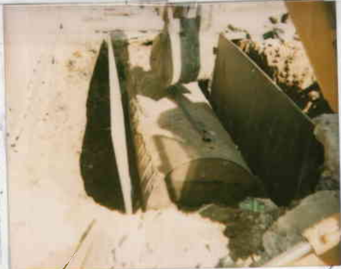
10-12-94 TANK IN PLACE W/ STD 3335 SITING RWESTON
