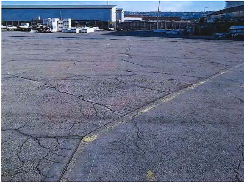
Photographs 13A and 13B: Cracking in Area P of the 2012 report. In 2013, the area has been sealed.
