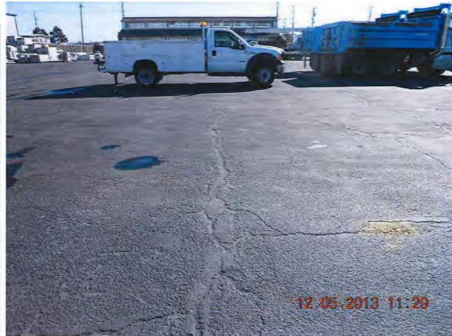
Photographs 9A and 9B: Cracking in Area K of the 2012 report. In 2013, the area has been sealed.
