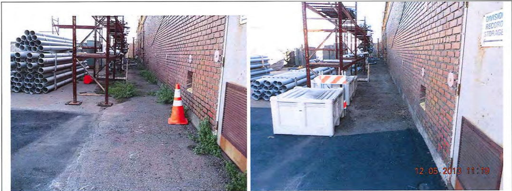
Photographs 2A and 2B: Vegetation along the southeastern side of the cap. In 2013, the foreground has been slurry sealed. Dead vegetation is present along the brick building and under the storage rack.
