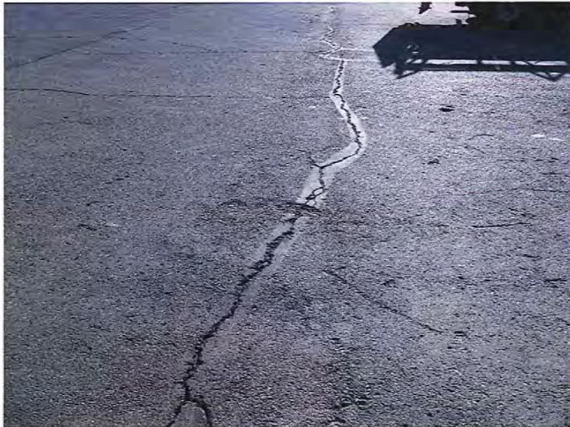
Photographs 9A and 9B: Cracking in Area K of the 2012 report. In 2013, the area has been sealed.
