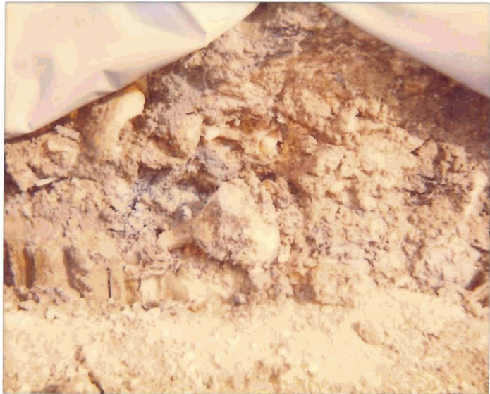
4930 Coliseum Way 11/26/91 RGE, asphalt backfill
