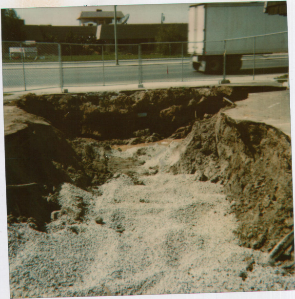
8/23/80 106 + 110 Hwy Filled in pit
