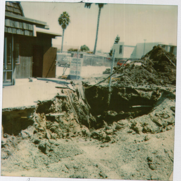
8/27/90 106 Meyenberg Overexcavating near building
