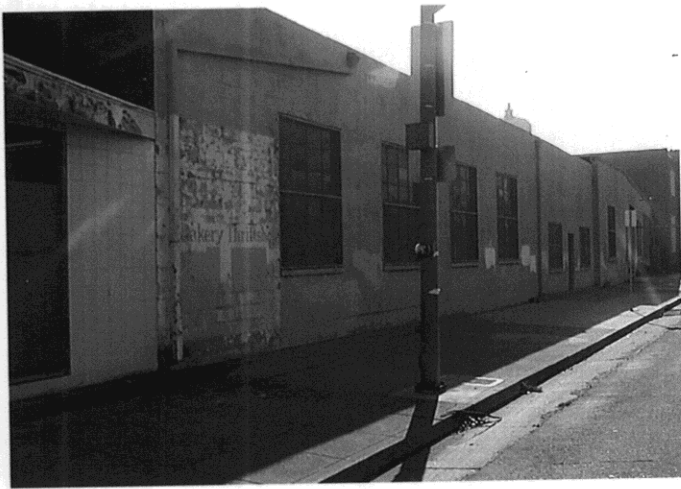
Along Adeline to 53 rd Rd. View of IBC warehouse 945-53 rd St
