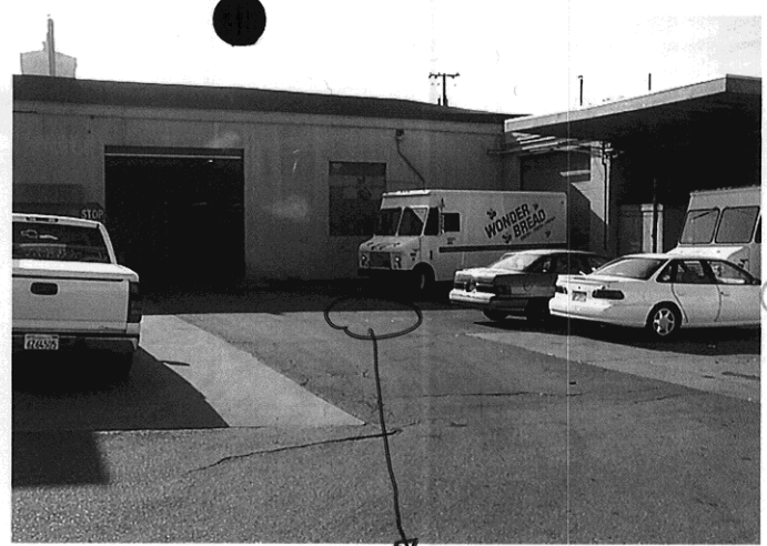
Facing South - MW-3 945-53rd St
