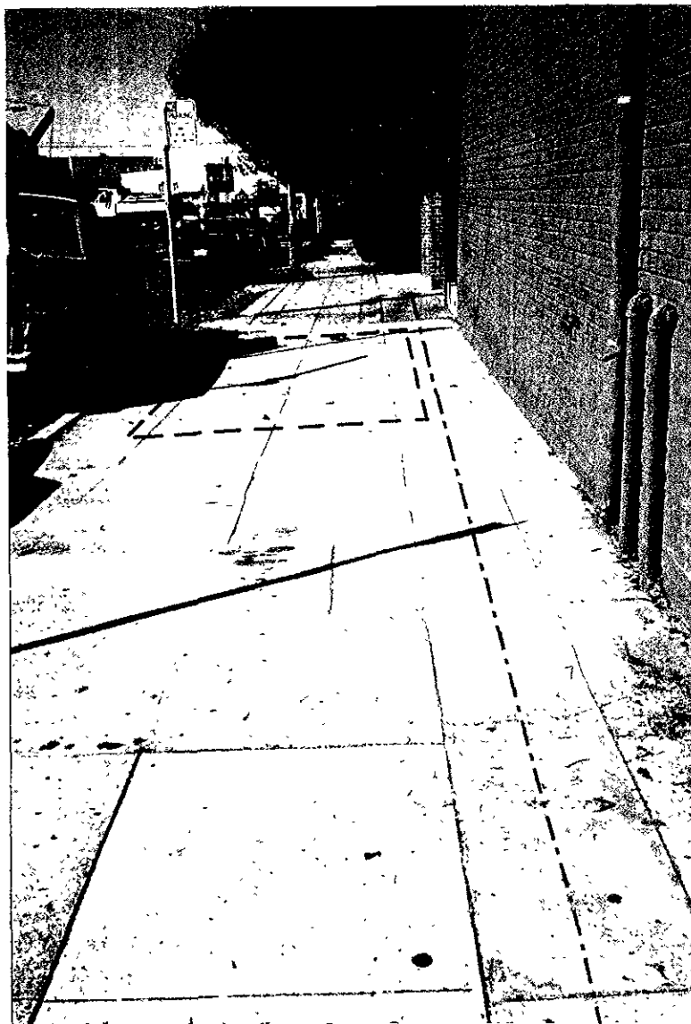
Photo 1 - View of tank area looking east toward Adeline Street. The edges of the tank are marked with the dashed line on the sidewalk and the 2" diameter gas line is marked by the dashed line between building and tank.
