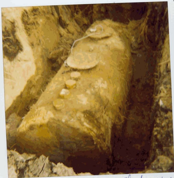
WST IN PLACE 1333 PARK AVE. Emerysville
