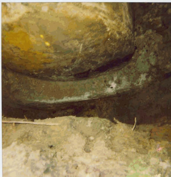
Slab under WST @ 1333 Park Ave Emerysville
