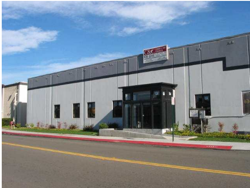
Photo 1. View looking northeast of front of subject property building.
