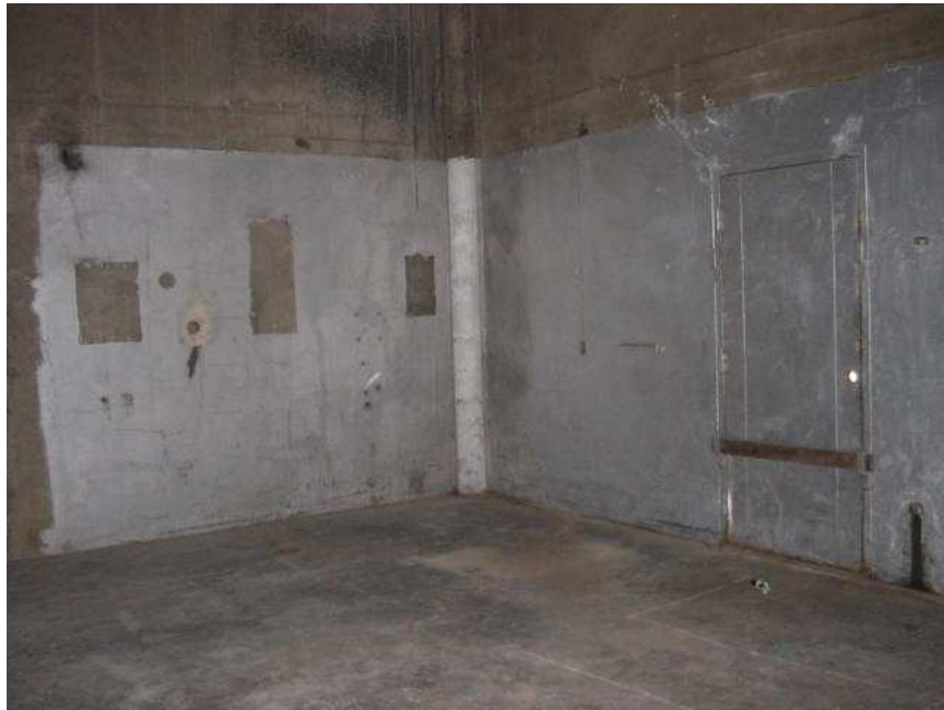
Photo 2. Northeast interior corner of building showing possible paint spray area.
