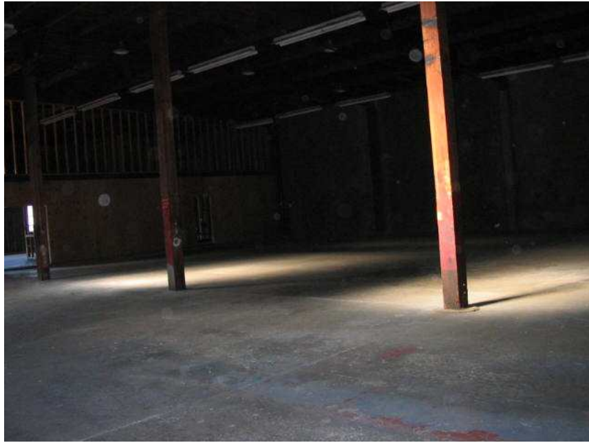
Photo 1. View looking northwest of building interior.
