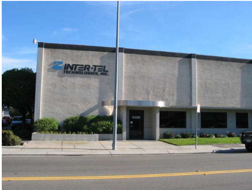
Photo 1. West side of subject property building.
