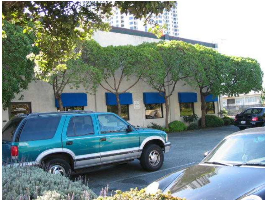
Photo 2. Parking lot at north end of subject property.
